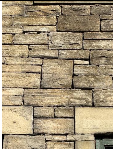
Photo 6: Example of gaps in stone work.
