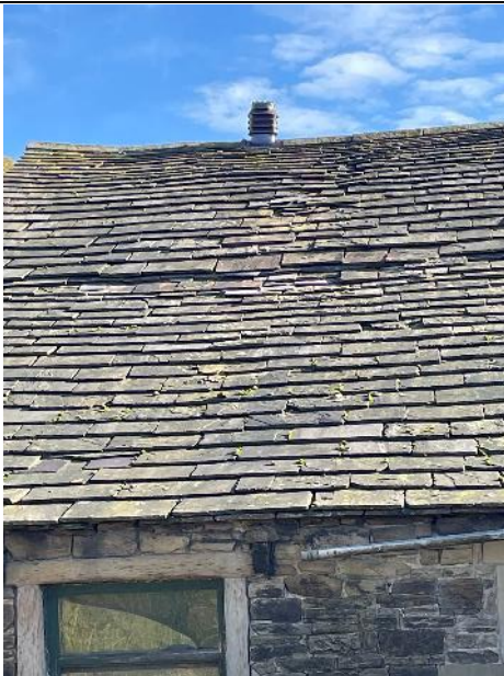
Photo 5: Example of lifted/missing roof tiles.
