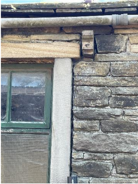
Photo 7: Example of gaps around window lintels/frames and around beam.
