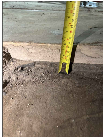
Photo of Existing Floor Construction
