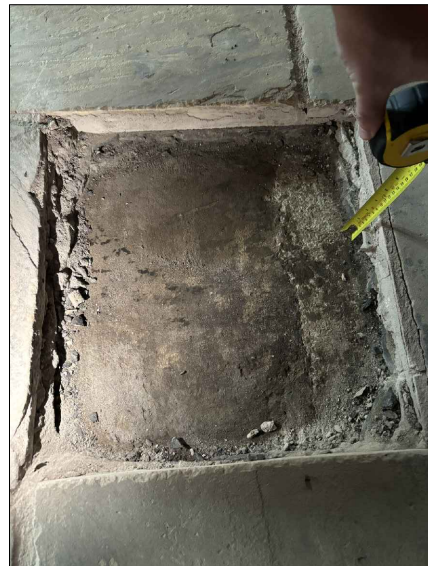
Photo of Existing Floor Construction
