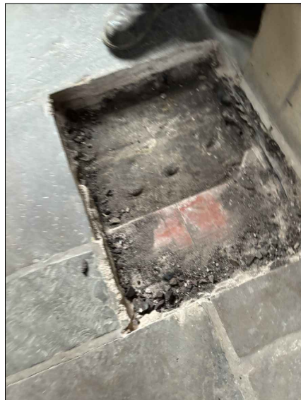
Photo of Existing Floor Construction
