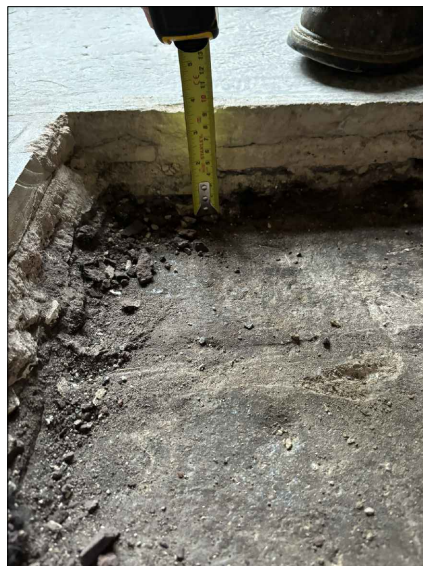
Photo of Existing Floor Construction
