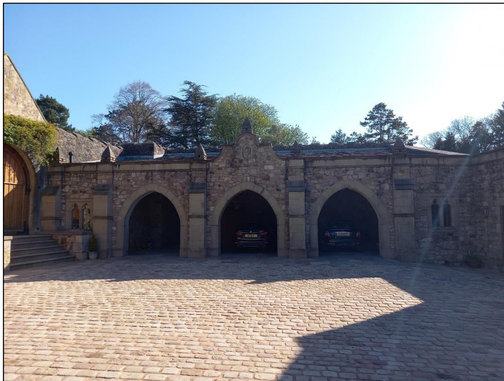
PL02: View of the modern garage extension from the west.
