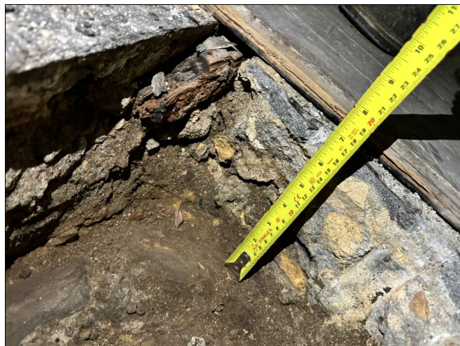
Photo of Existing Floor Construction
