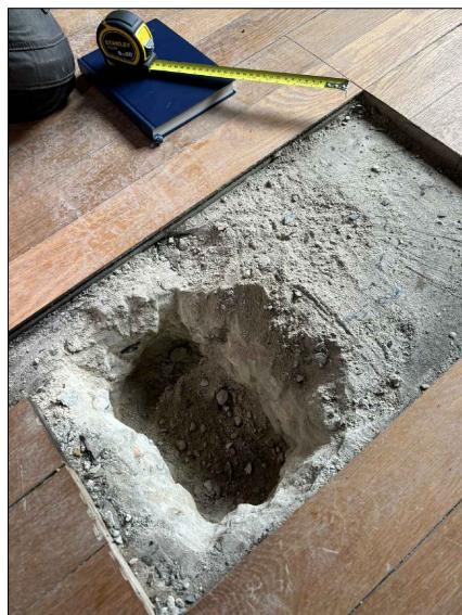
Photo of Existing Floor Construction
