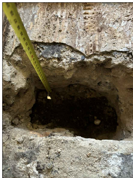
Photo of Existing Floor Construction
