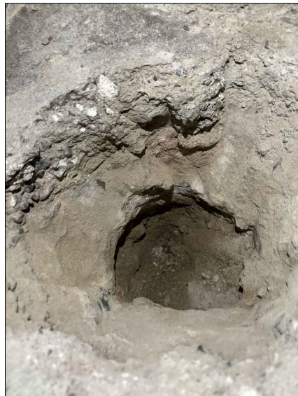
Photo of Existing Floor Construction
