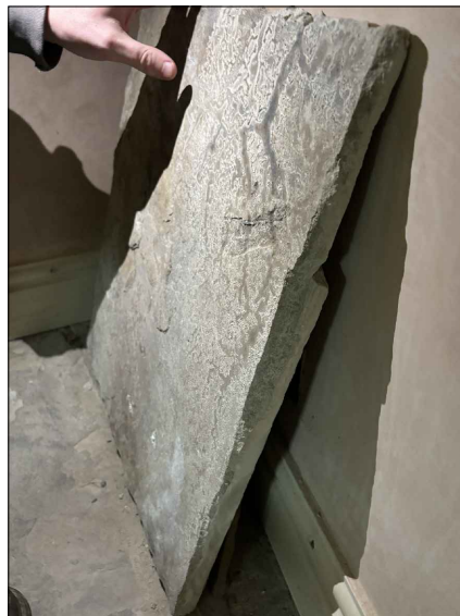
Photo of Existing Floor Construction
