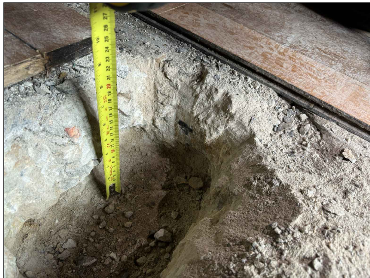
Photo of Existing Floor Construction
