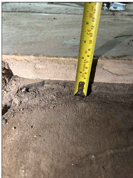
Photo of Existing Floor Construction
