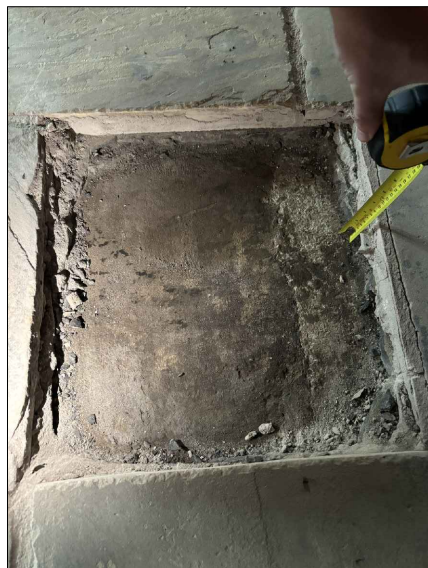
Photo of Existing Floor Construction
