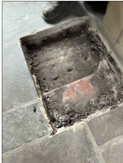
Photo of Existing Floor Construction
