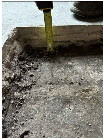
Photo of Existing Floor Construction
