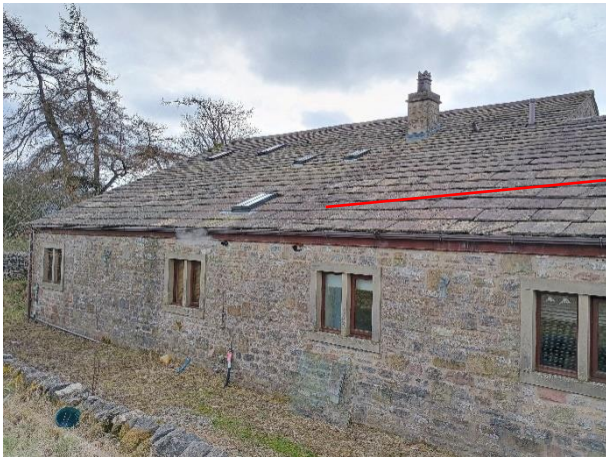
Photograph 3: Northeast elevation of B1
