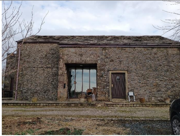
Photograph 1: Southwest elevation of Building 1 (B1)
