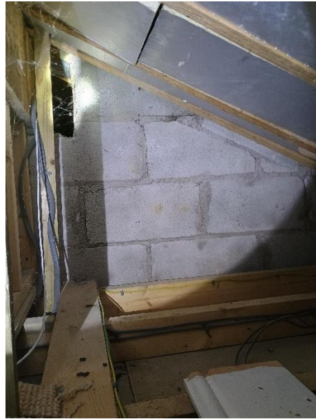
Photograph 8: Wardrobe crawl space on first floor of B1
