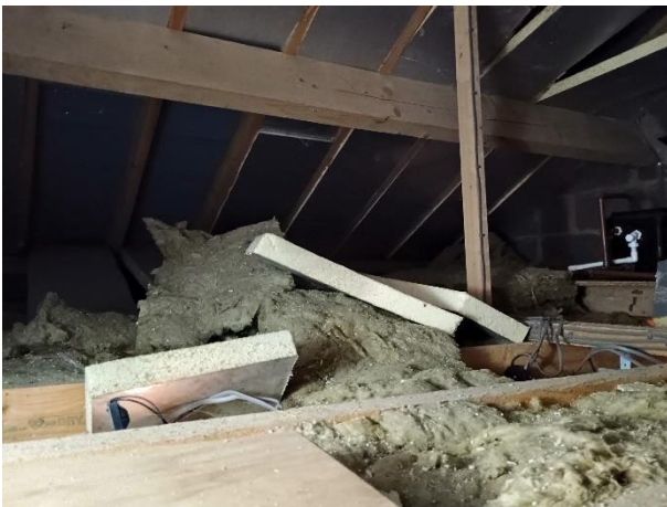
Photograph 9: Loft space on first floor of B1
