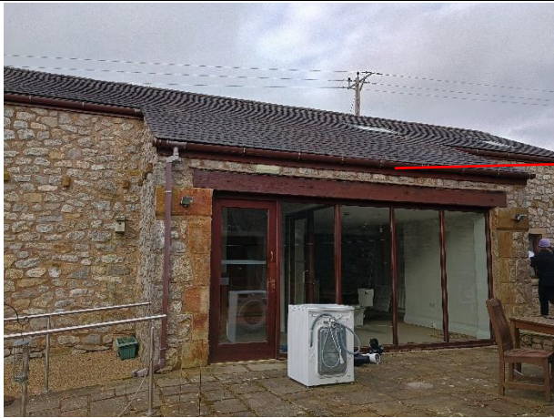
Photograph 11: Southeast elevation of Building 2 (B2)
