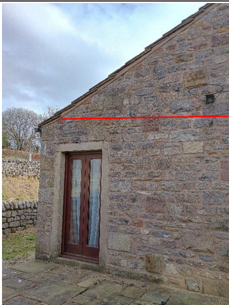
Photograph 5: Part of B1 northwest elevation
