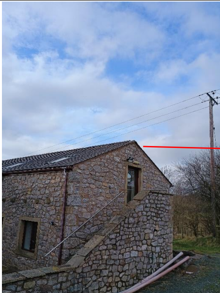
Photograph 15: Northeast/east elevation of B2
