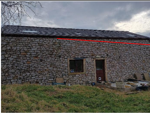
Photograph 13: Northwest elevation of B2
