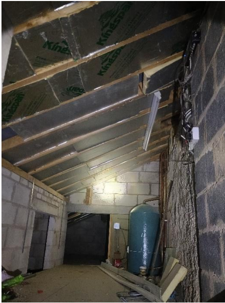
Photograph 7: Loft space on ground floor of B1
