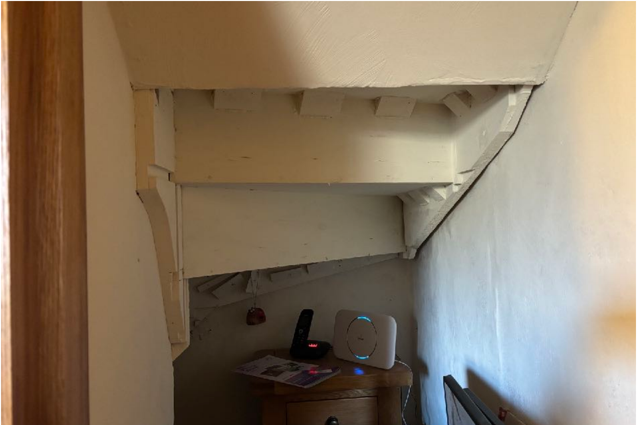
Figure 5: Underside of stairs.
