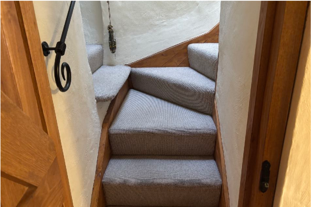
Figure 3: Stairs as seen from the living room. The bathroom stair now discharges on to one large full step.
