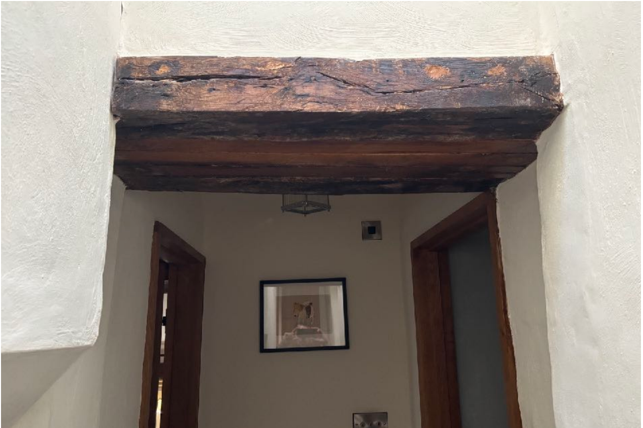
Figure 7: As above, prior timber lintels and reclaimed timbers used.
