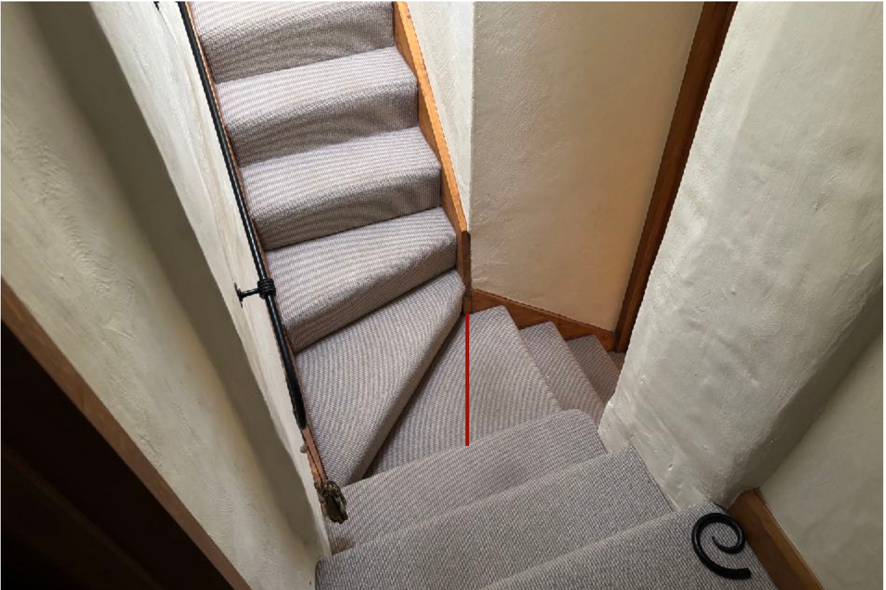
Figure 1: Replacement stair as seen from the bathroom doorway. The red line indicates the former position of a step (see figure 2). This has been removed and the steps reconfigured so as to form a small landing making use of the 'bathroom' steps safer.
