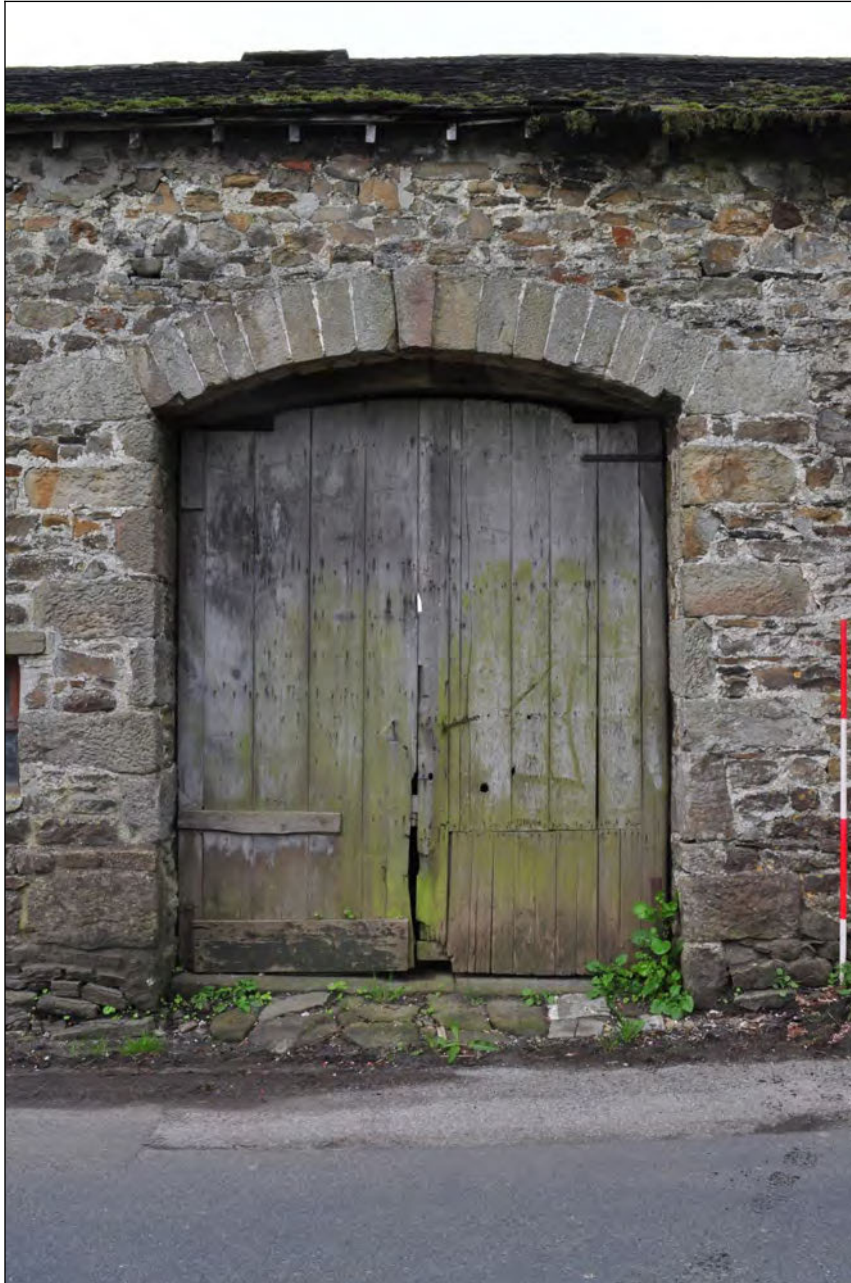
Photo 6: Main building: cart entrance, north elevation
