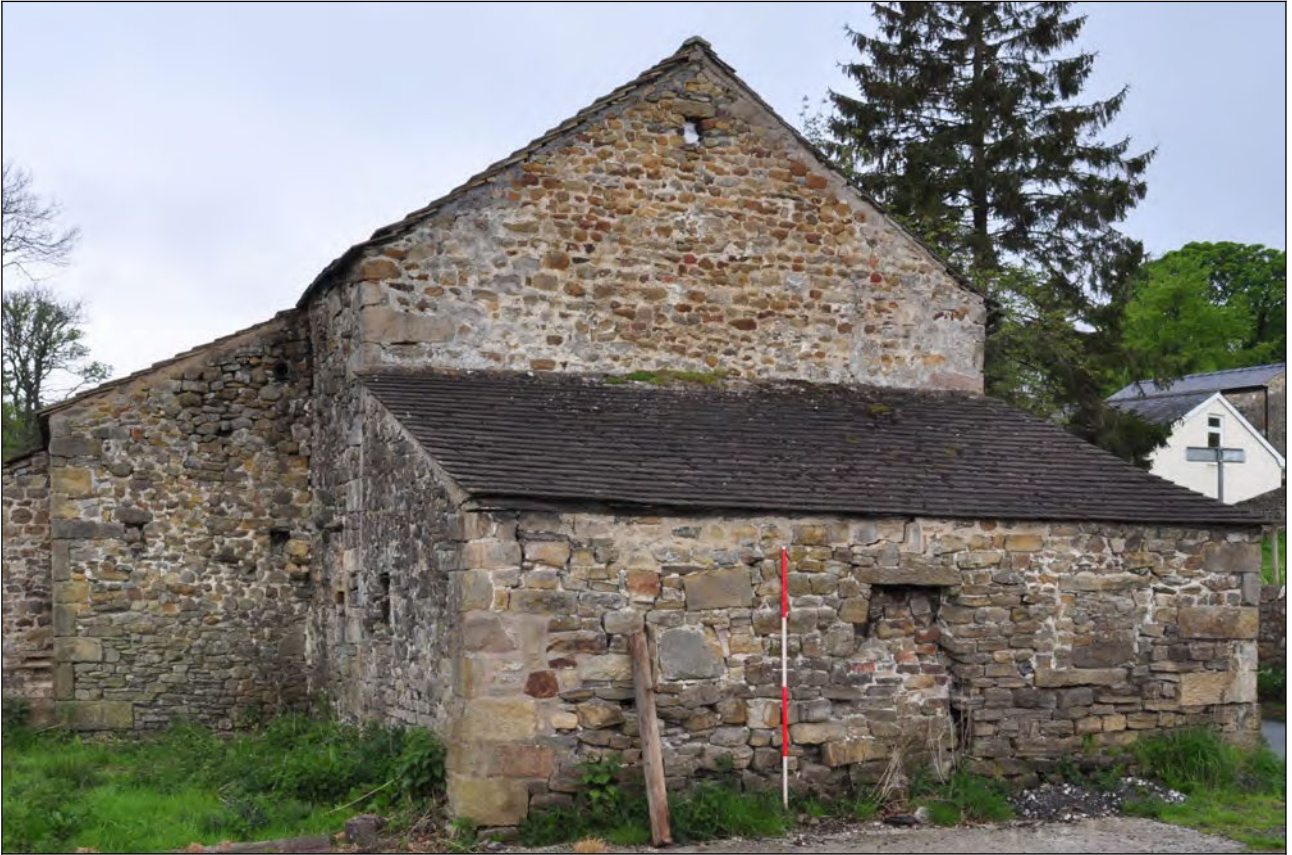
Photo 56: East lean-to, looking north-west
