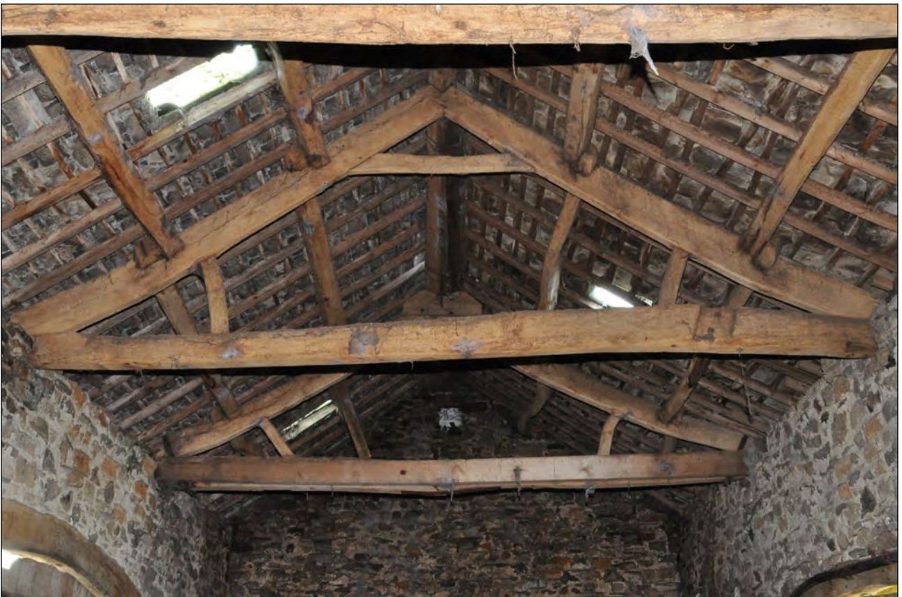
Photo 35: Main building: eastern roof trusses, looking east
