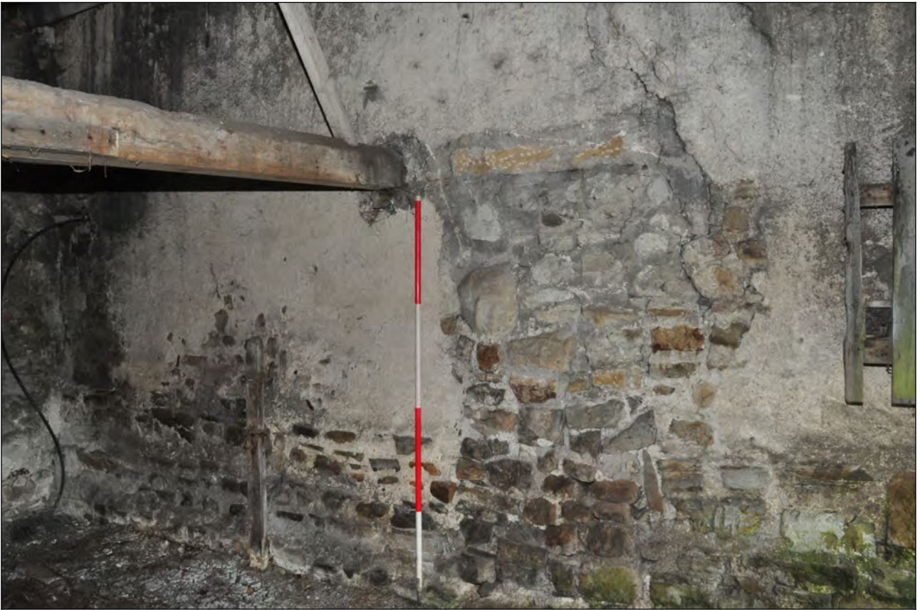
Photo 21: Main building: blocked doorway in east gable, within later lean-to
