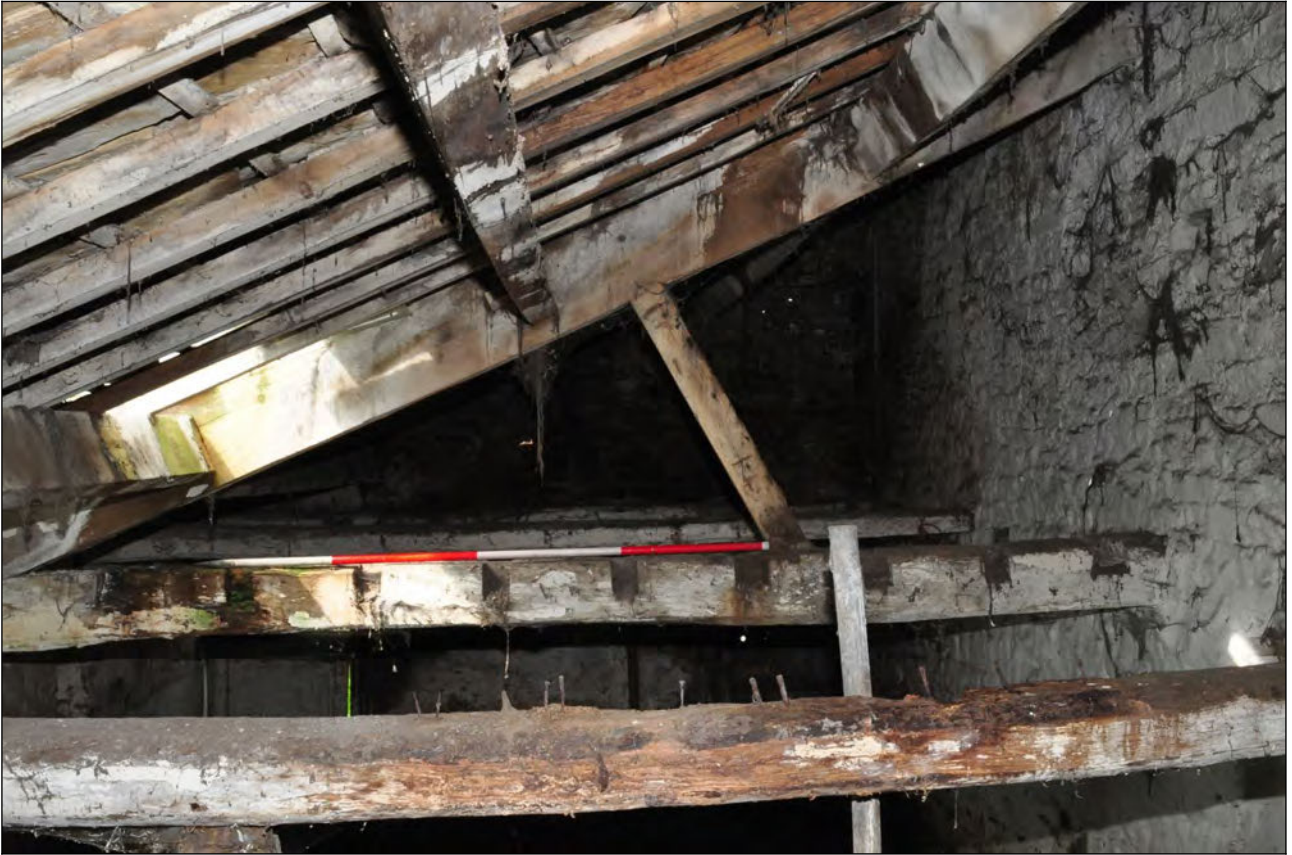
Photo 54: South shippon: interior, showing roof structure, looking west
