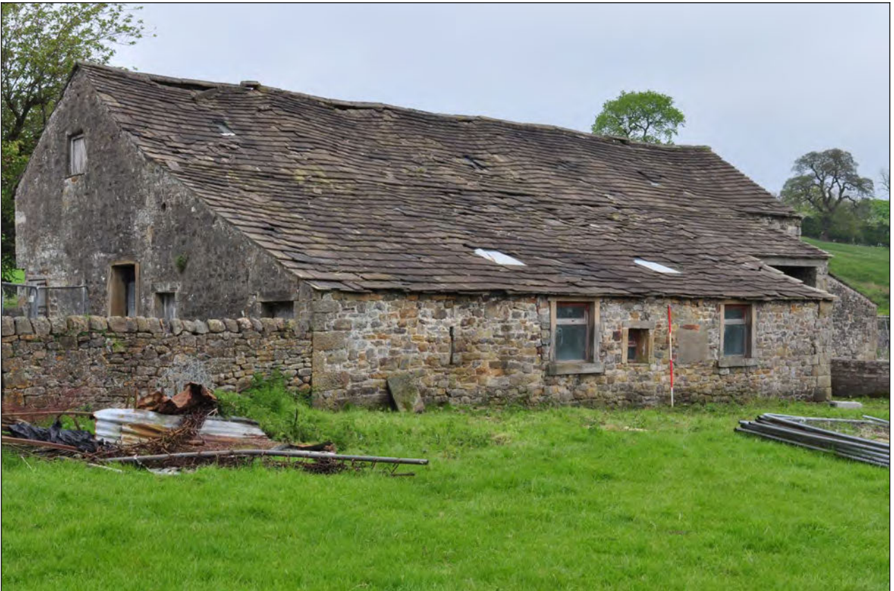
Photo 45: South shippon, looking north-east
