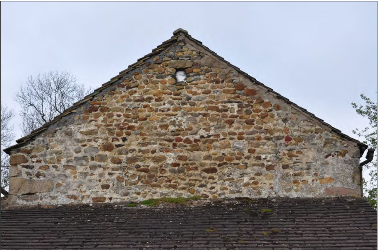
Photo 22: Main building: east gable
