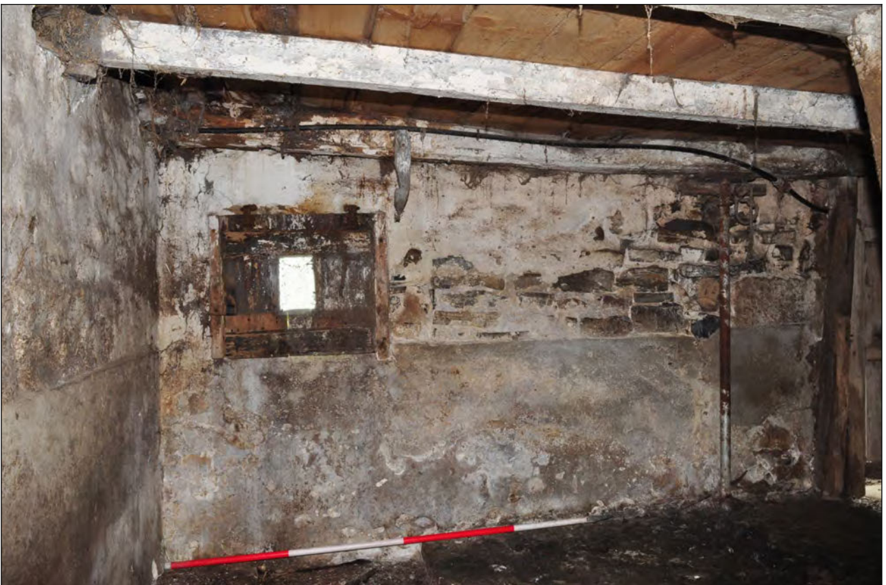
Photo 31: Main building: interior, detail of mucking-out hole in south side of shippon
