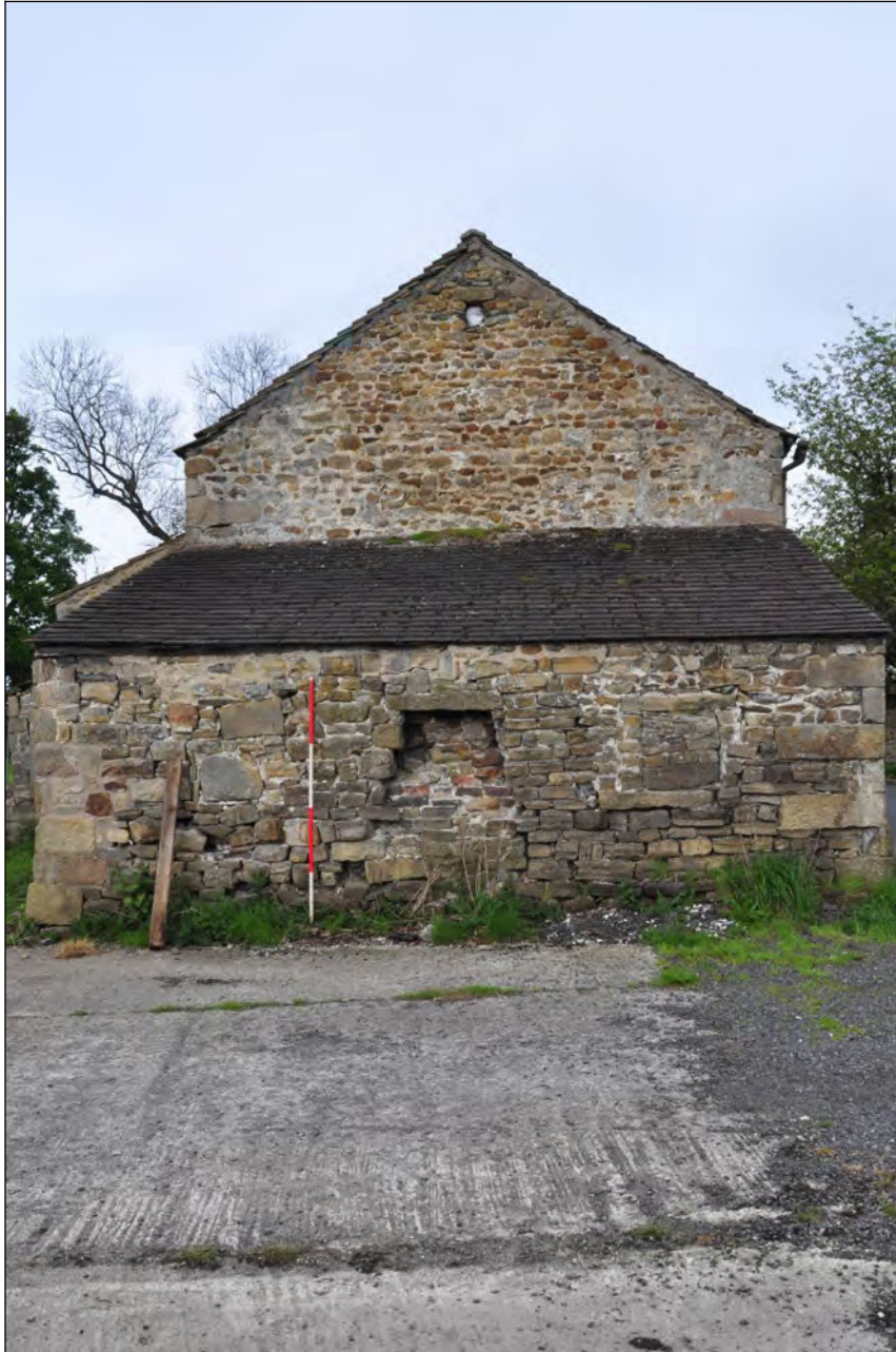
Photo 20: Main building: east gable
