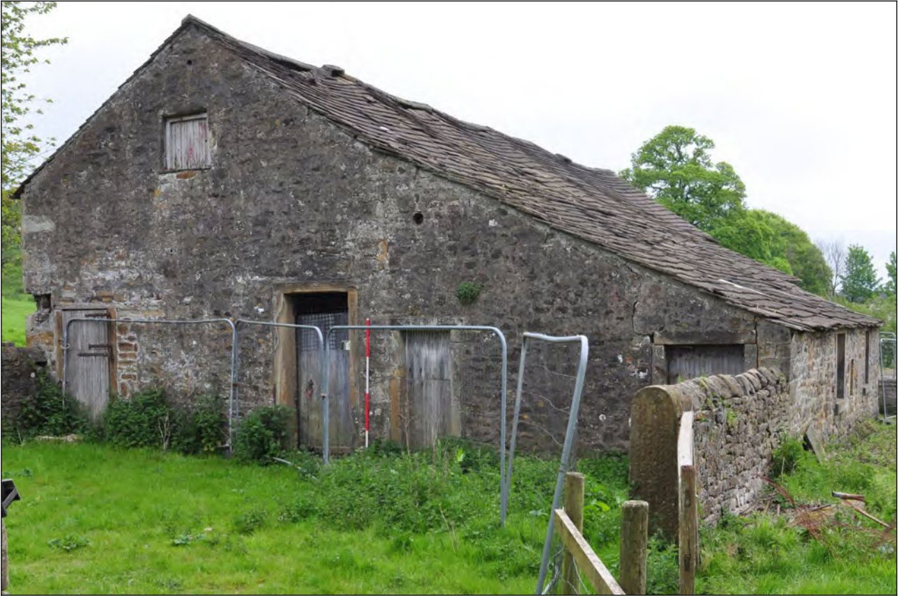
Photo 48: South shippon, looking north-east
