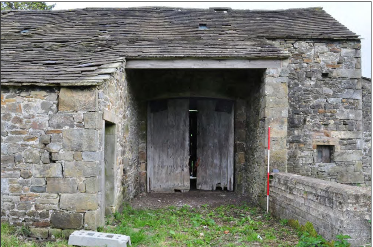
Photo 16: Added porch on south side, looking north
