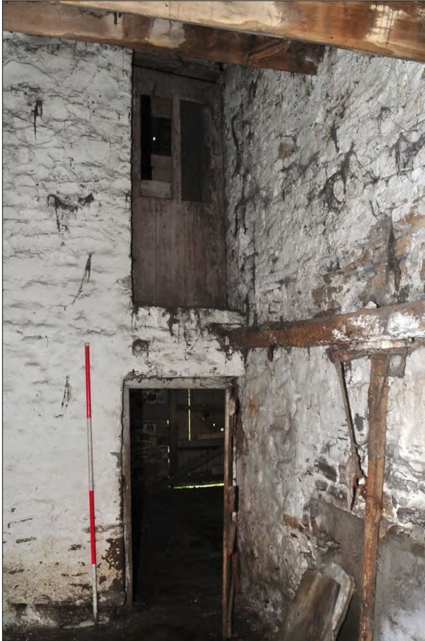
Photo 18: Main building: inserted doorways in south side, within later shippon
