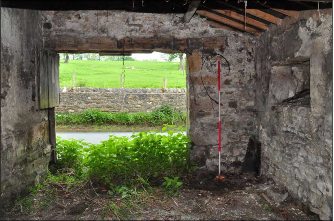
Photo 60: East lean-to: interior, looking north
