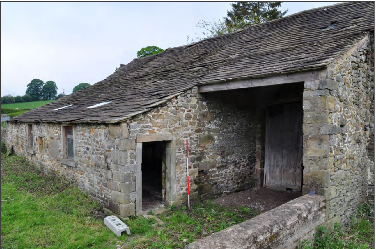
Photo 47: South shippon, looking north-west
