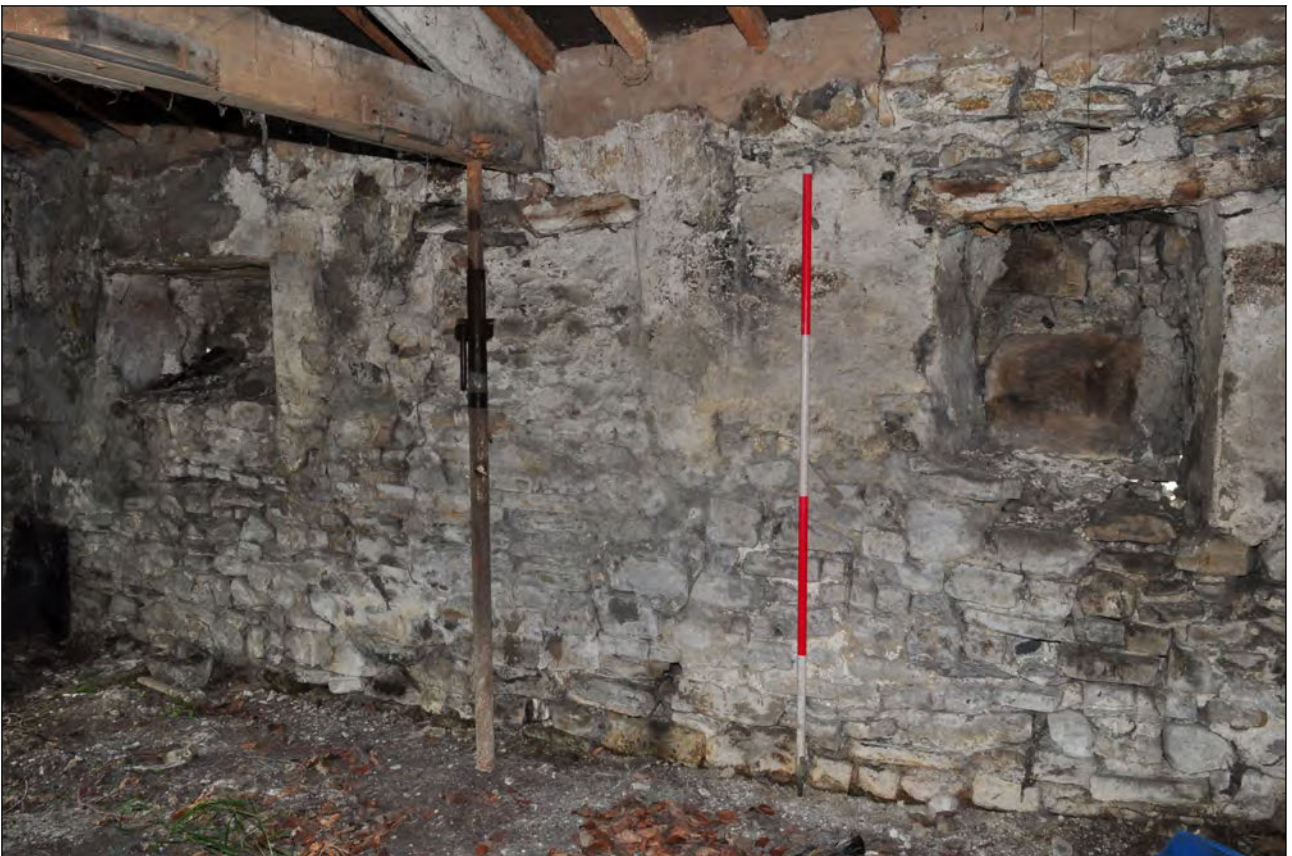
Photo 59: East lean-to: interior, looking north-east
