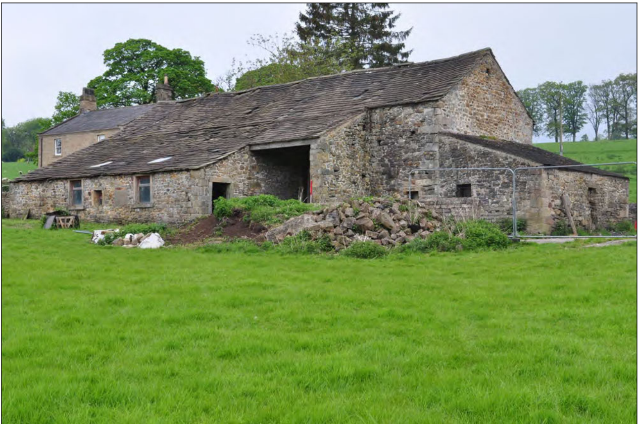
Photo 2: General view, looking north-west
