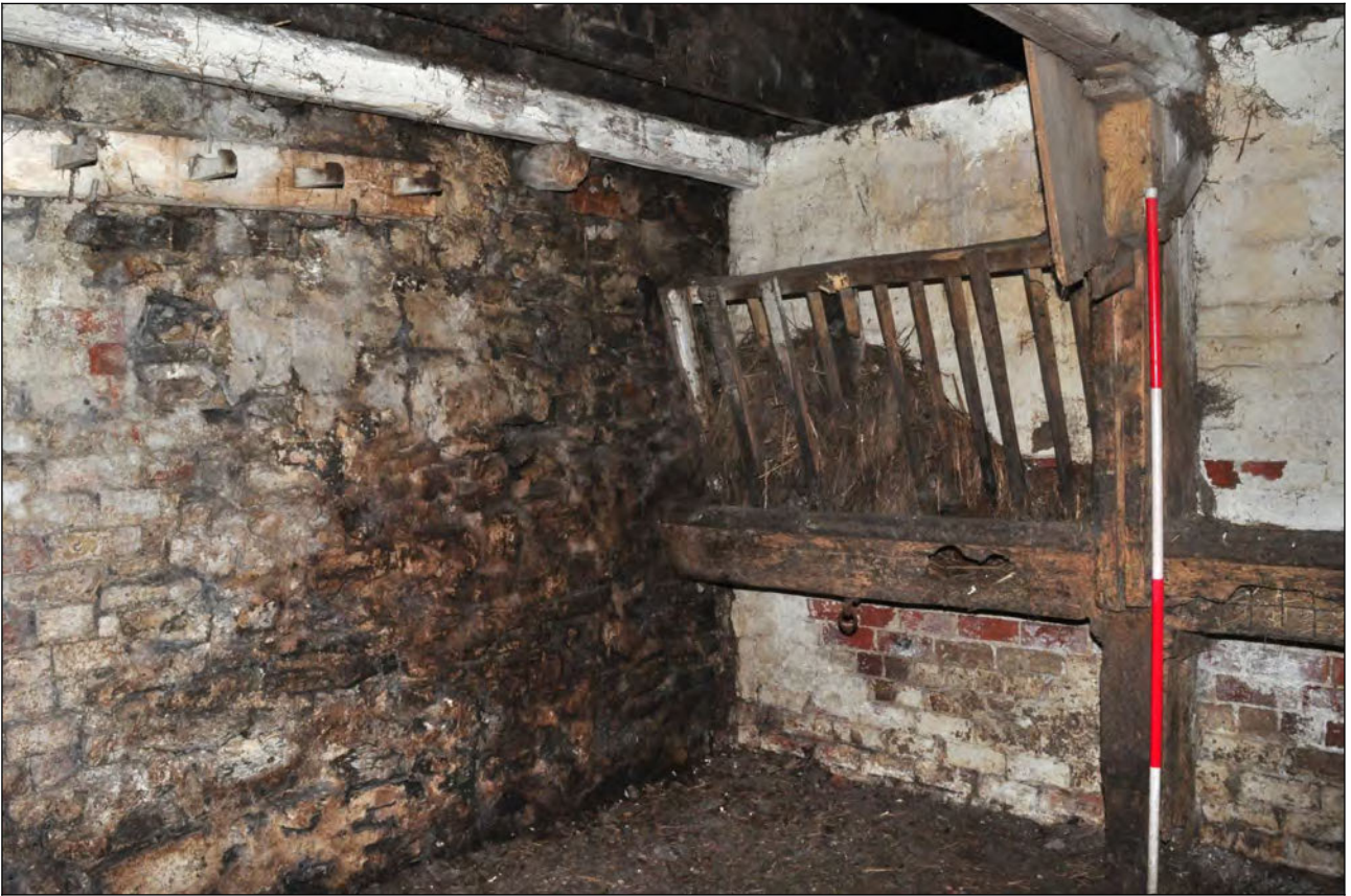
Photo 40: Main building: stable at west end, looking north-west
