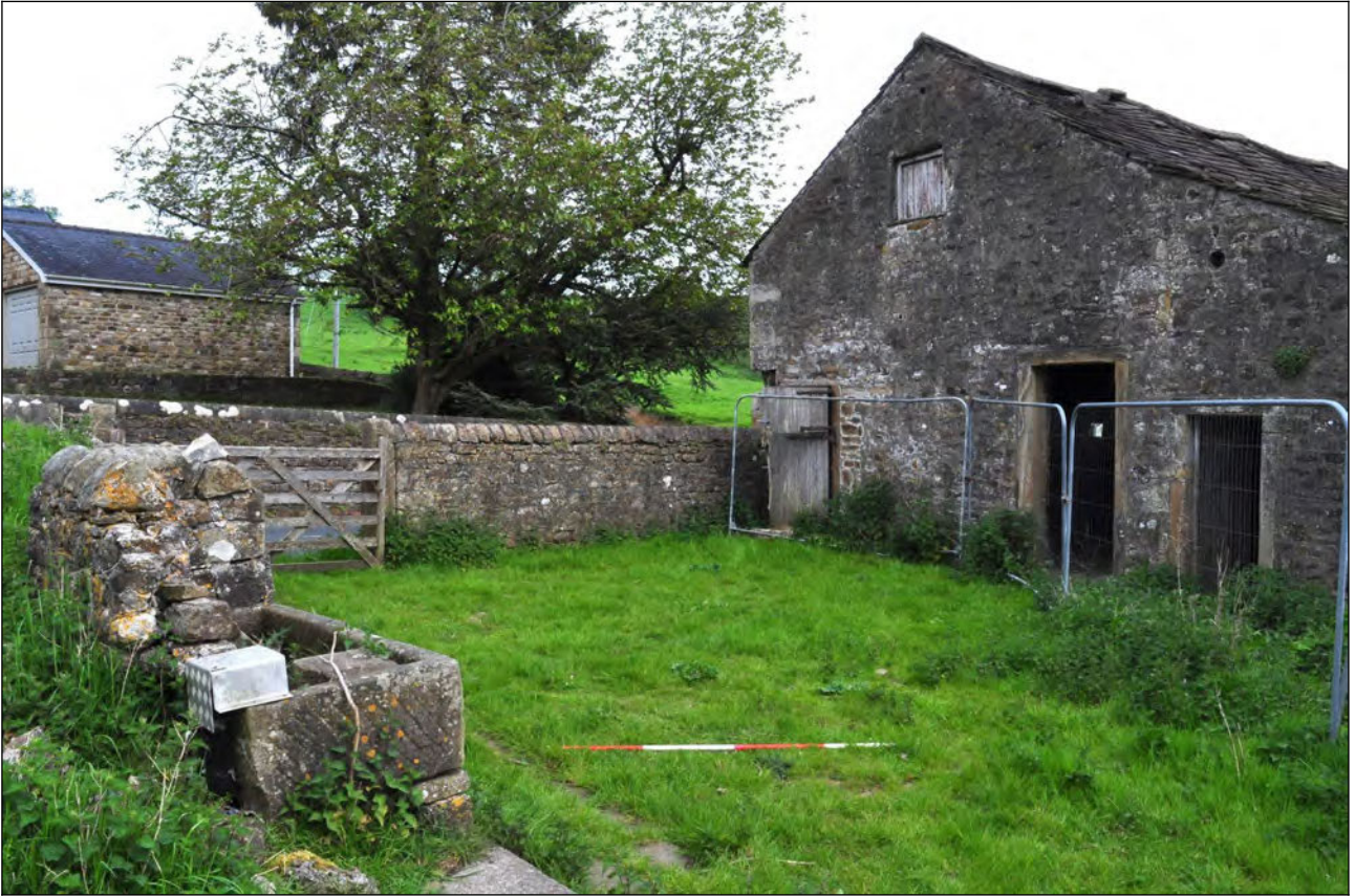
Photo 13: Fold-yard at west end of building, looking north-east
