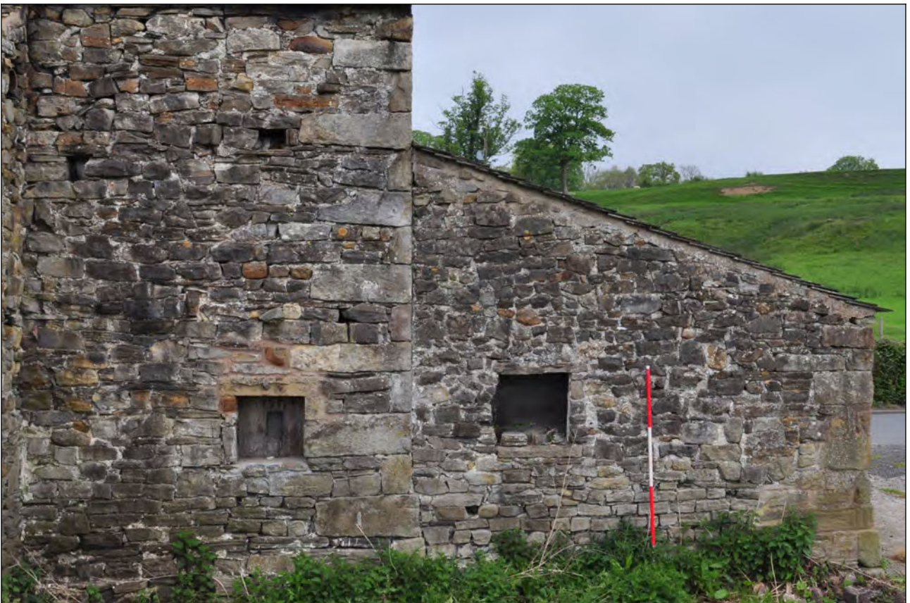
Photo 57: East lean-to: south side
