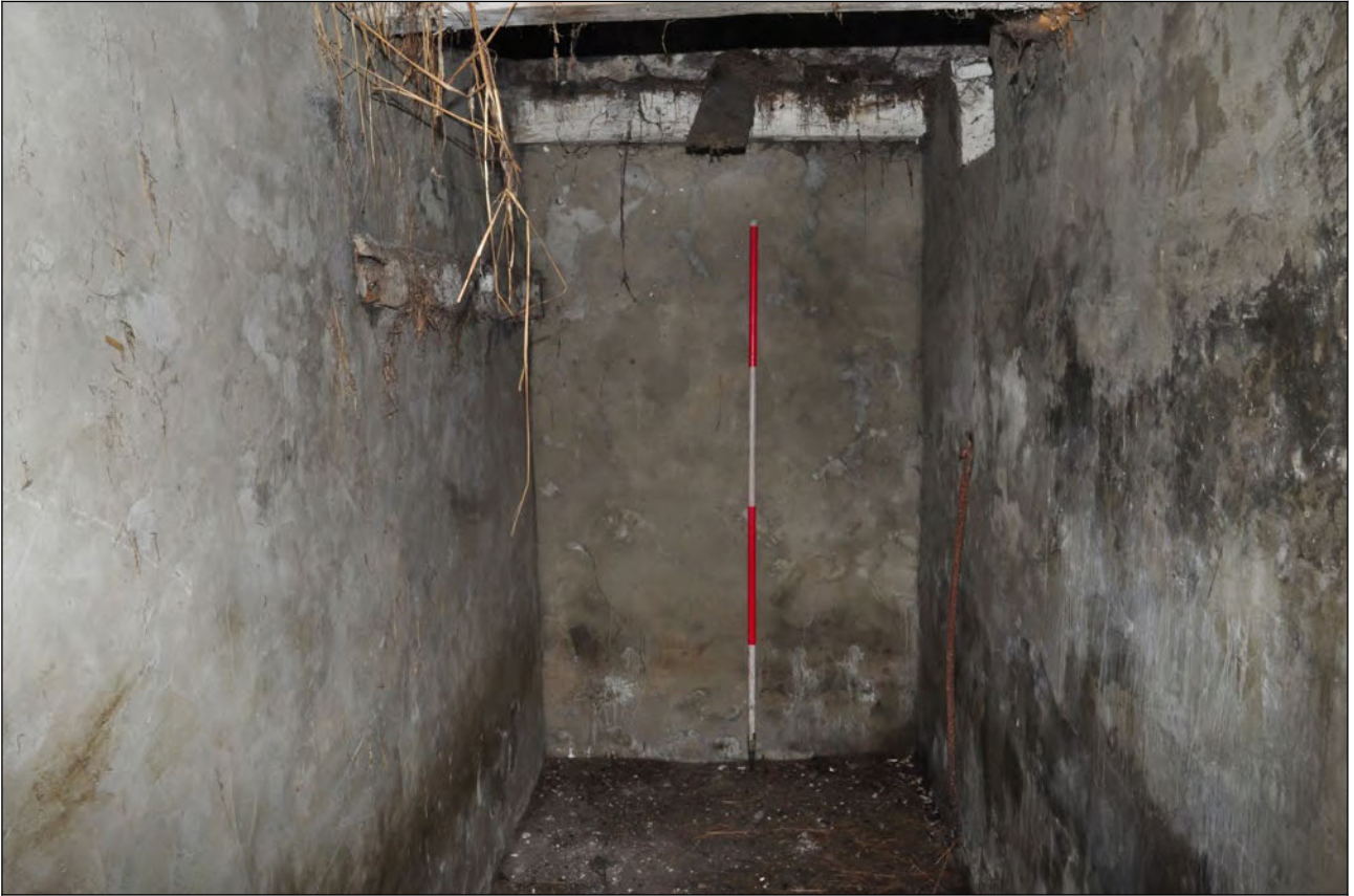
Photo 44: Main building: rendered cell at north-west corner, looking east
