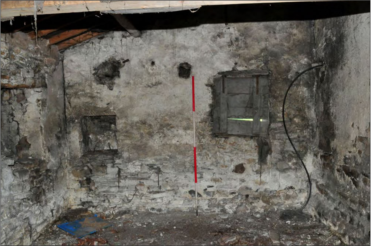
Photo 58: East lean-to: interior, looking south
