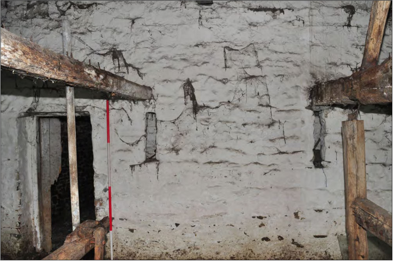
Photo 19: Main building: breathers in south side, within later shippon
