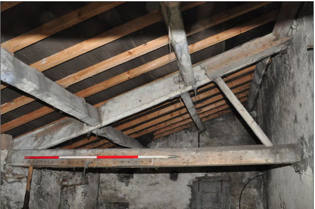
Photo 61: East lean-to: interior, roof structure, looking south
