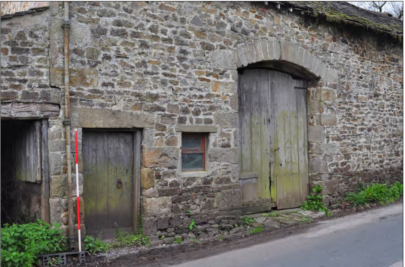
Photo 8: Main building: cart entrance and shippon doorway, north elevation
