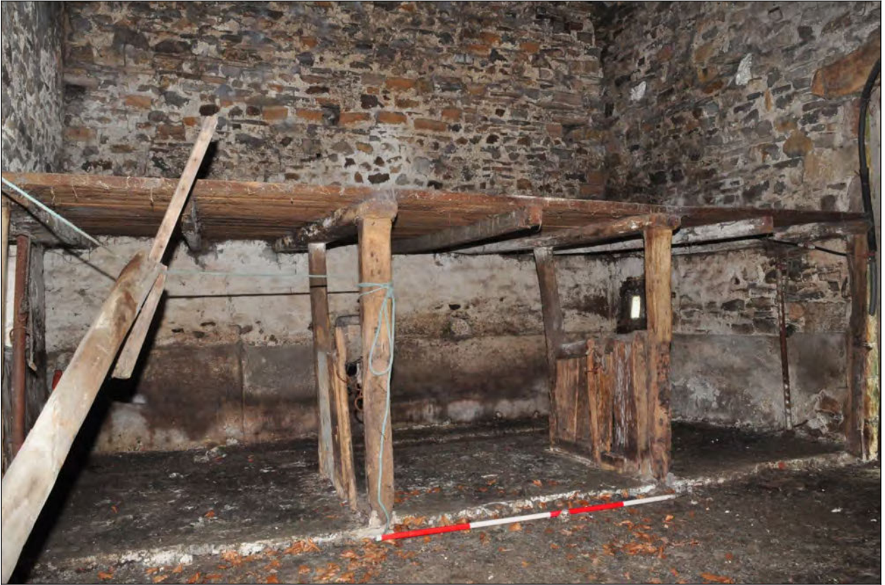
Photo 28: Main building: interior, looking south-east towards shippon
