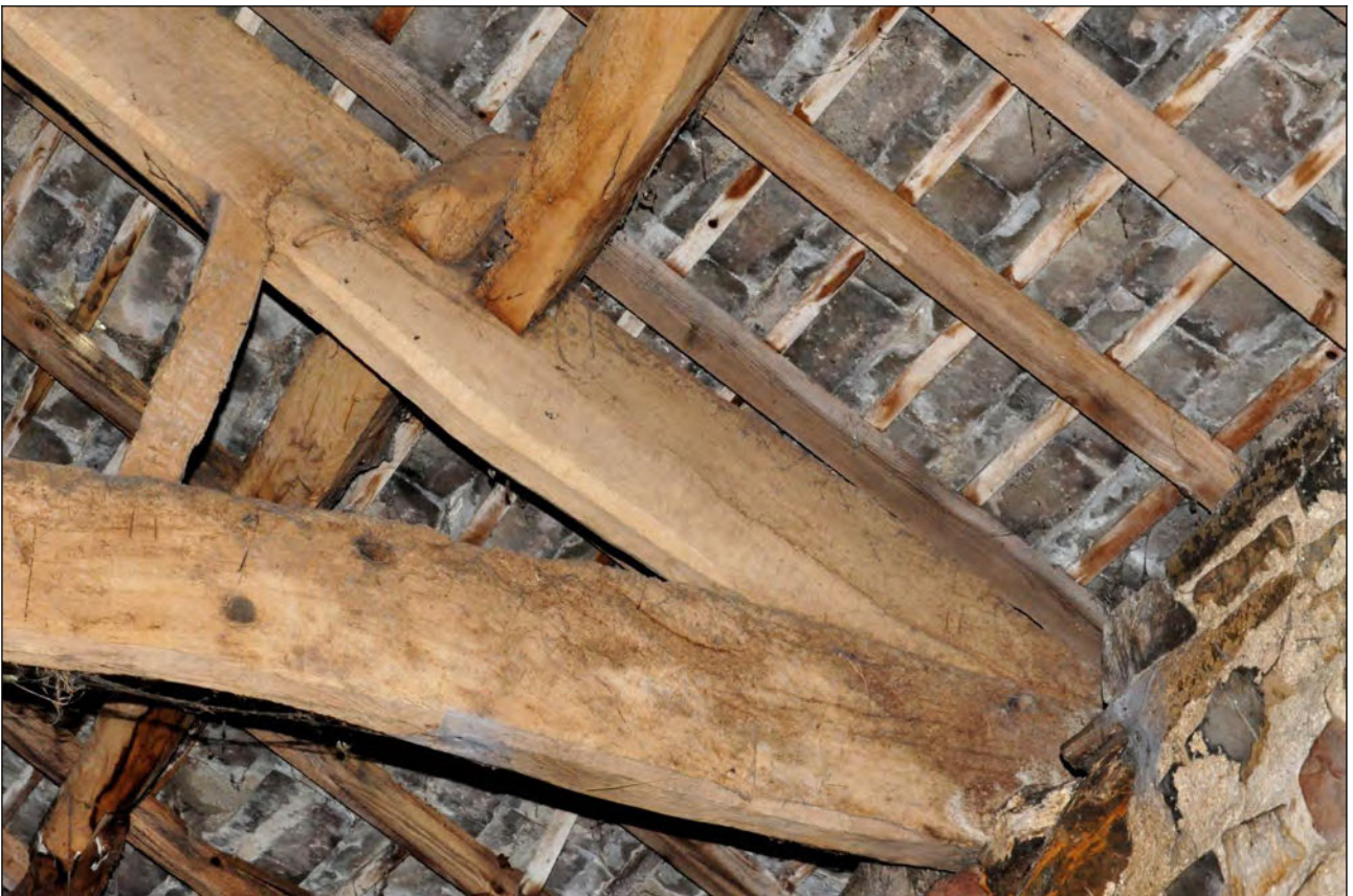
Photo 37: Main building: detail of north end of roof truss, looking west
