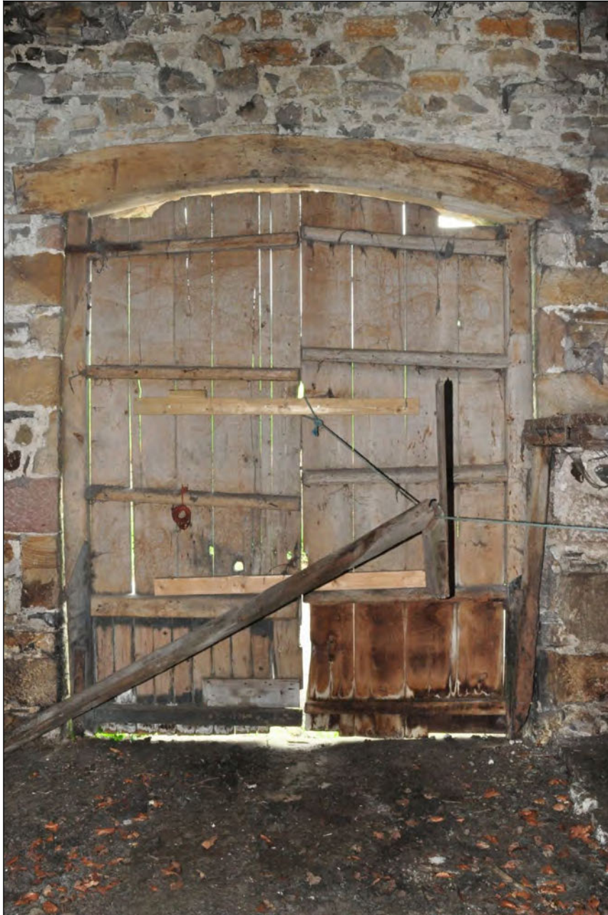
Photo 25: Main building: interior view of north cart entrance
