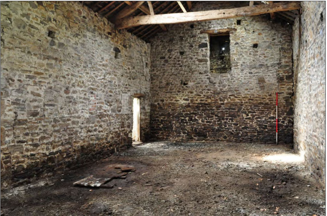
Photo 33: Main building: interior, looking south-west
