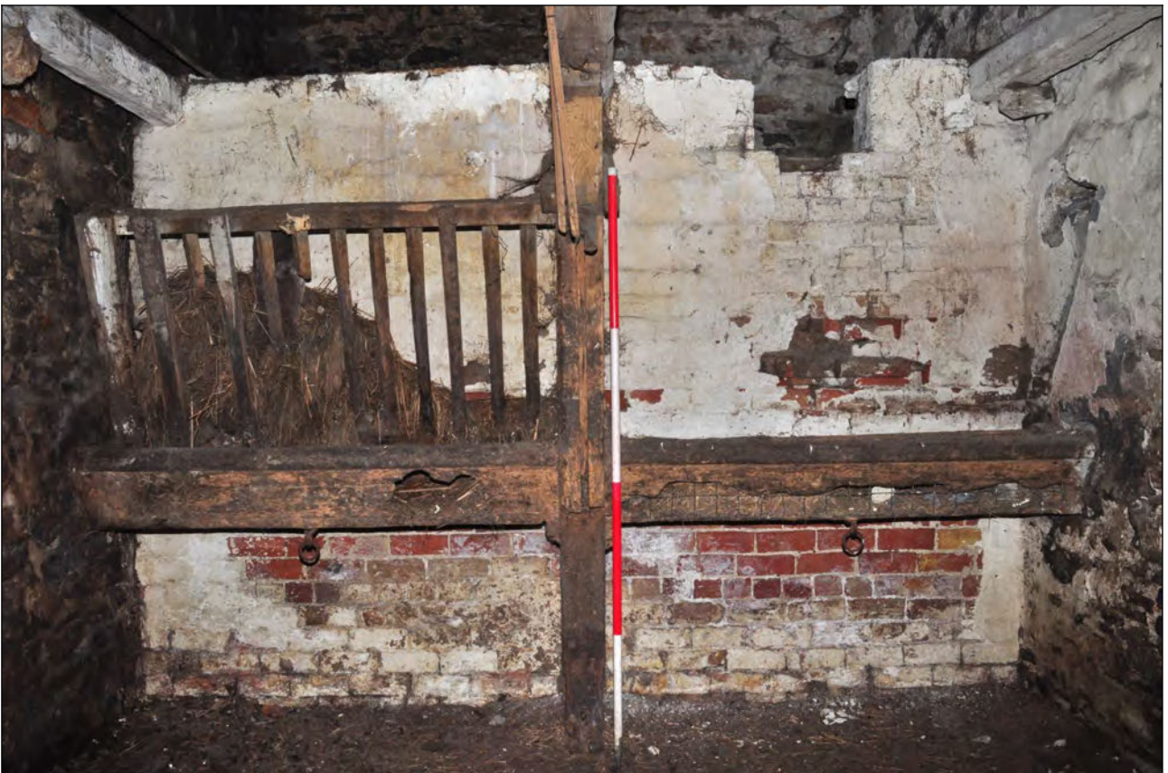
Photo 39: Main building: stable at west end, looking north
