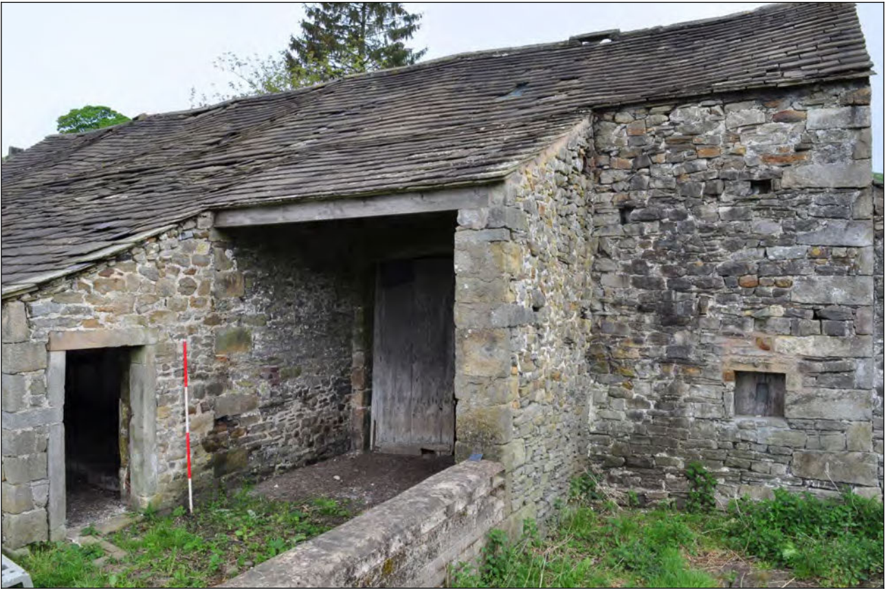
Photo 15: Added porch on south side, looking north-west
