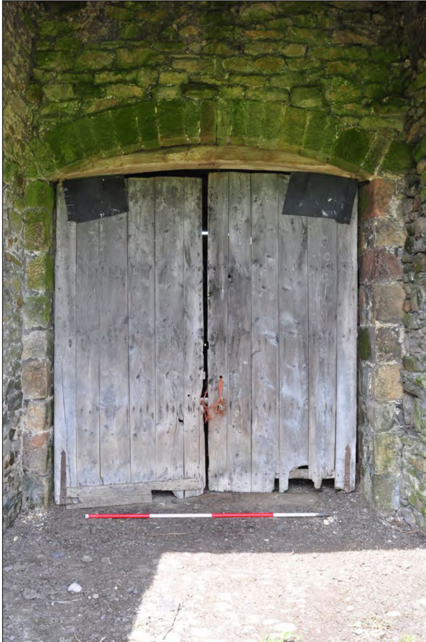
Photo 17: Main building: cart entrance, south elevation
