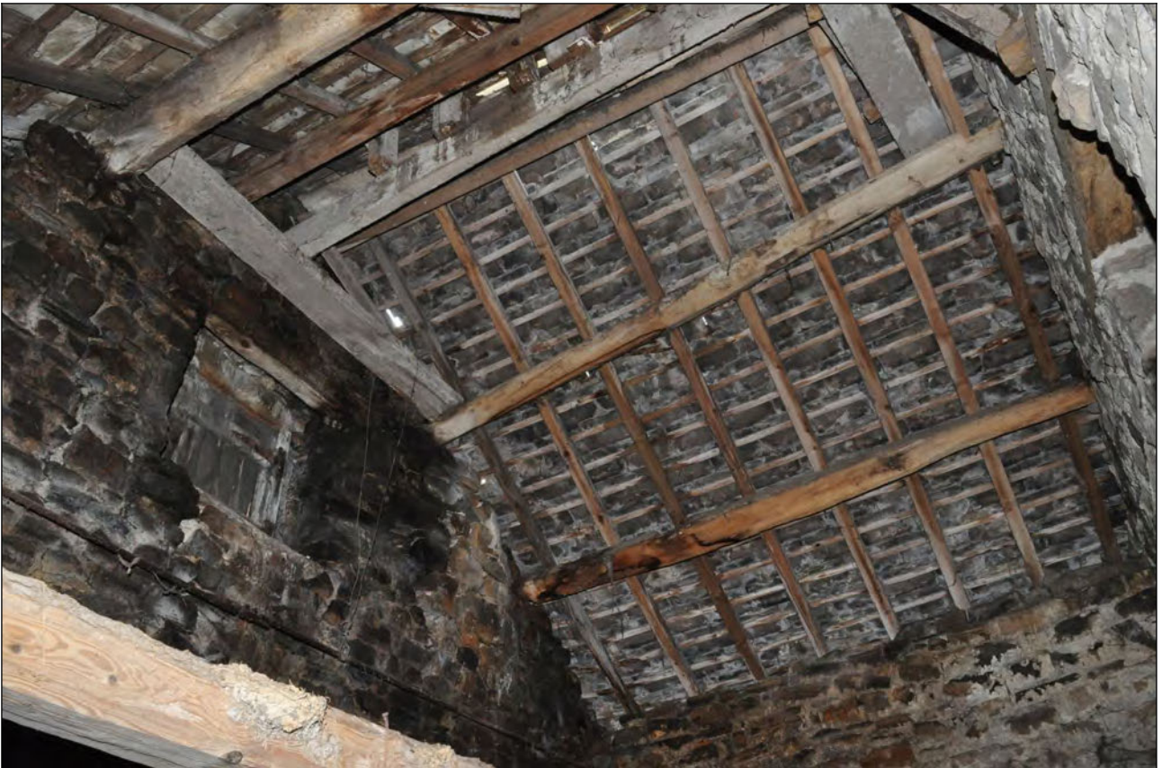
Photo 43: Main building: roof over stable at west end, looking south-east
