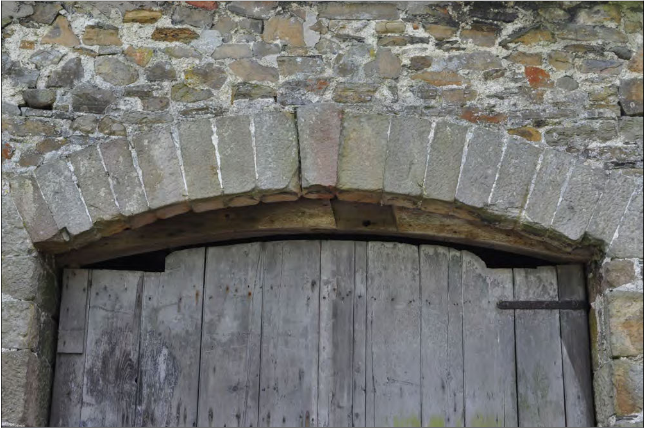
Photo 7: Main building: arch over cart entrance, north elevation
