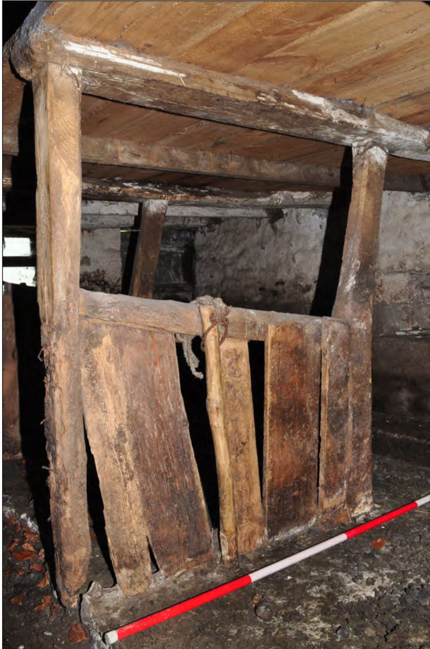
Photo 29: Main building: interior, detail of boskin in shippon, looking north-east
