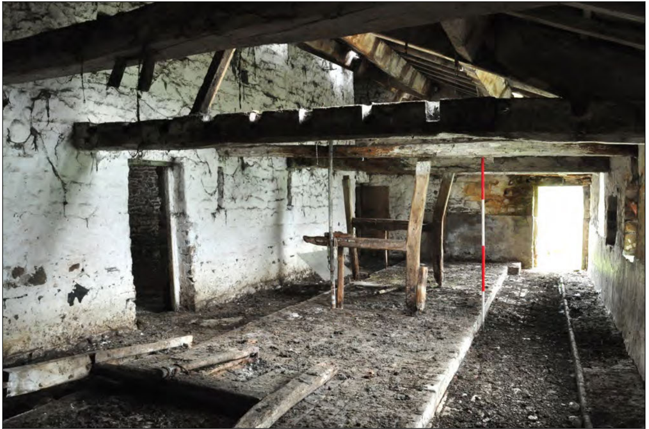
Photo 50: South shippon: interior, looking north-east
