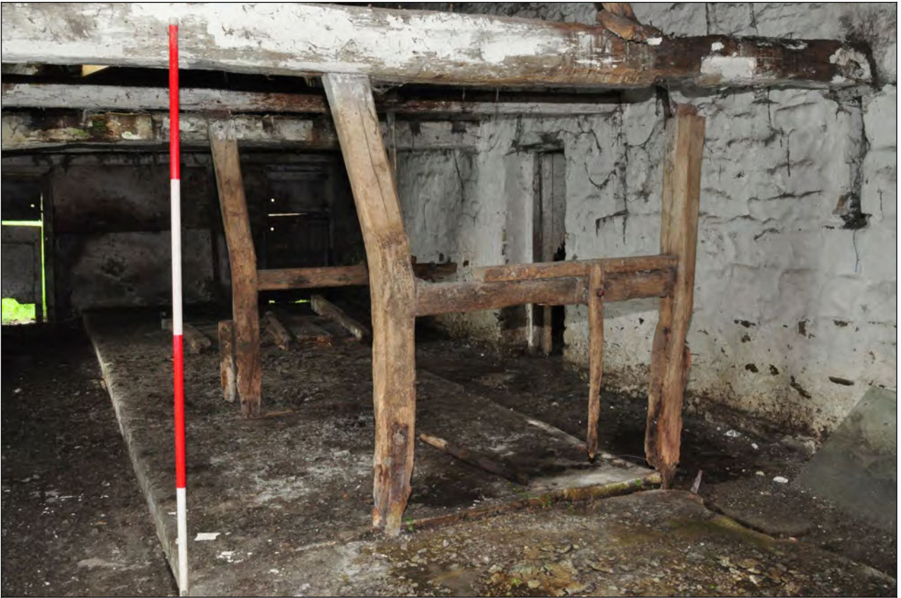
Photo 52: South shippon: interior, remains of boskins, looking north-west
