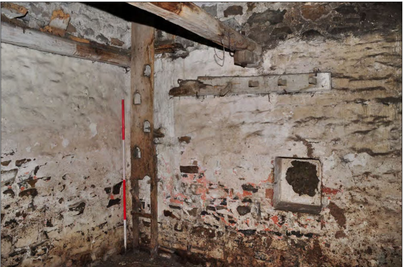
Photo 41: Main building: stable at west end, looking south-east
