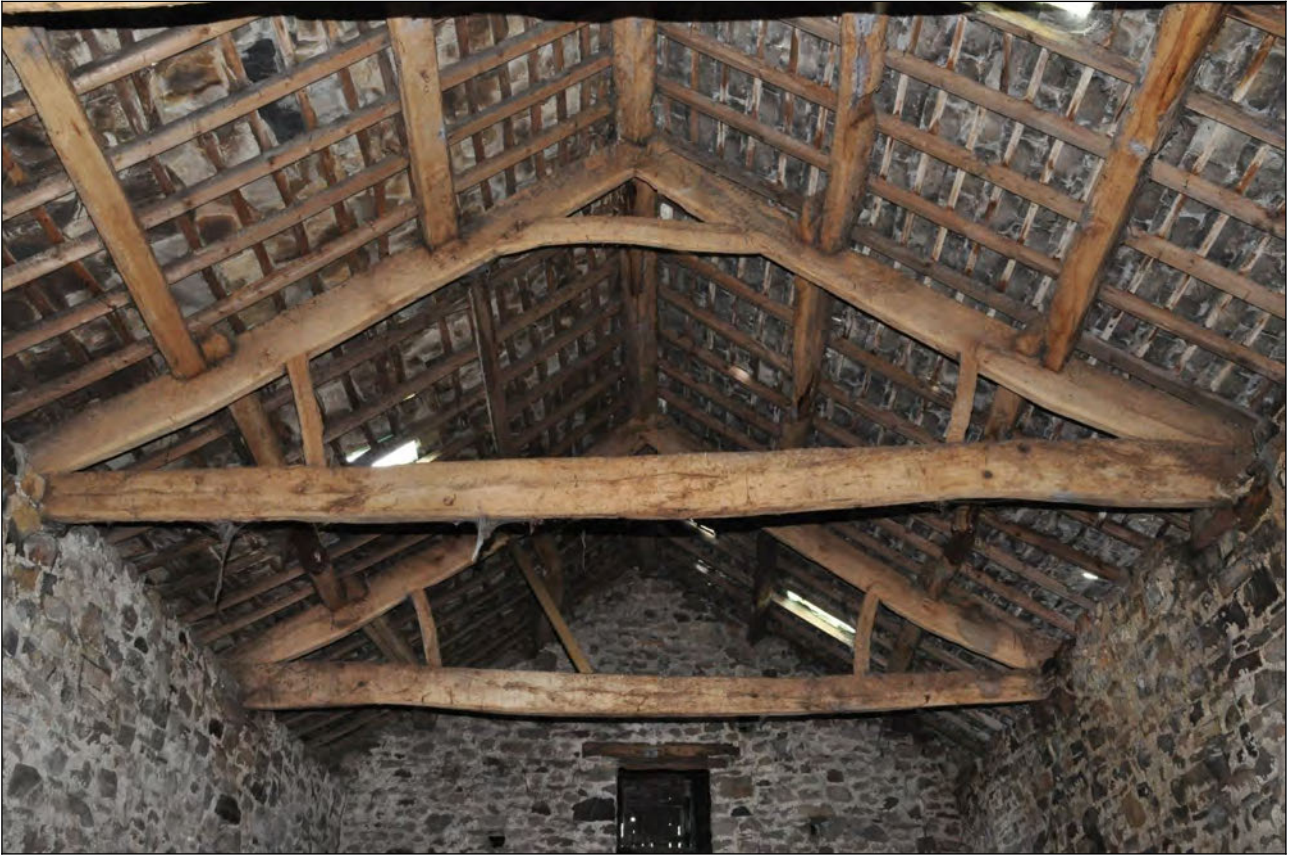
Photo 36: Main building: western roof trusses, looking west
