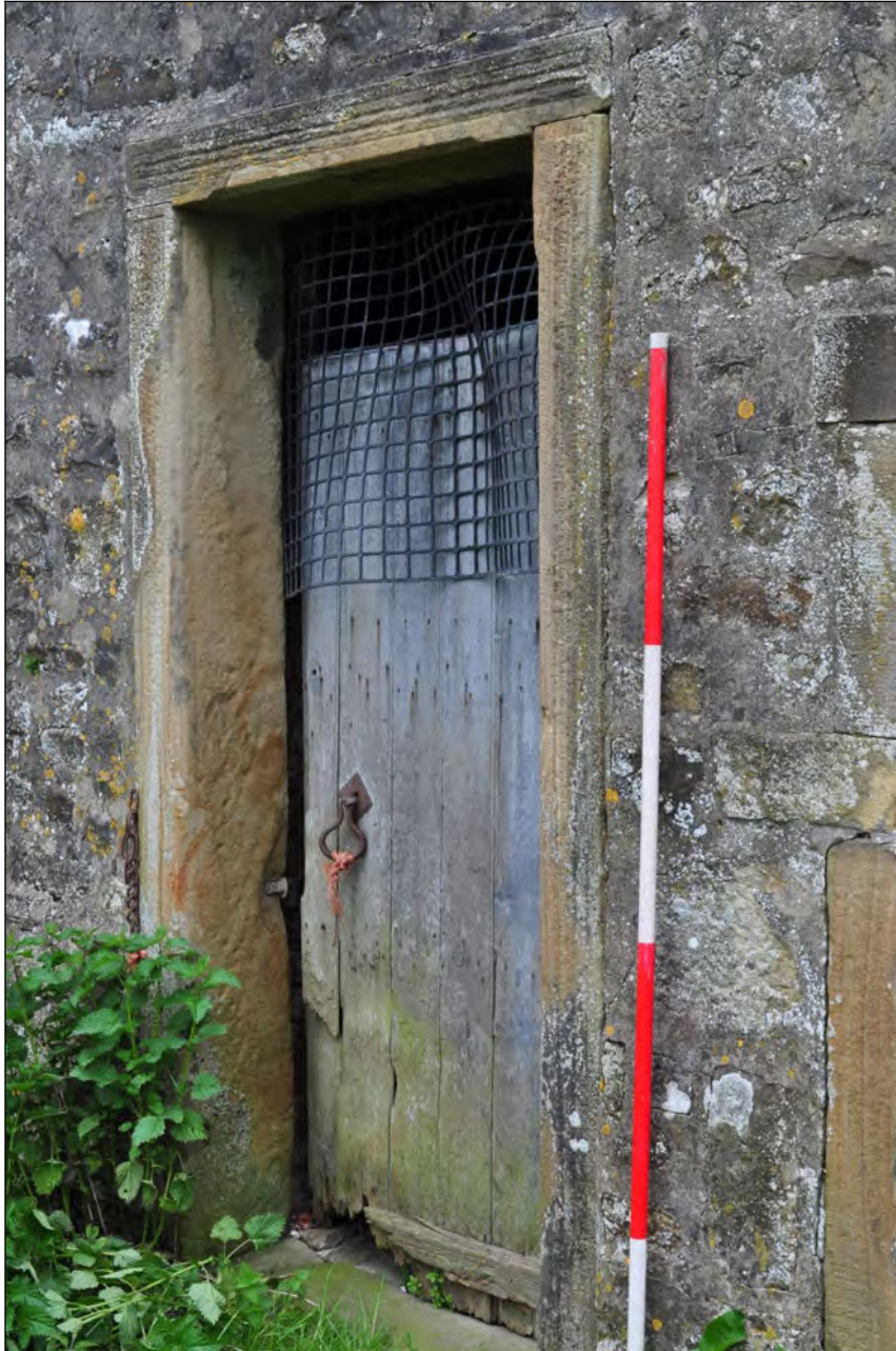
Photo 12: Main building: stable doorway, west elevation
