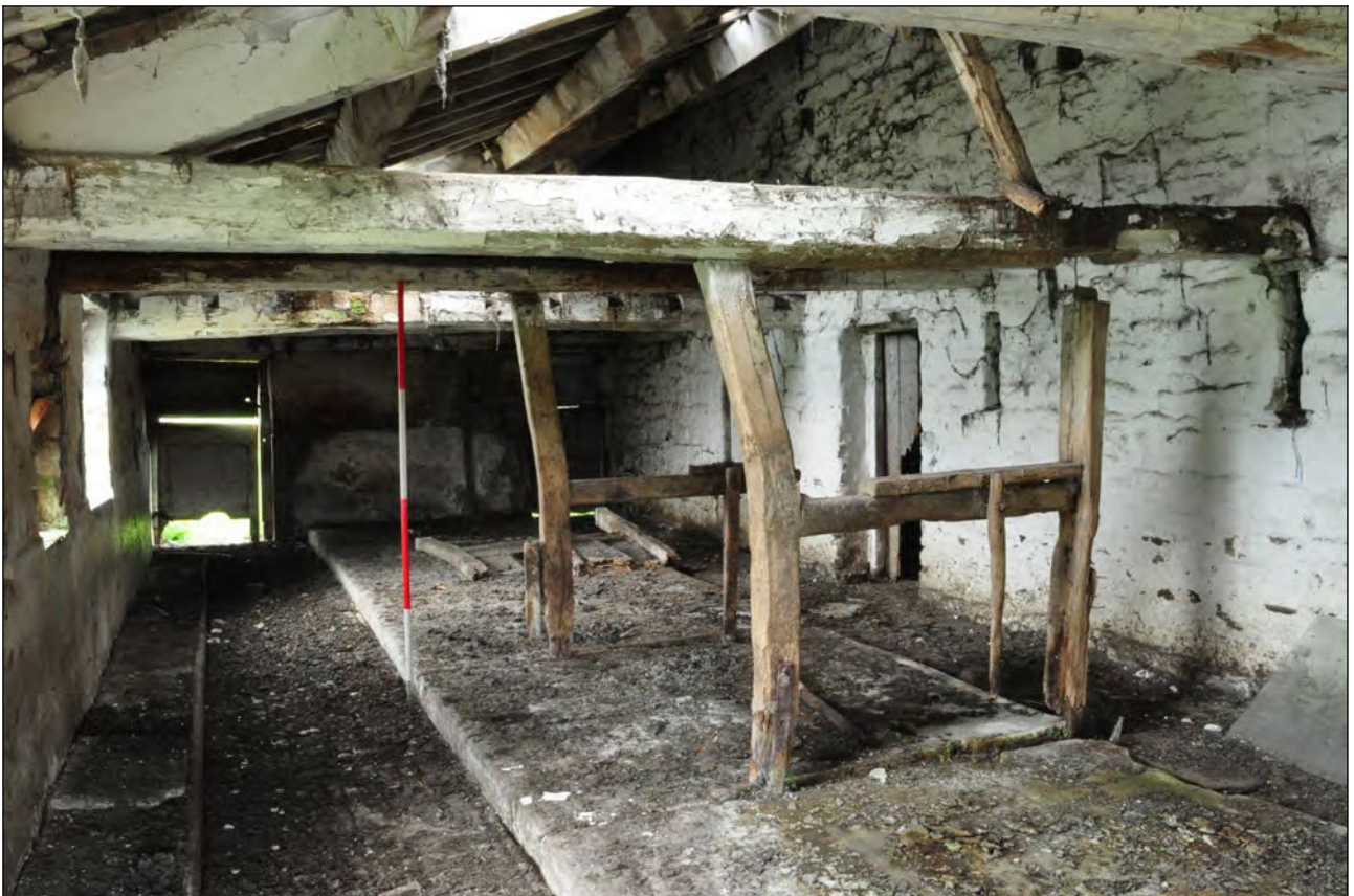
Photo 51: South shippon: interior, looking north-west
