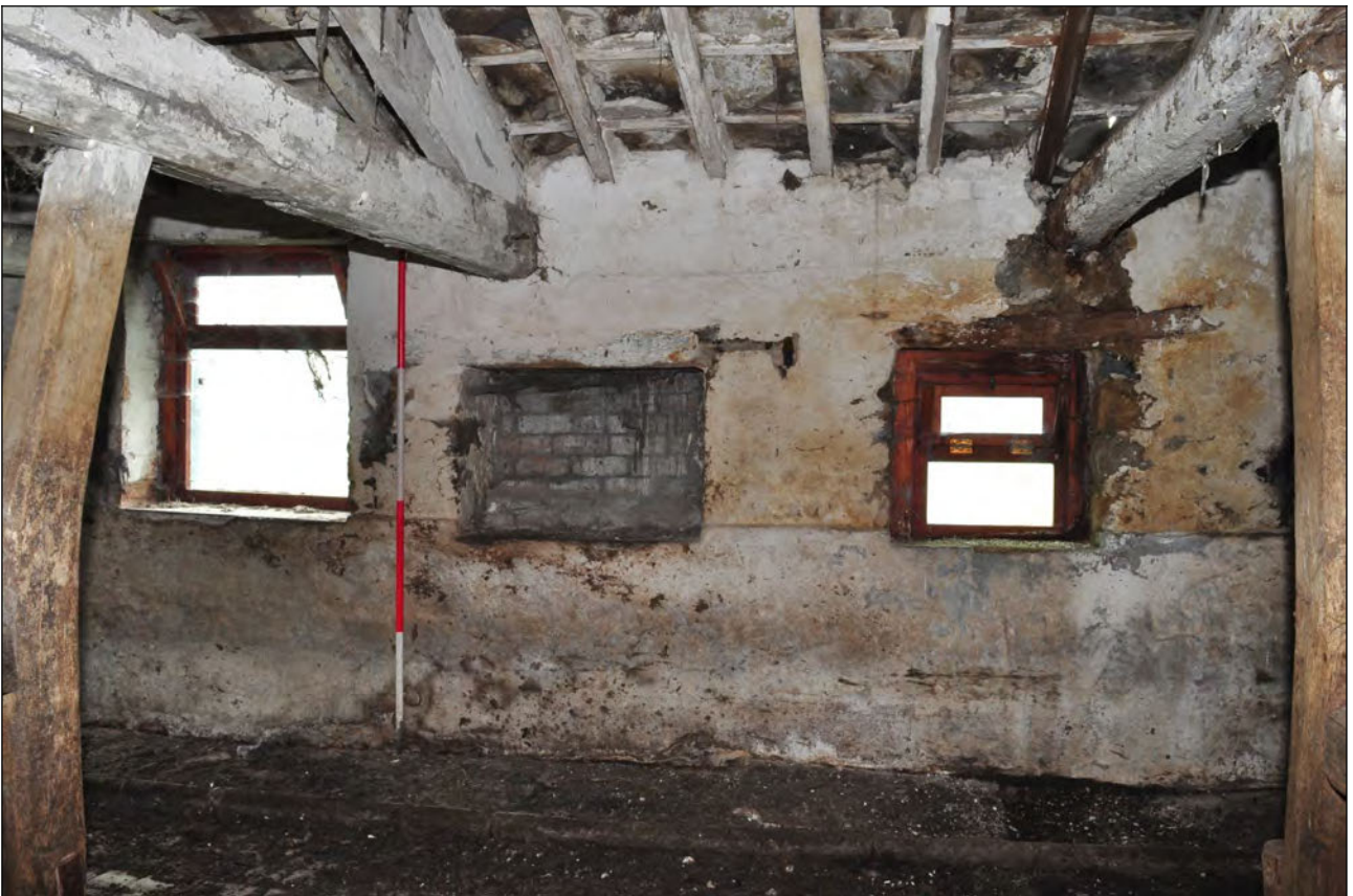
Photo 53: South shippon: interior, openings in south wall
