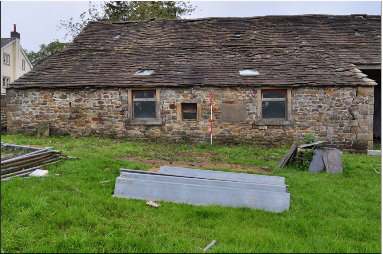
Photo 46: South shippon, looking north
