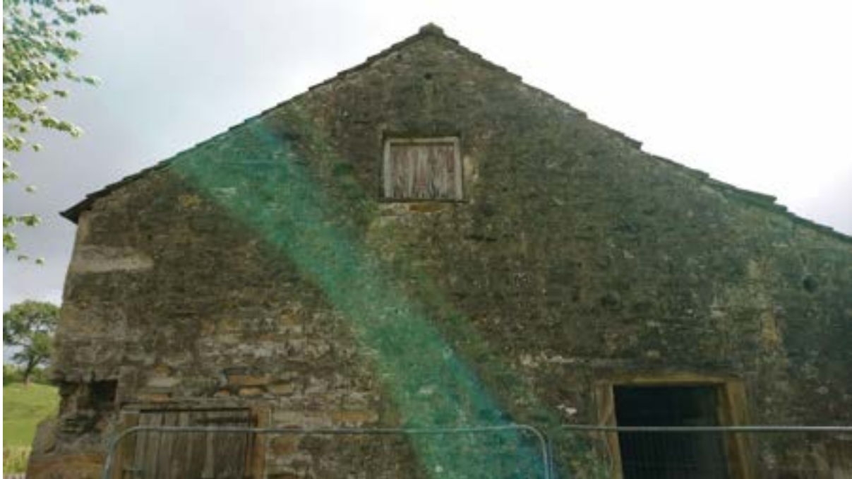
Figure 32: External view of WP5.
