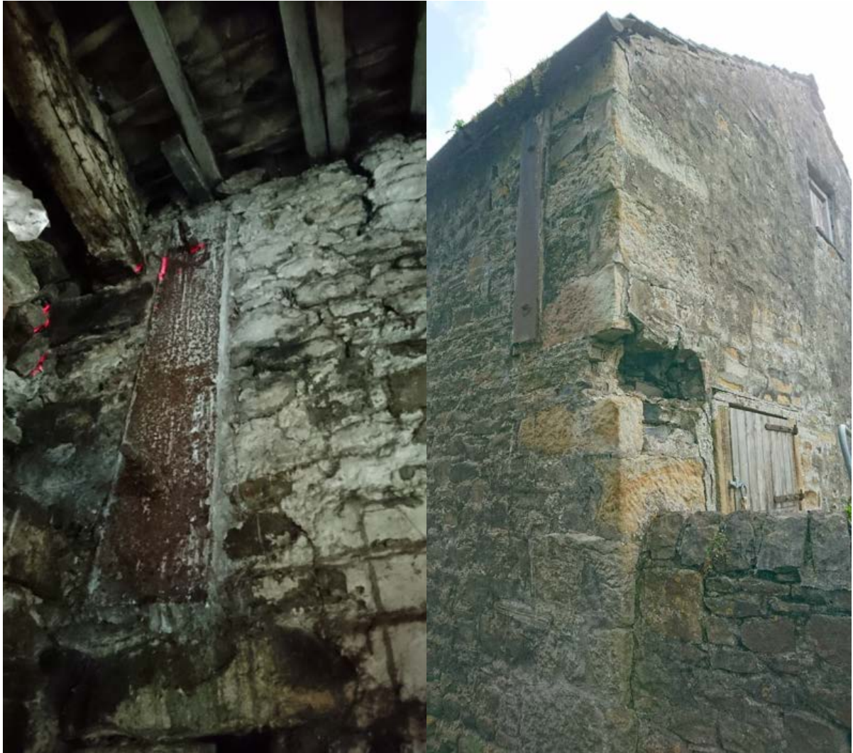
Figure 14: Steel parrass plates in WP 3 (image left) and WP1 (image right)
