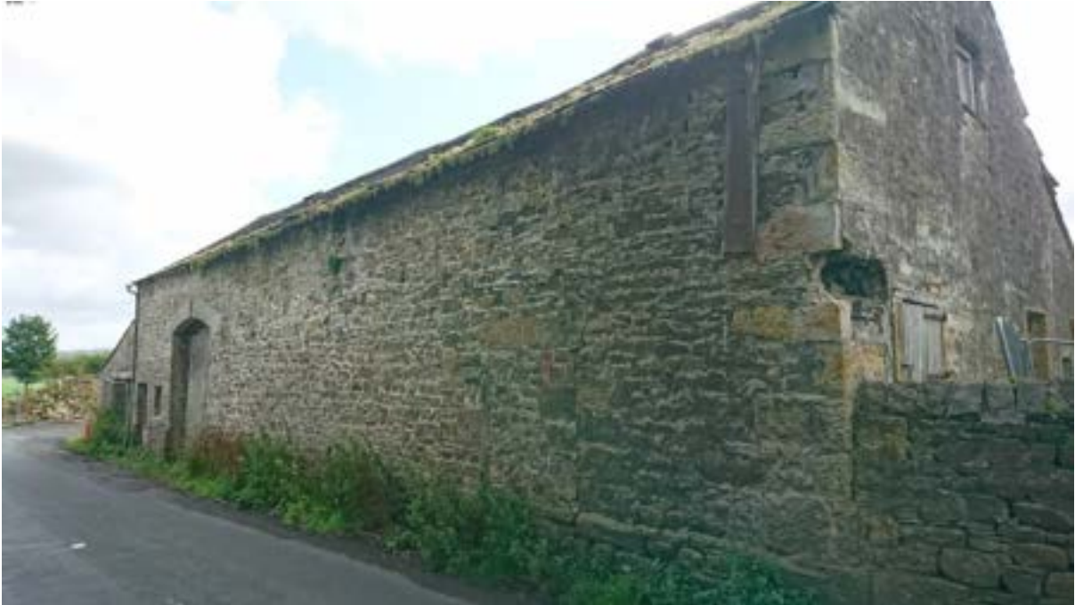
Figure 18: External view of WP1.
