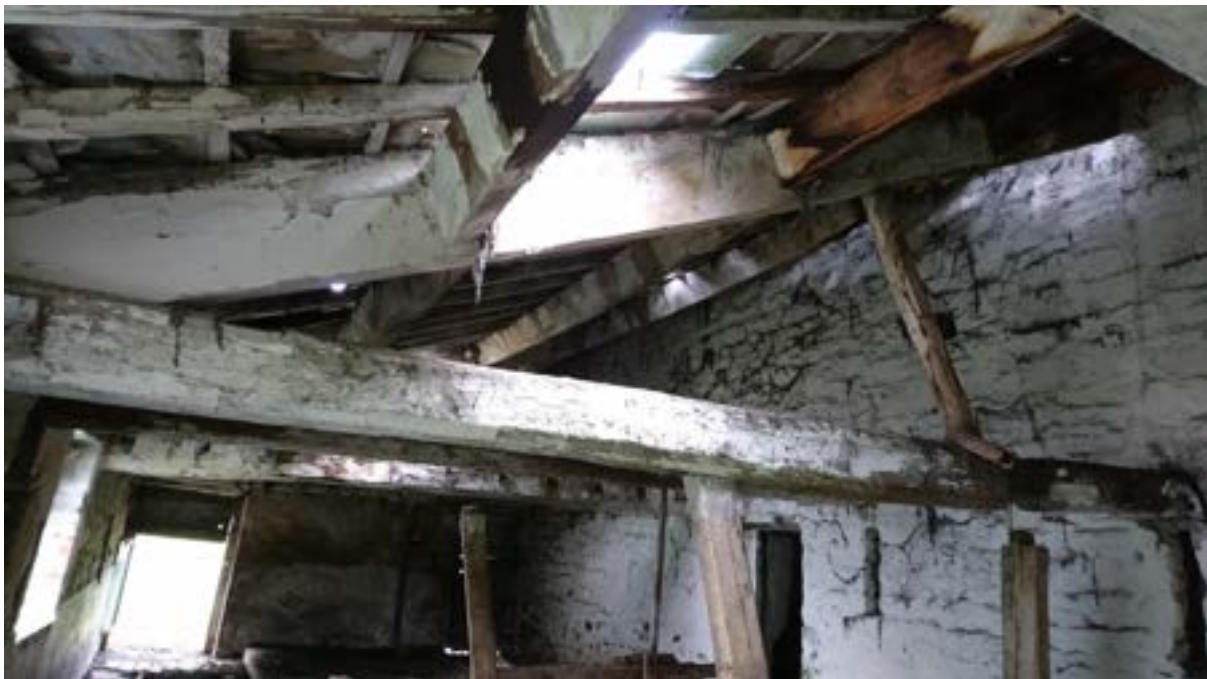
Figure 10: Typical internal view of the roof structure in Extension 2.
