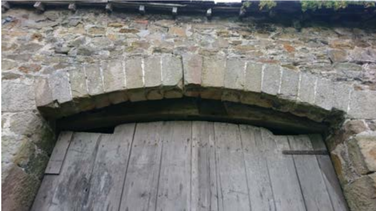
Figure 21: Masonry arch lintel.
