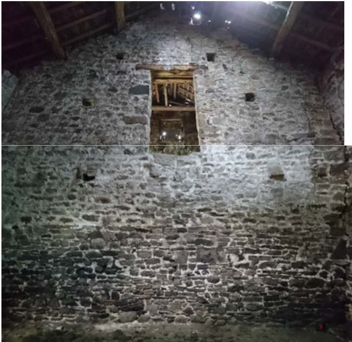
Figure 30: WP4 viewed from the Main Barn.
