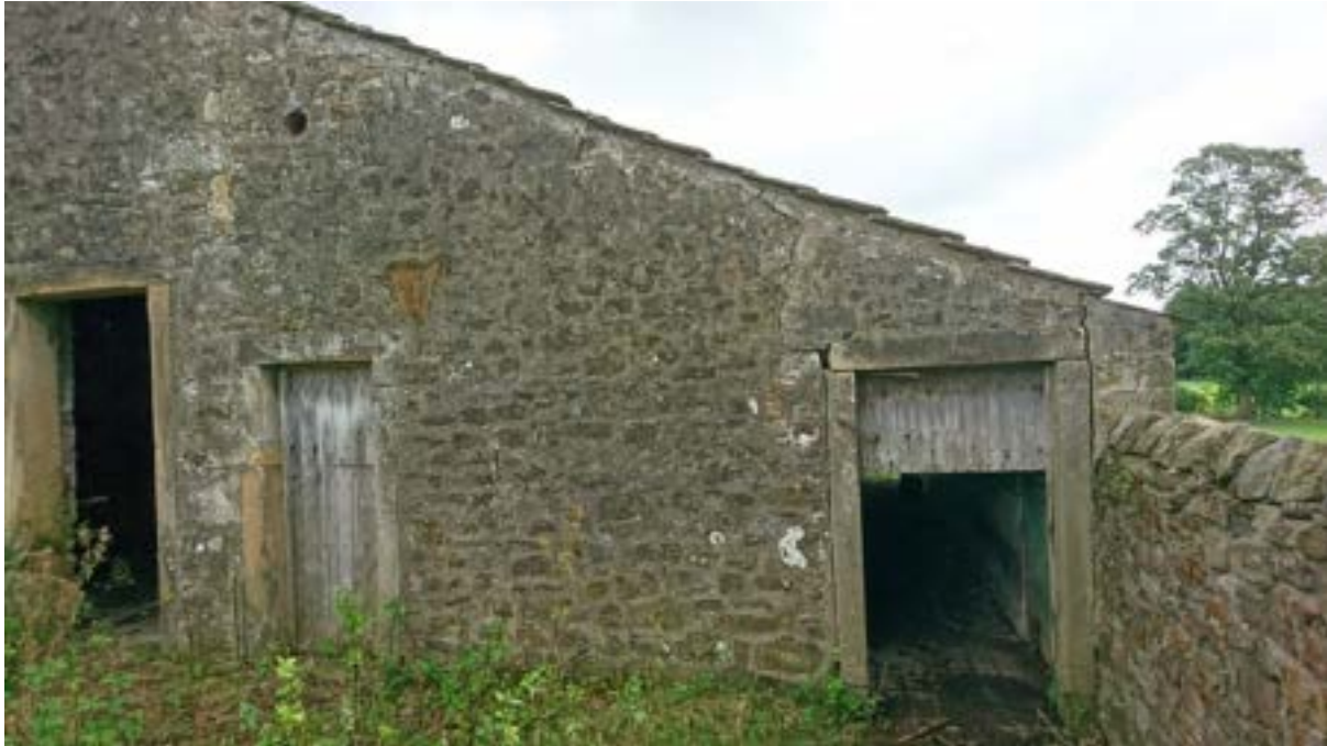
Figure 42: External view of WP6.
