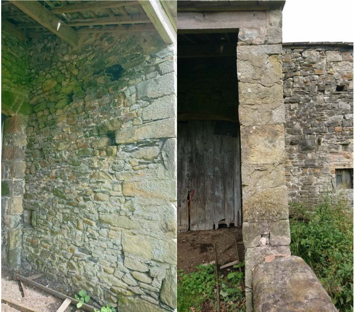
Figure 50: WP 9, straight and plumb.
