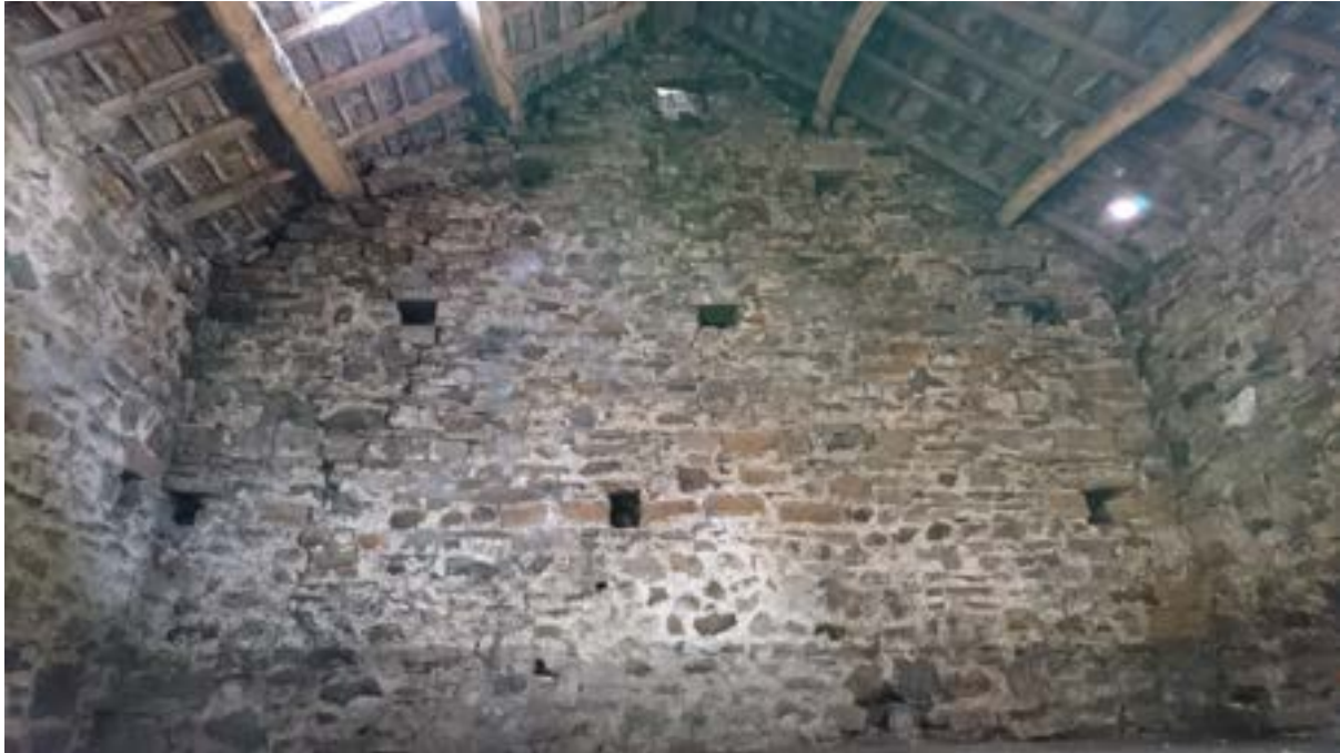
Figure 22: WP2 viewed from the main barn.
