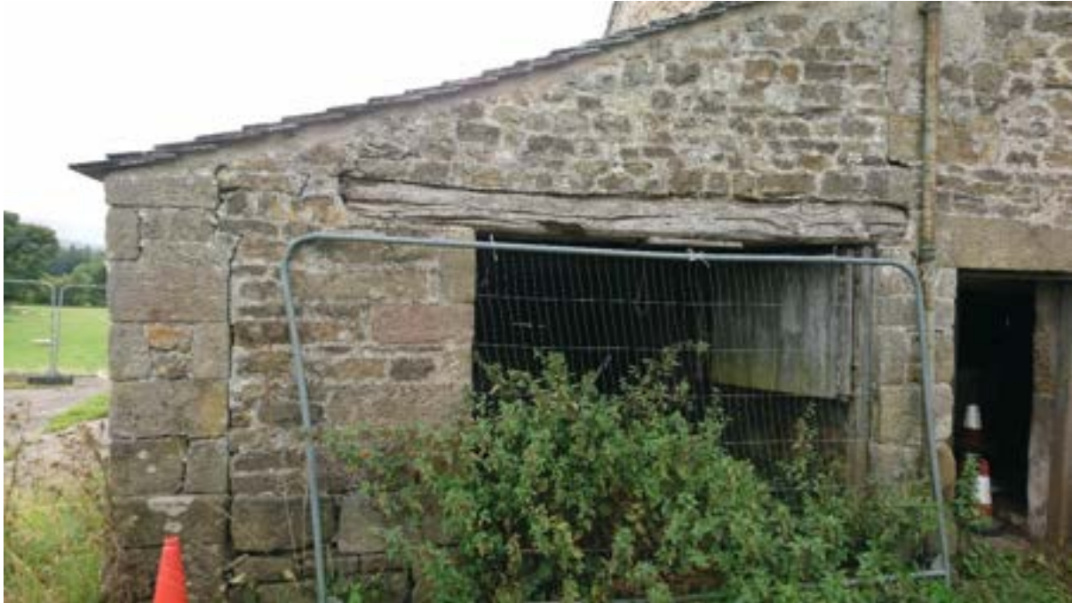
Figure 40: WP12 - the northern elevation of Extension 1.
