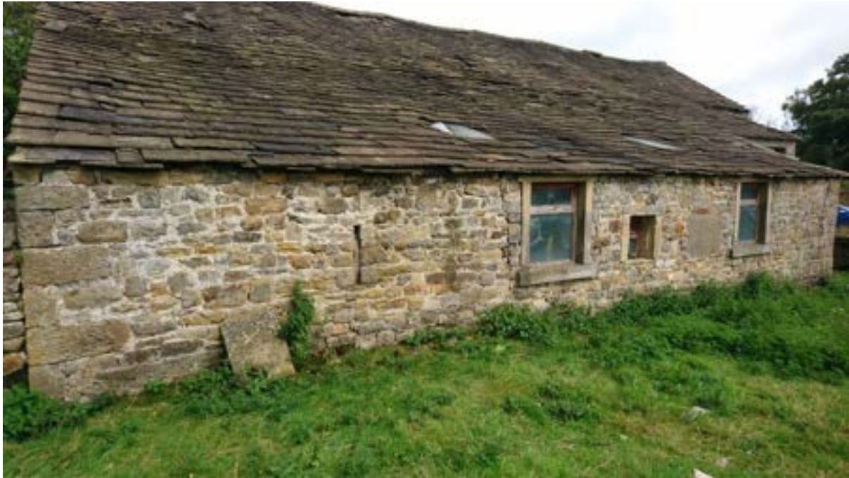
Figure 45: WP7, viewed from the south.
