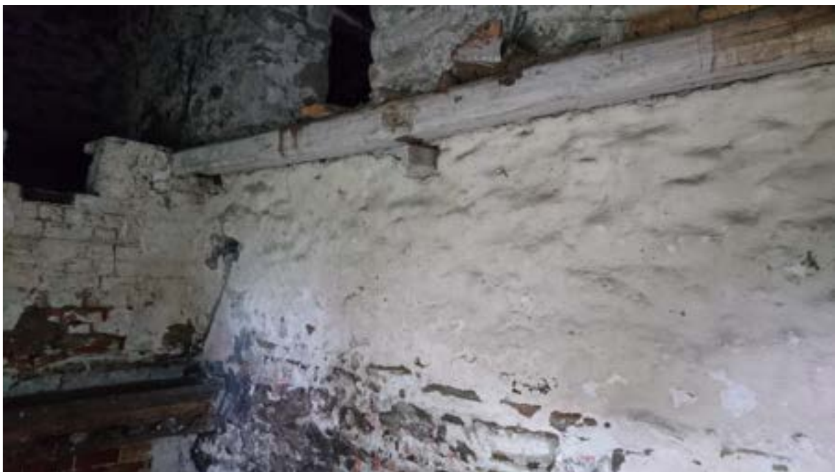
Figure 51: Remains of the first-floor structure over the Stable.
