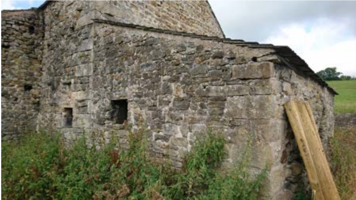
Figure 37: WP 10 - the southern elevation of Extension 1.
