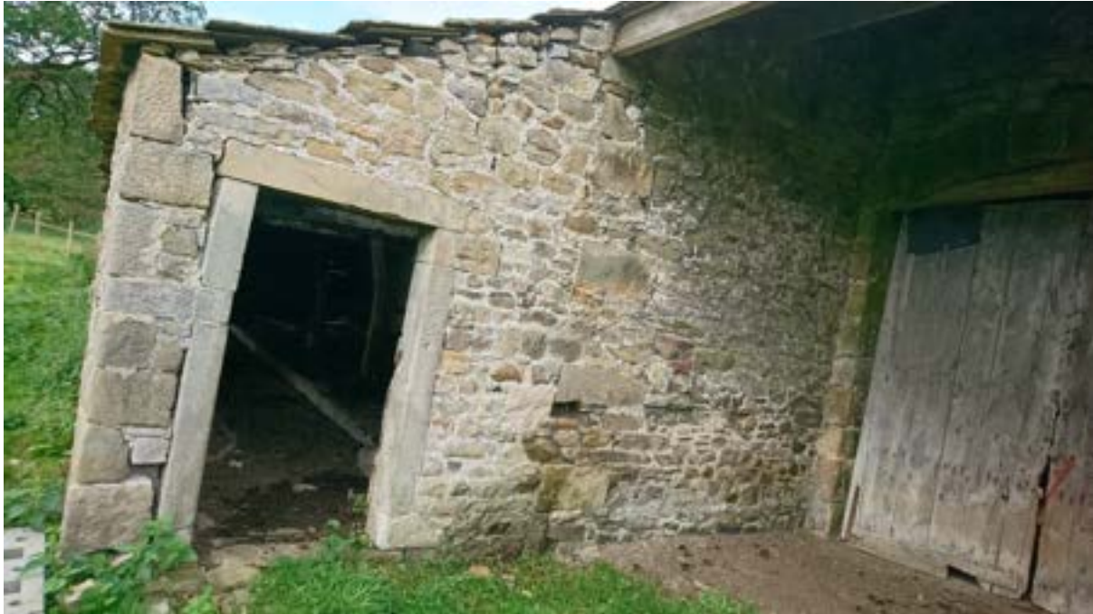
Figure 48: External view of WP8.
