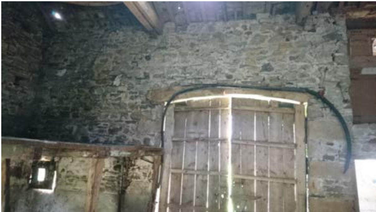
Figure 23: Internal view of WP3 at the eastern end.
