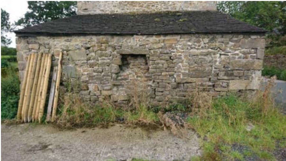
Figure 7: The roof on Extension 1, external view.
