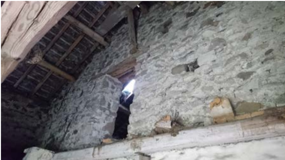
Figure 31: The top of WP4 viewed from the Stable.
