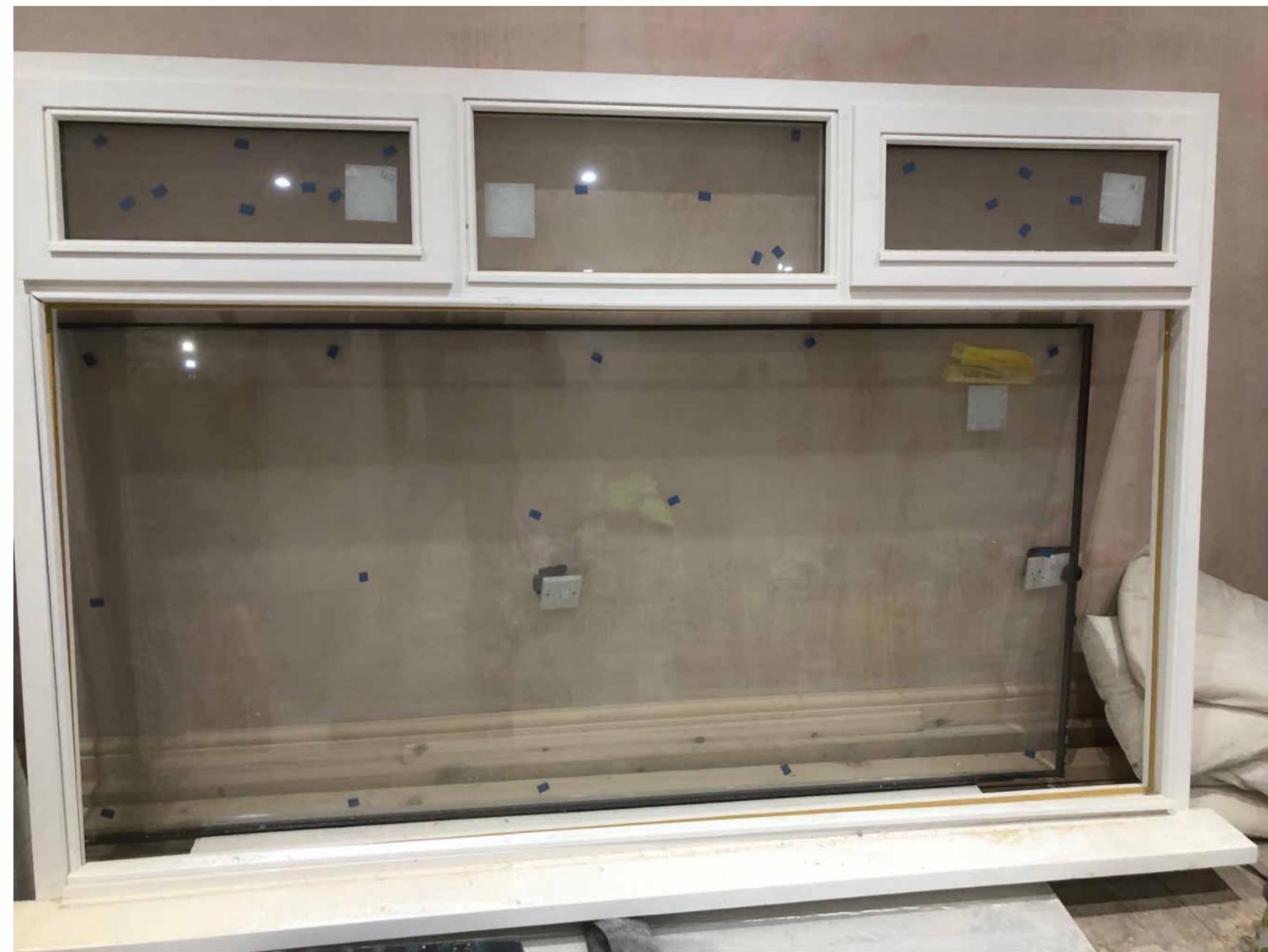
TIMBER CASEMENT WINDOW TO REPLACE EXISTING DAMAGED WINDOW.
