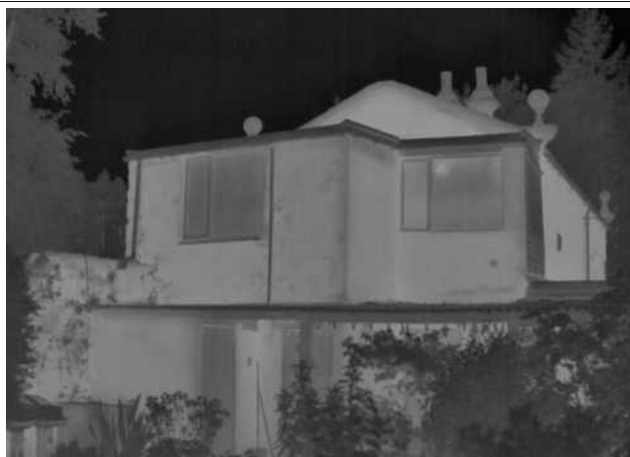
Thermal camera coverage of gable end at end of survey
