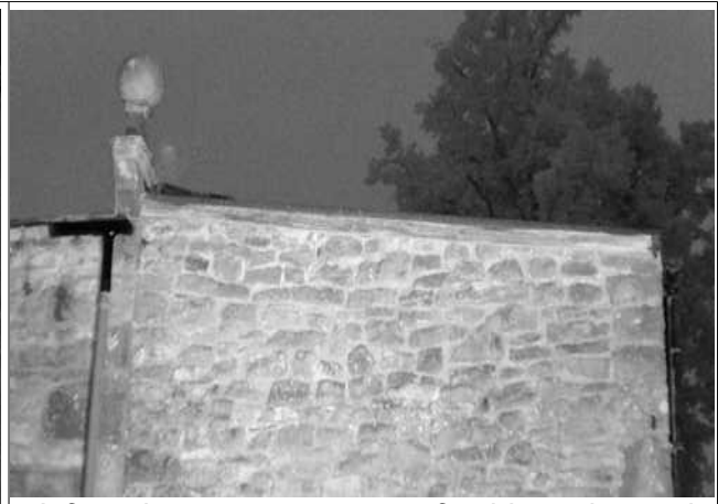
Infrared camera coverage of gable end at end of survey
