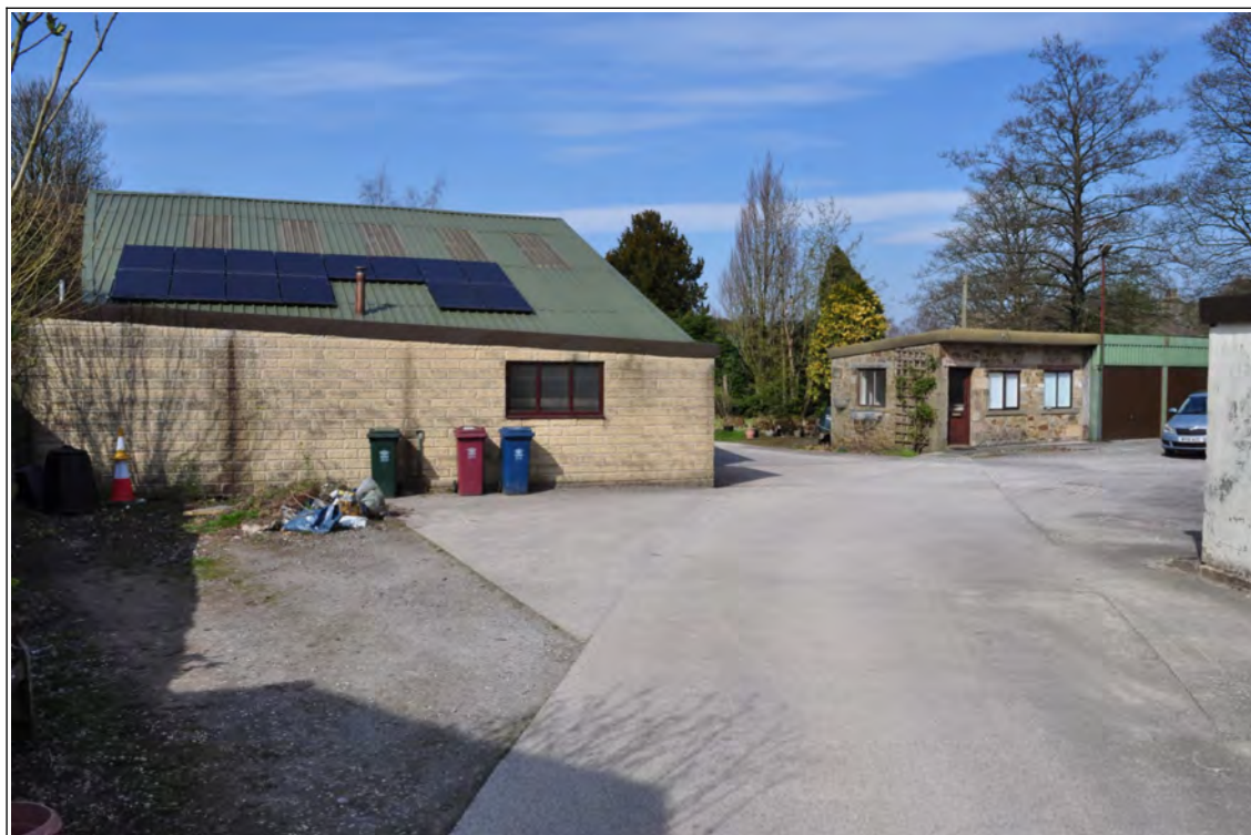
Photo 1: Approach to the site from the south, from Talbot Yard
