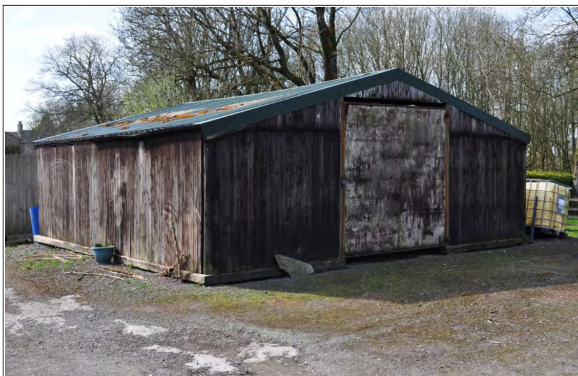
Photo 2: Garage/workshop proposed for demolition
