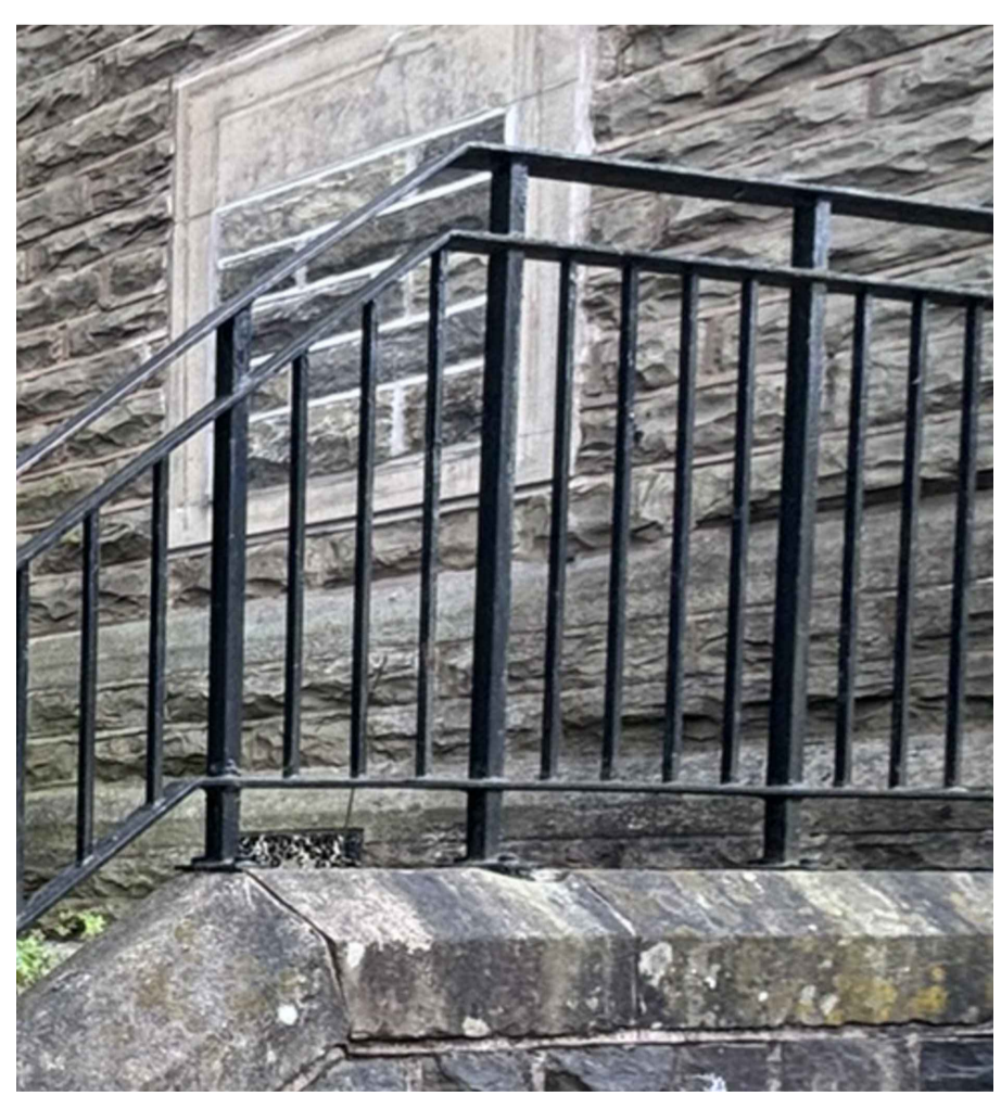
EXAMPLE OF EXISTING METAL RAILINGS
