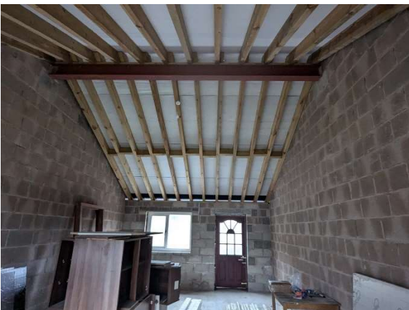
Photograph 14: Internal structure of B2 showing vaulted ceiling with breathable membrane.
