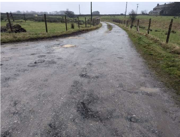
Photograph 3: Existing artificial substrate access road.
