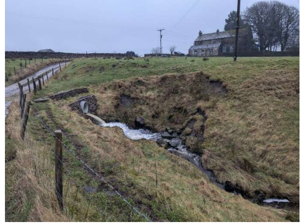
Photograph 4: Brook running through culvert under access track.
