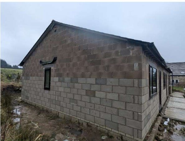
Photograph 13: Northern gable of B2.
