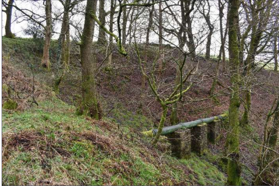
Plate 9: Wooded west side of the application area showing supported pipeline, looking southeast
