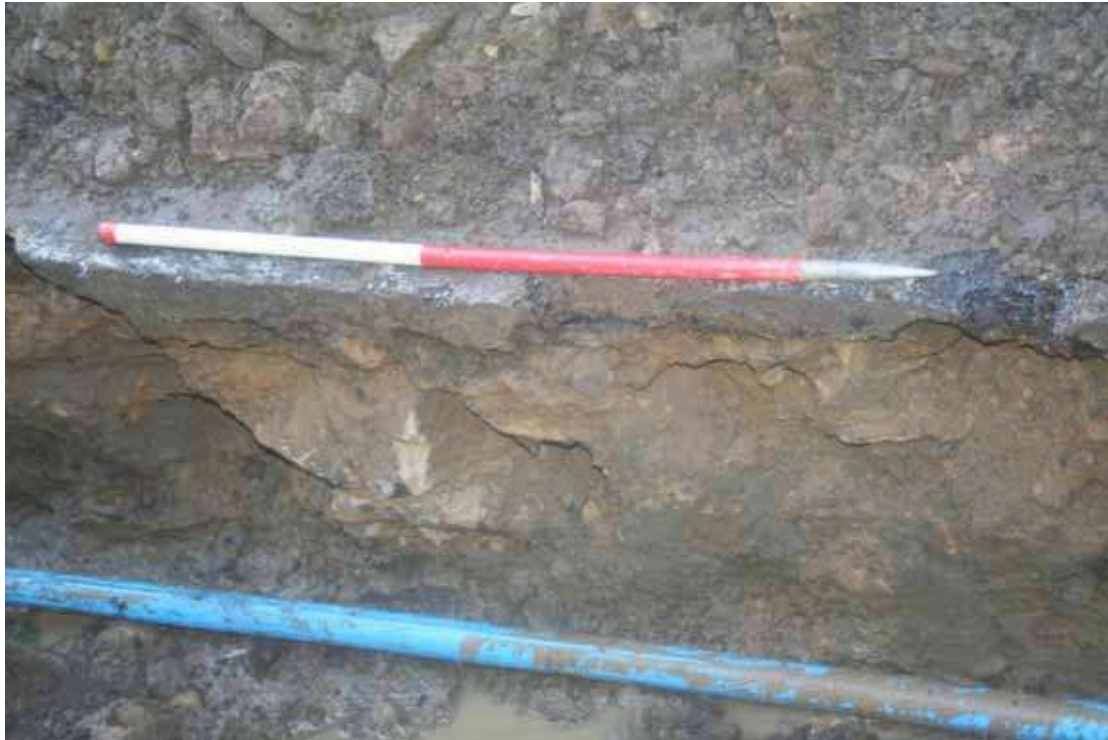
Plate 12: Deposits of large sandstone blocks beneath the surface of Clitheroe Old Road
