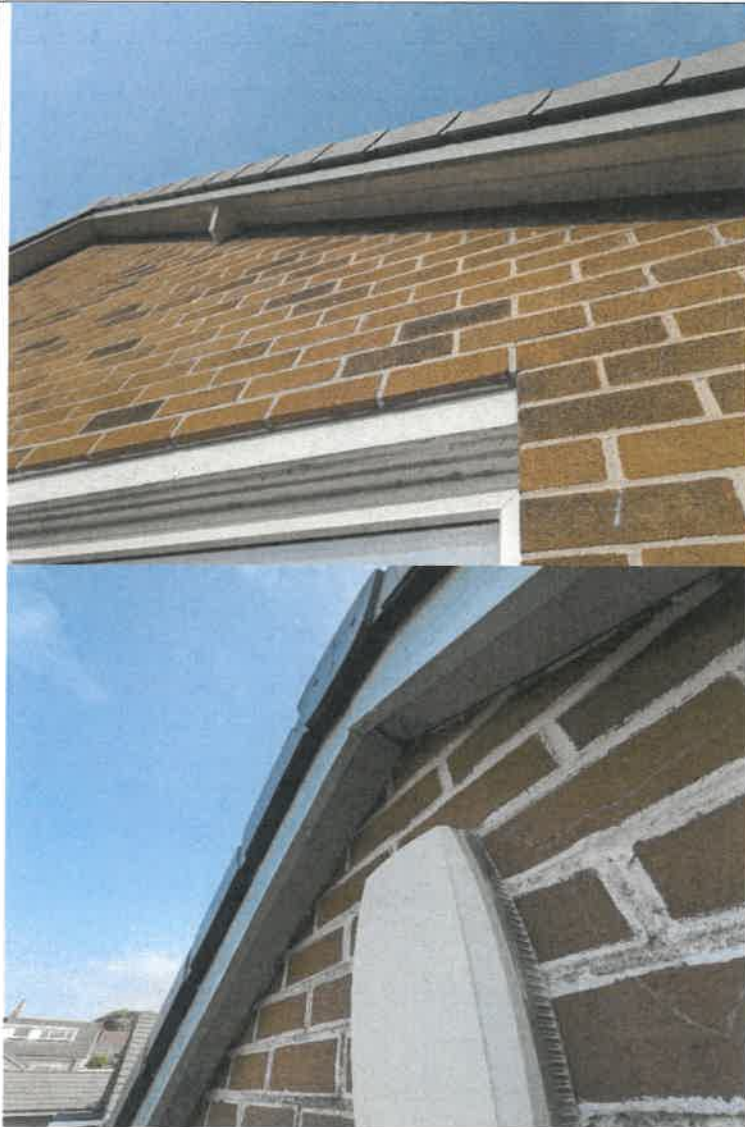
Photos 3 a & 3b. Example of soffits well sealed to the walls.
