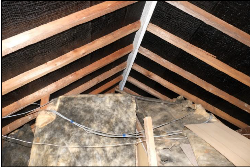
Image of roof void showing deep rock wool and intact bitumastic hessian roof liner.
