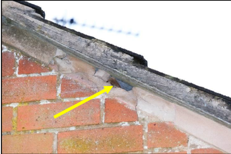
Image showing single cavity on north west gable with some potential for bats to gain access into roof void.
