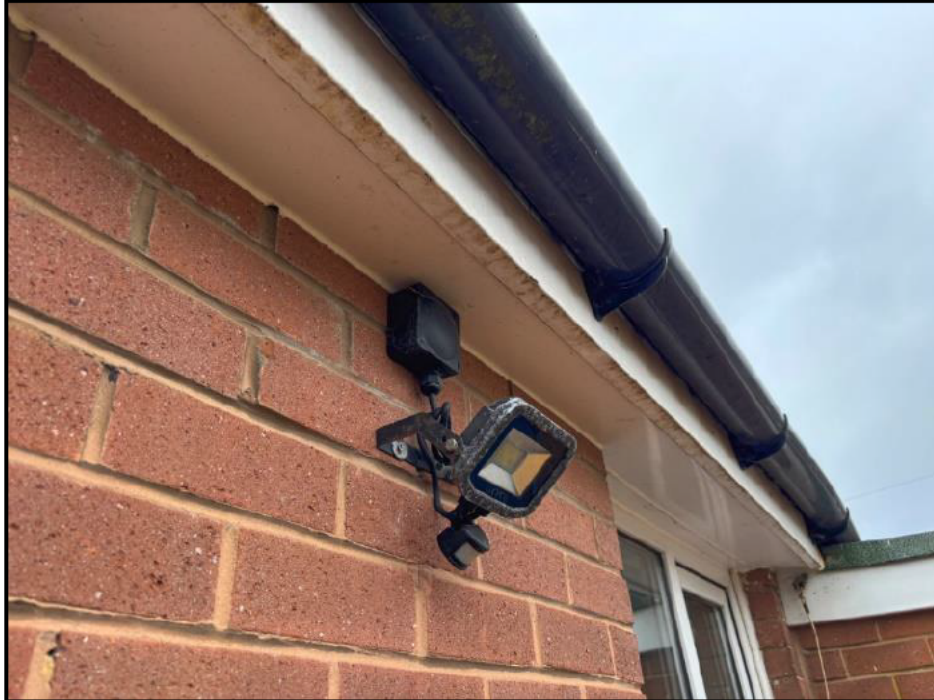
Image showing sealed soffits, no gaps present along roof edges.
