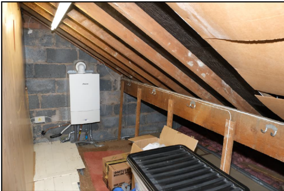
Image of roof void showing boarded floor and internal block walls. This area is currently used for storage.
