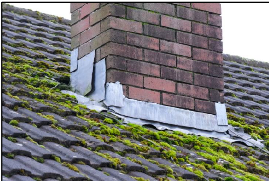
Image showing lead flashing on chimney base with some small gaps and cavities present providing some potential for use by bats.
