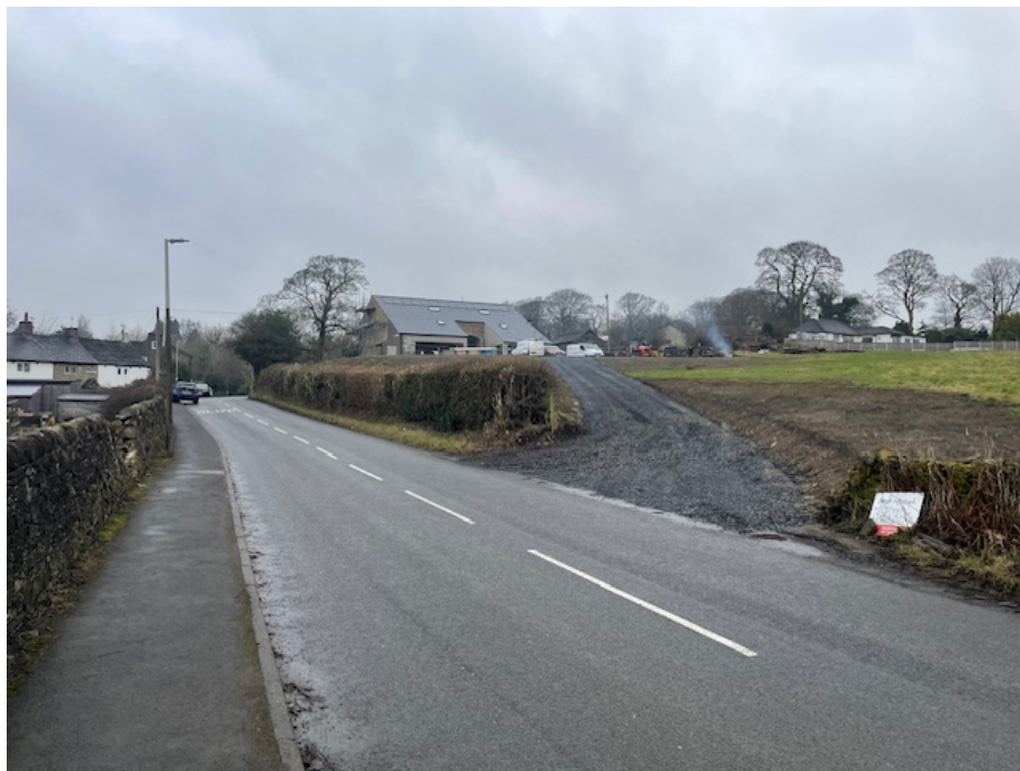
View looking at the entrance on Simonstone Lane
