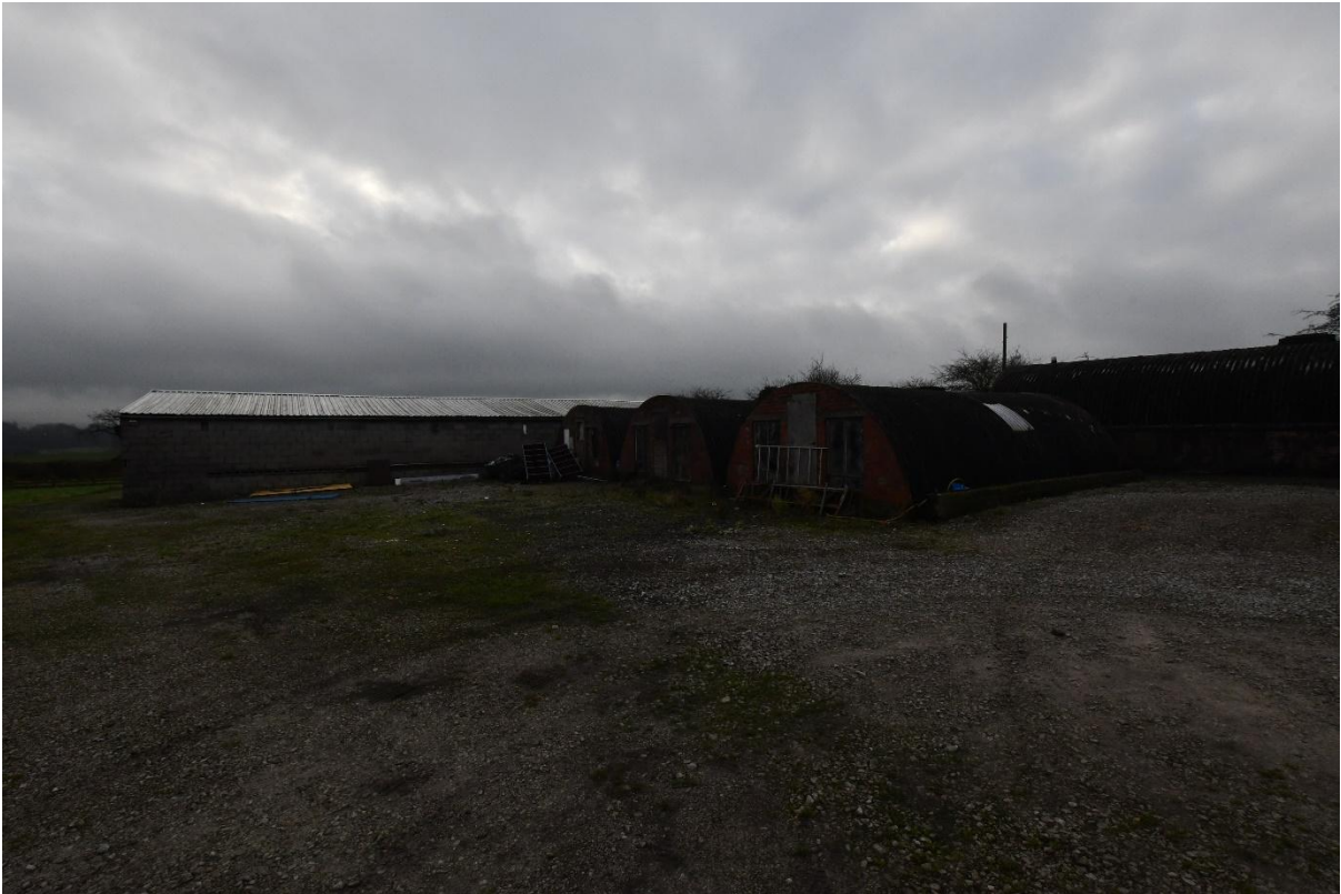
Image 1 South across site to large workshop (target building) and nissen type sheds
