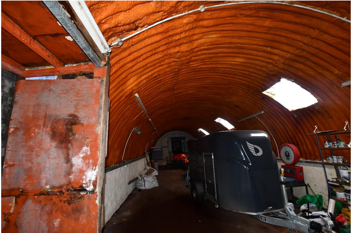
Image 3 Internal structure of Image 2 with ambient light from skylights
