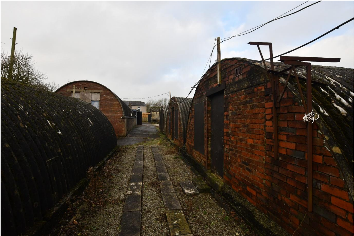
Image 5 Looking north through the various buildings
