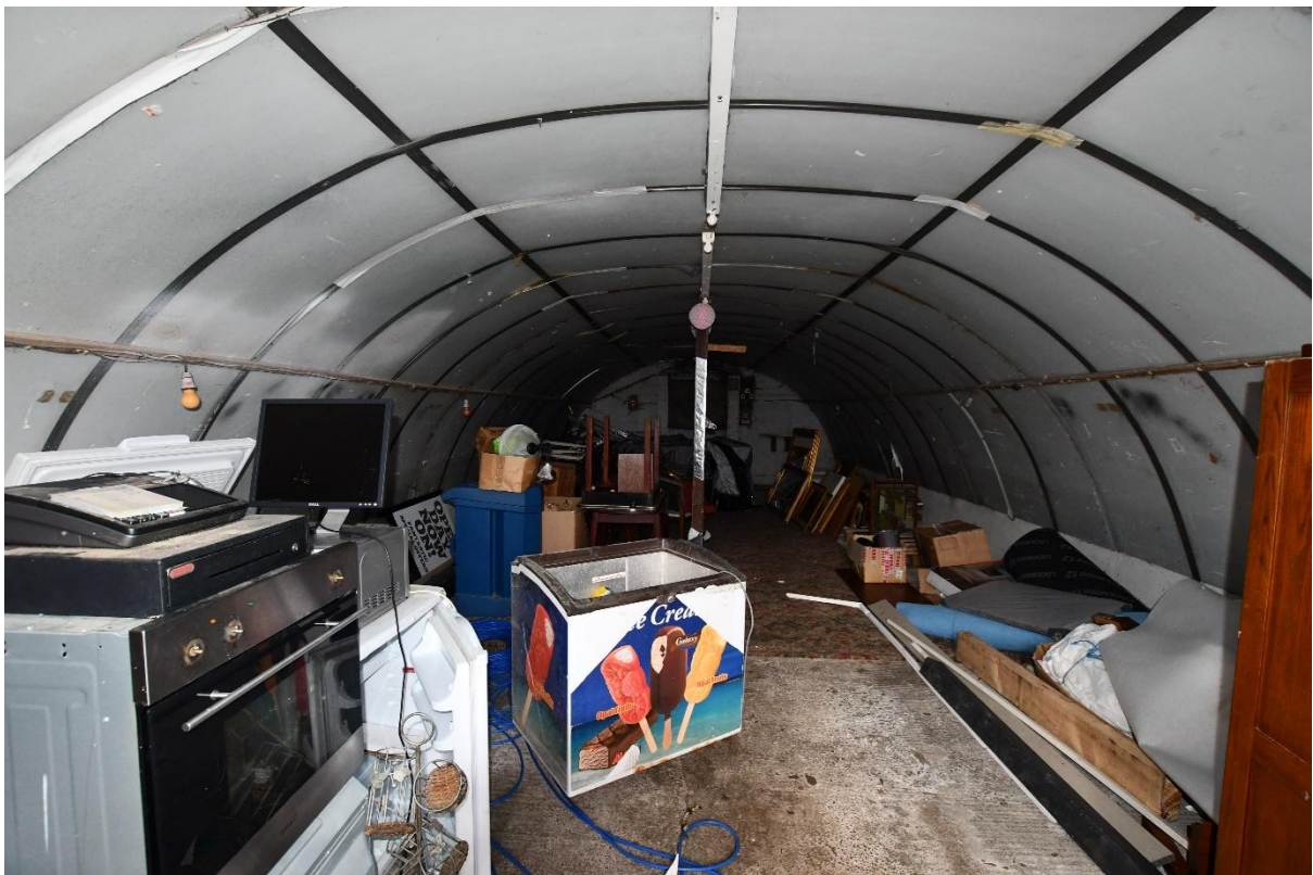
Image 4 Internal structure of large workshop target building
