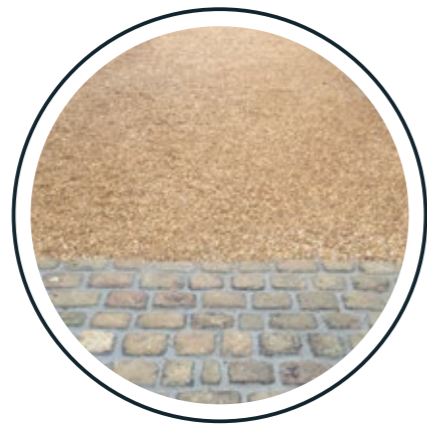
2 Permeable road surface
