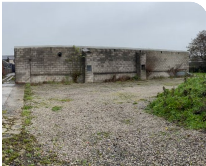
Figure 2.1: Existing south elevation
