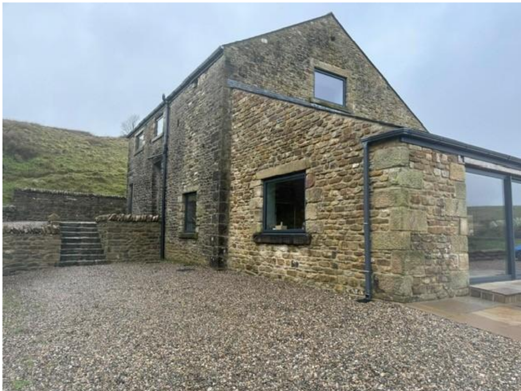
Rear elevation (South) and part of east elevation
