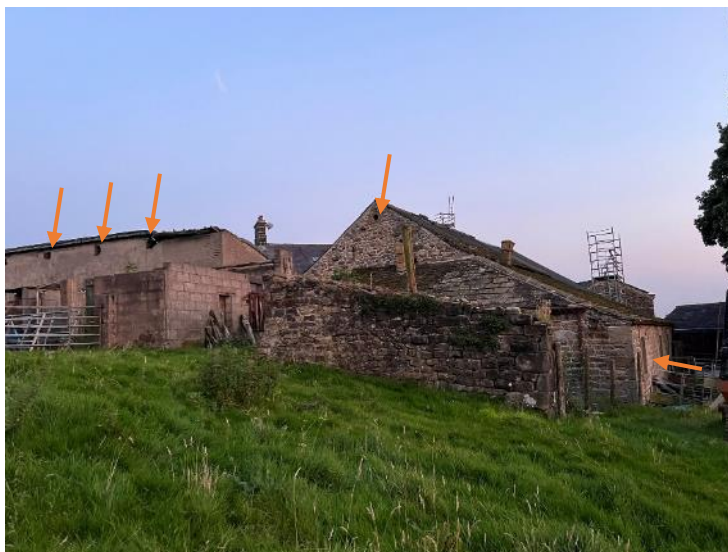
Figure 6: B1 & B3: North elevations with openings marked by arrows.
