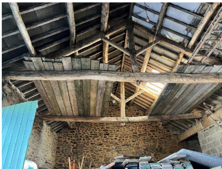
Figure 7: Example of exposed timbers and roof lining of B1.
