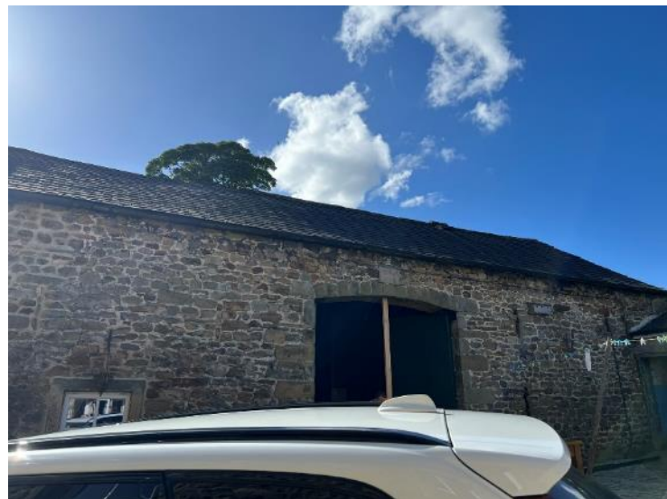
Figure 5: B1 east elevation, main entrance.
