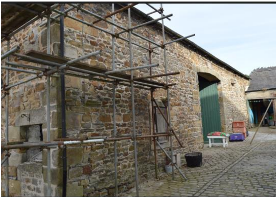
PL01: East facing photo of Green Barn (Front Elevation)
