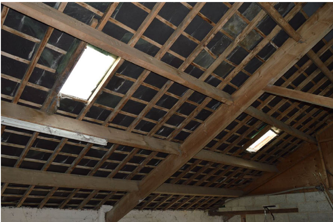
PL19: Photo showing underside of outbuilding 2 roof, comprising of sawn timber half trusses, purlins, rafters battens with natural slate over
