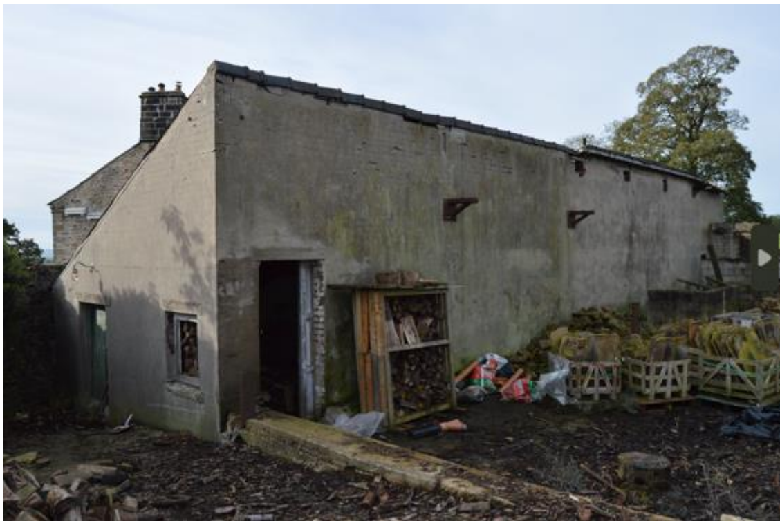
PL09: Outbuilding 2; more recent construction comprising of solid brickwork / blockwork walls rendered with mono pitch roof. To be refurbished and altered for use as proposed garages.
