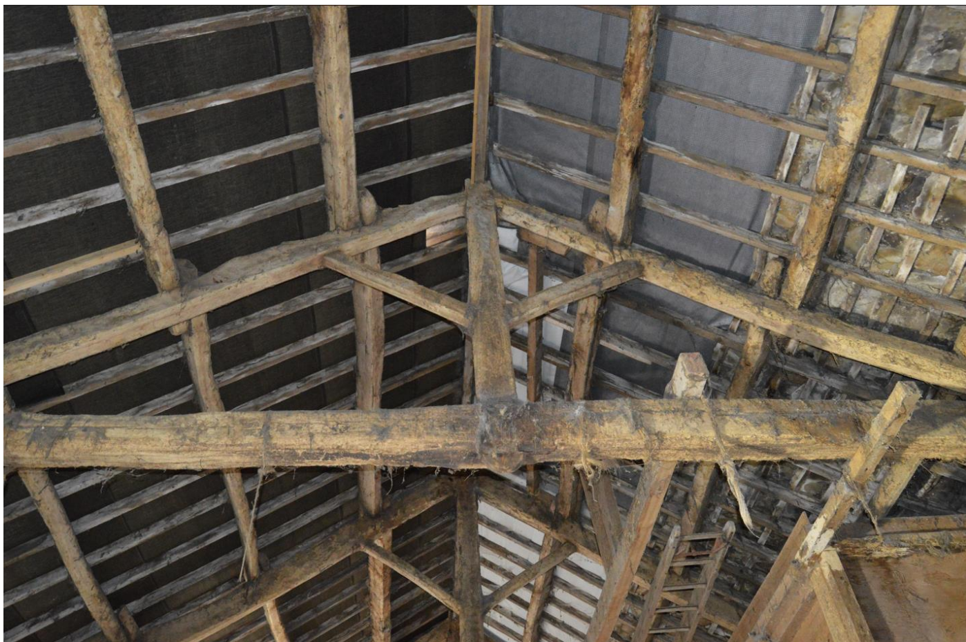
PL14: Photo showing internal roof structure with king post trusses.
