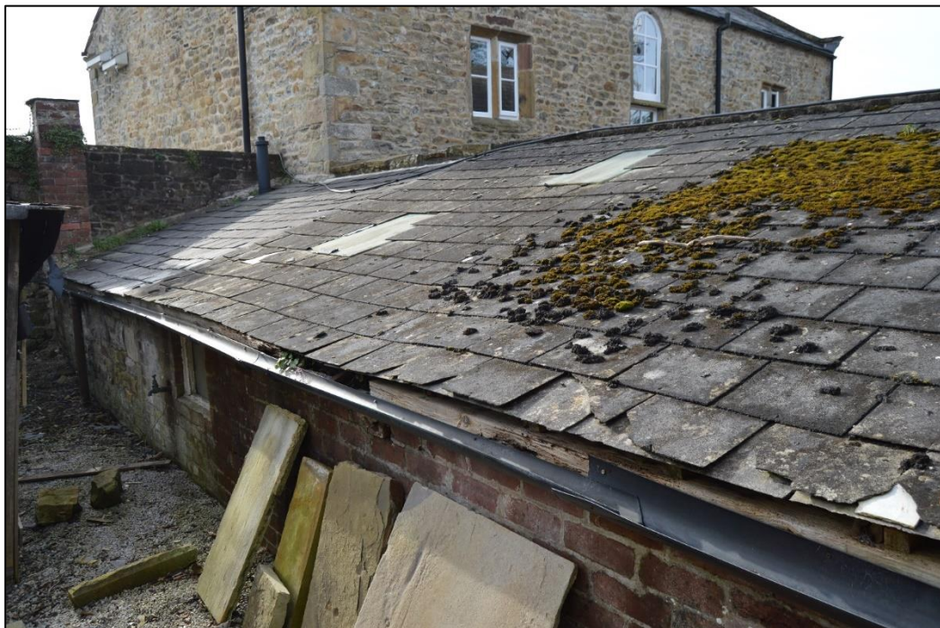
PL18: Photo showing slate/tile roof finish over Outbuilding 1 (which adjoins Eaves House Farm to the rear)
