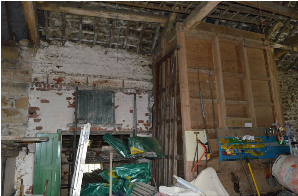
PL21: Original opening built up with brickwork with steel beam over.
