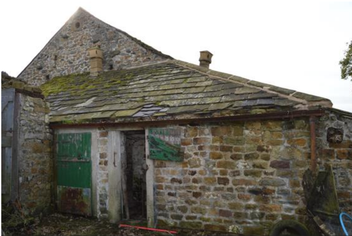
PL02: North facing photo of Green Barn and shippon (Side Elevation)
