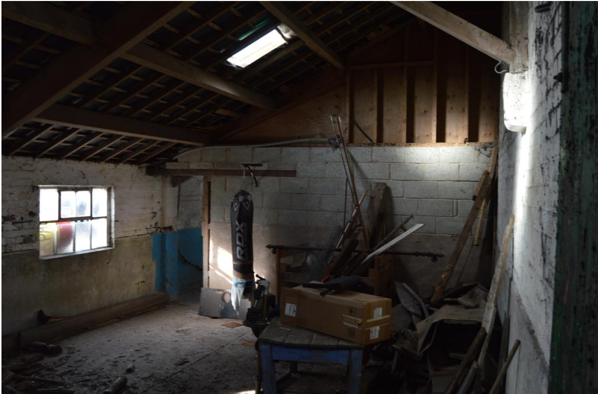
PL10: Outbuilding 2; more recent construction than Green barn, internal photo showing mono pitch rafter and purlin roof with supporting half trusses all in more recent sawn timber than the barn. To be refurbished and altered for use as proposed garages.
