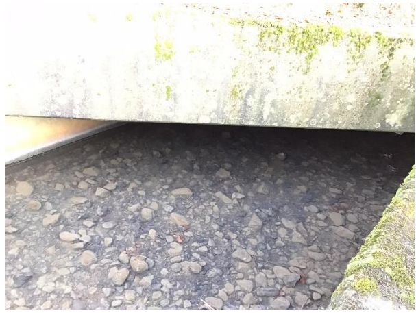
Photograph 4: Coarse Bed Material at Pimlico Link Road Culvert Outlet
