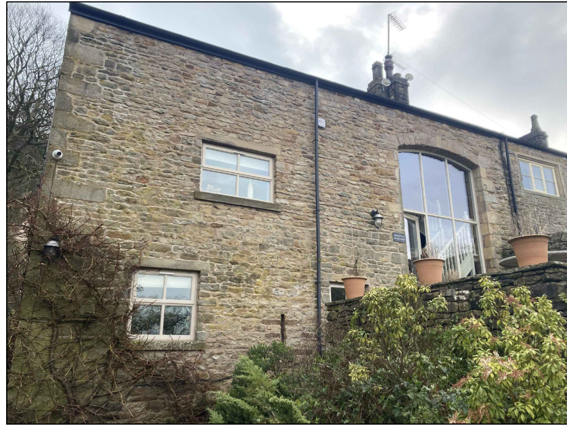
Photograph of North west elevation
