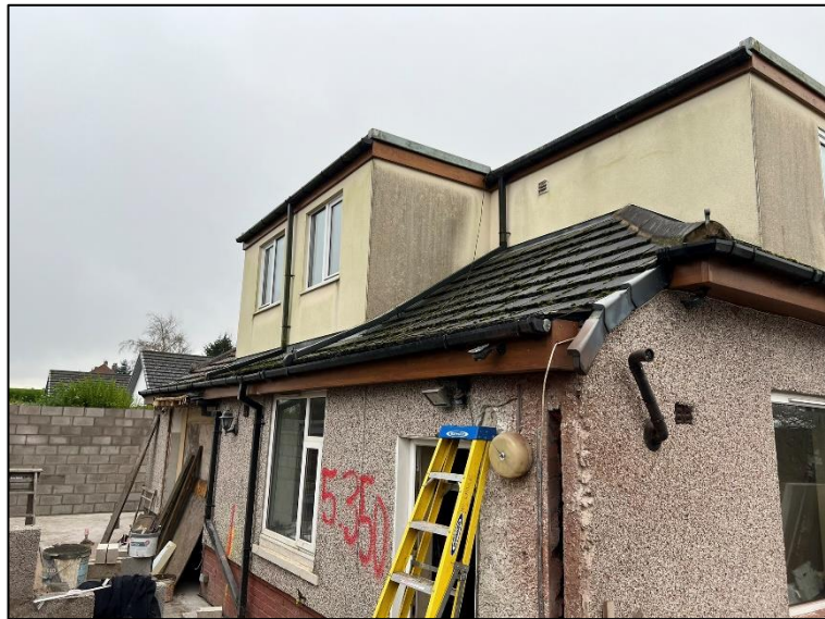
Photo 4: North elevation showing close-up of area where the extension will be constructed. The corner section of the gutter box is shown removed for inspection.
