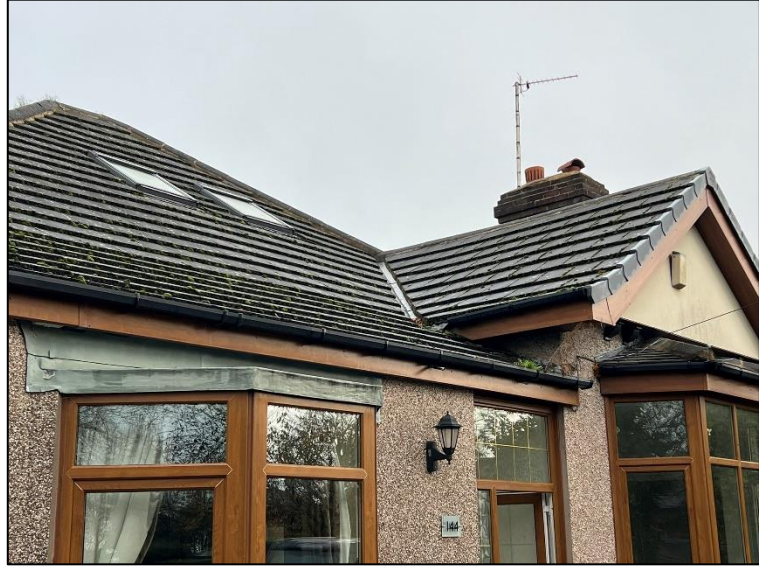
Photo 3: South elevation of the building, showing roof tiles and ridge and roofline materials in good order.
