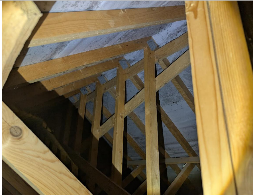
Photo 7 Loft of extension.
