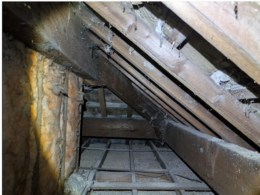
Photo 8 Crawl space around attic (fully accessed).
