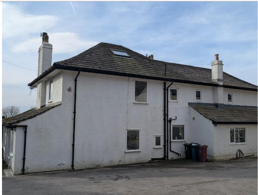
Photo 1 Rear (north) elevation (with converted attic).
