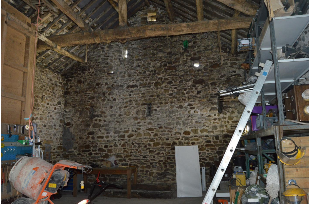
Internal photo of Green Barn
