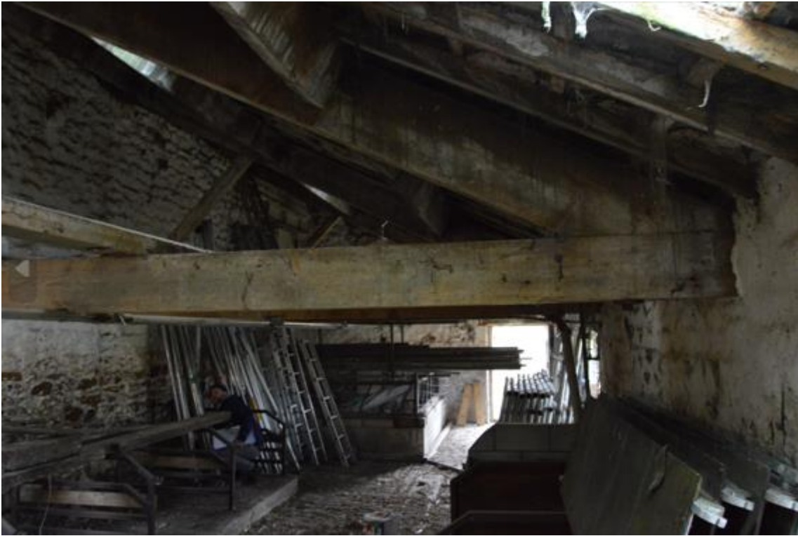
PL08: Internal photo of Green Barn Shippon looking to the south
