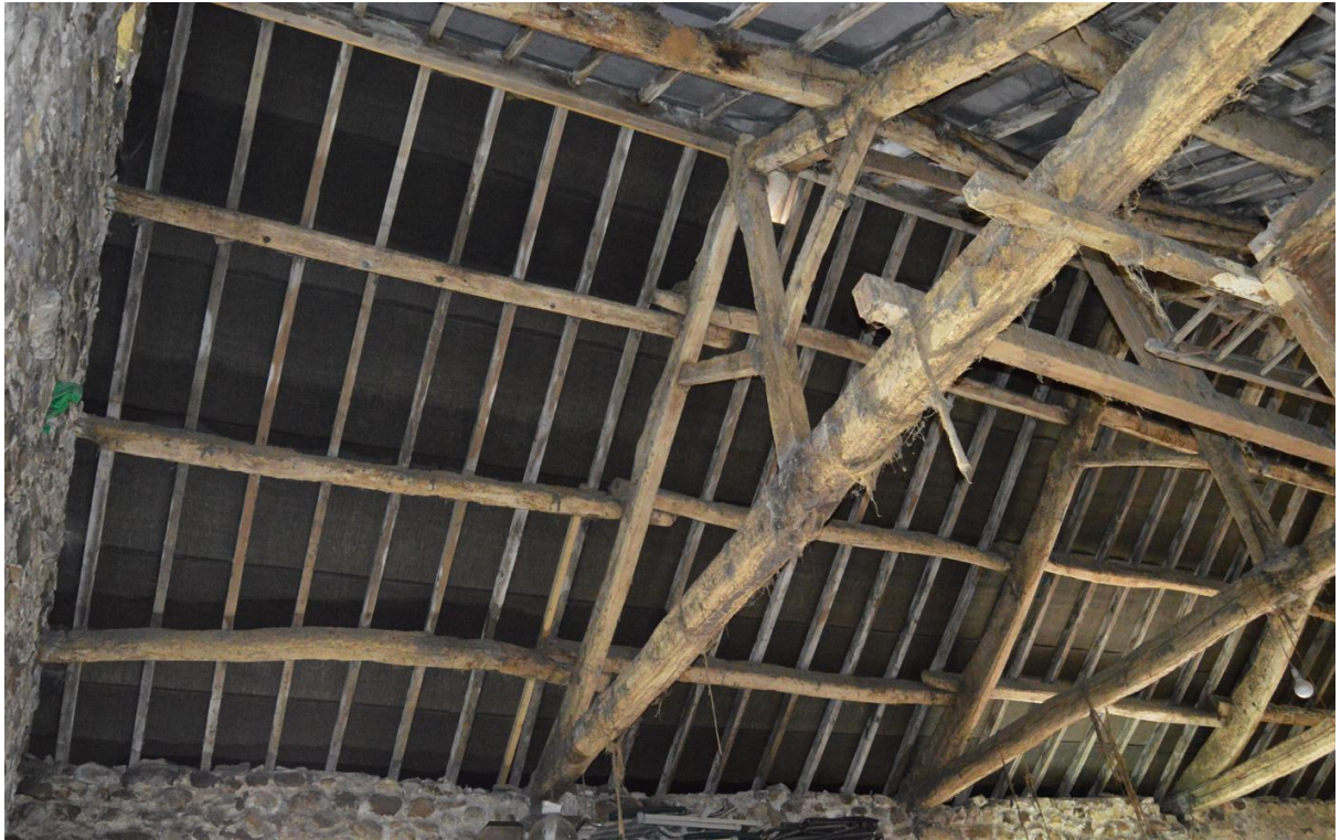
PL15: Photo showing underside of bituminous roofing felt, with battens and blue slate over. Original timber trusses and purlins.
