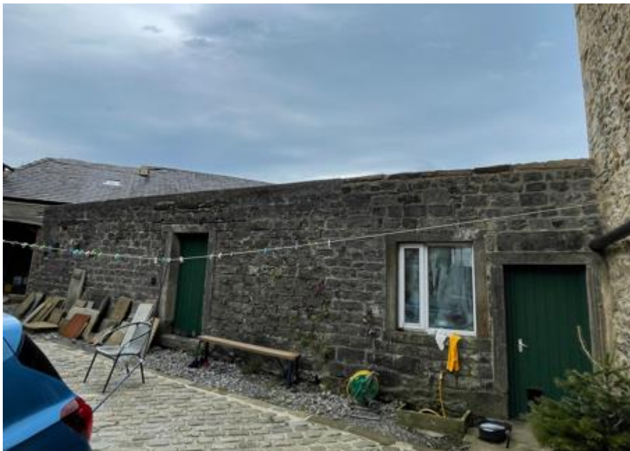
PL11: Outbuilding 1; The right hand side is currently used for plant room, it is proposed to refurbish the end section on the left hand side to use as office accommodation. Structurally the walls are in natural stone and the refurbishment will consist of dry lining internally without disturbing the existing building fabric.
