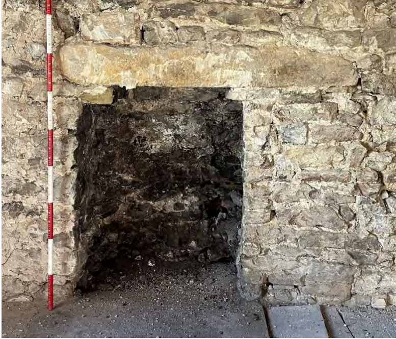
Fireplace detail with heavy stone lintel.
