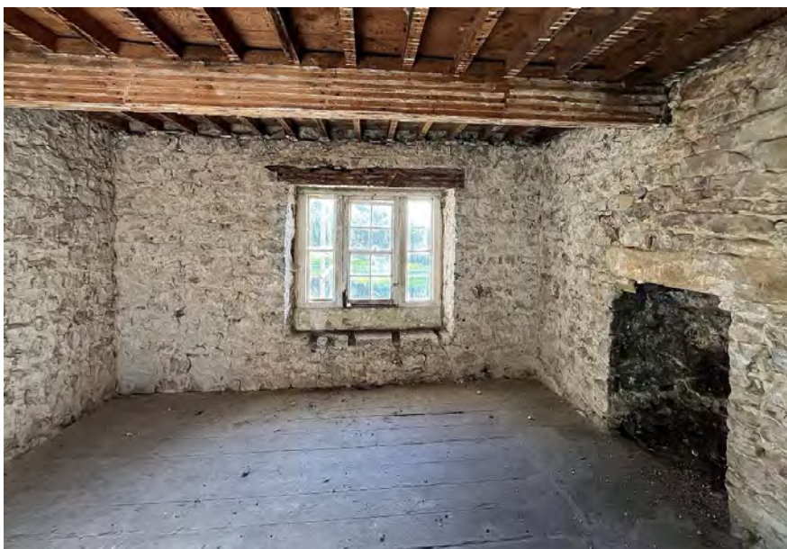
Front room west
