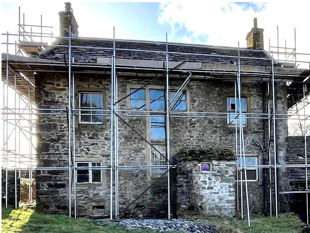
Rear elevation. Fine windows set in random rubble walling
