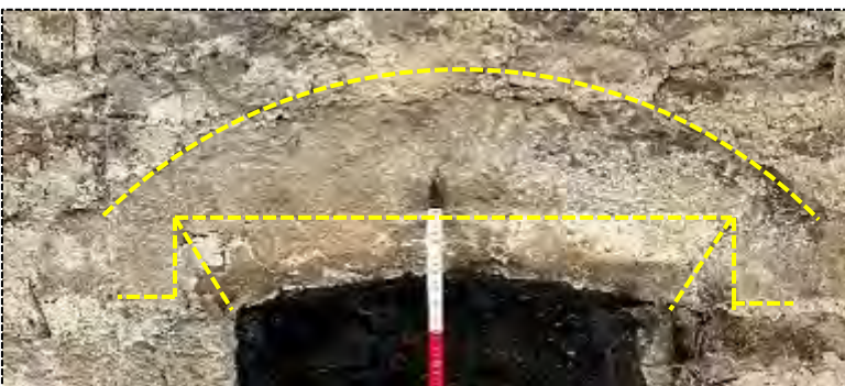
Detail of relieving arch
