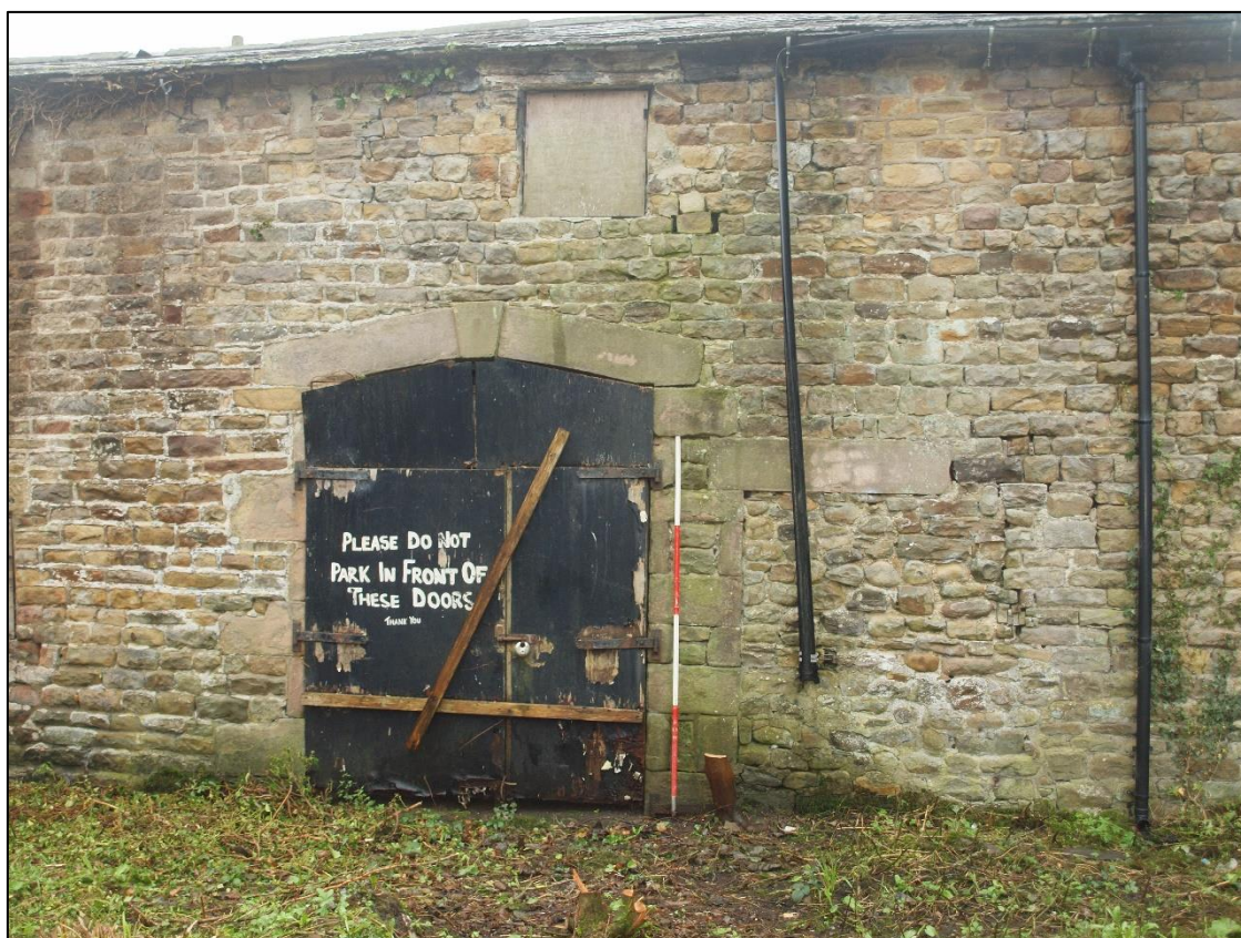
Plate 10: Barn door with cill to be raised
