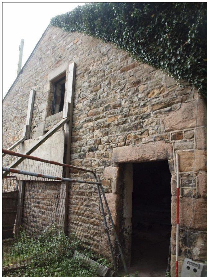
Plate 6: East gable showing doorway to have cill raised
