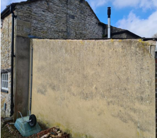
The garage has block/ brick walls with a smooth render finish.
