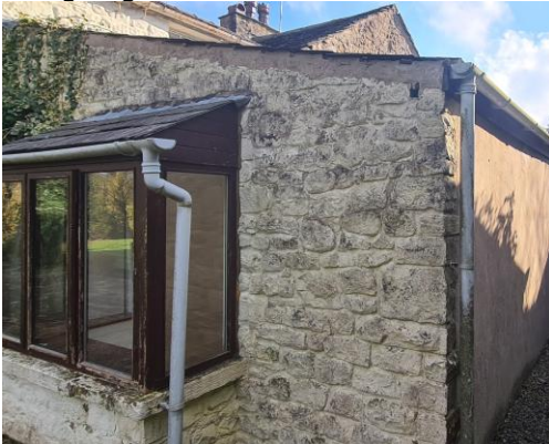
The southwest lean to extension has stone faced side walls and a smooth rendered finish to the southwest elevation.
