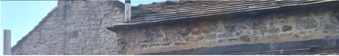
The existing cottage has pointed random solid stone walls
