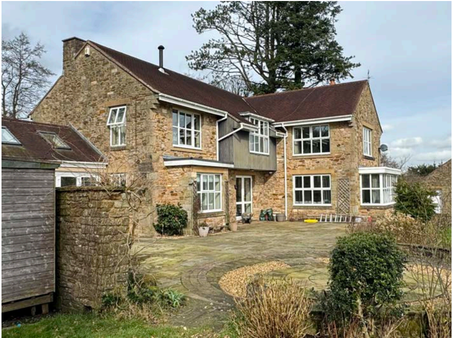
Inelegant 'flying' rear extension with upvc guttering
