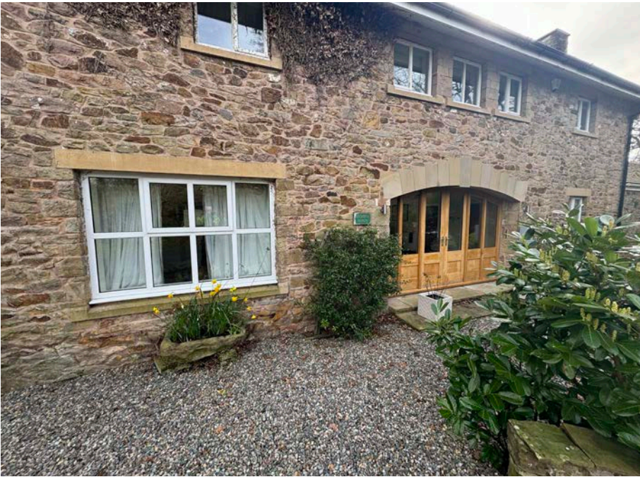
'Fake' stone arch and corbelled roof overhang
