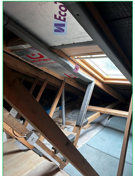
Showing the skylight in the loft space.
