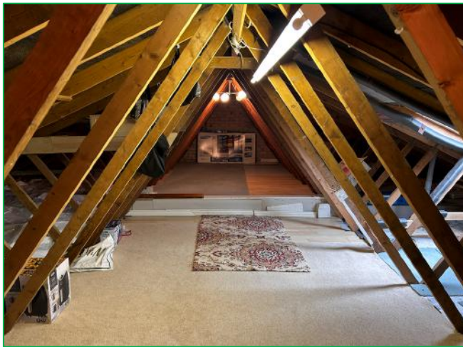
The loft space.
