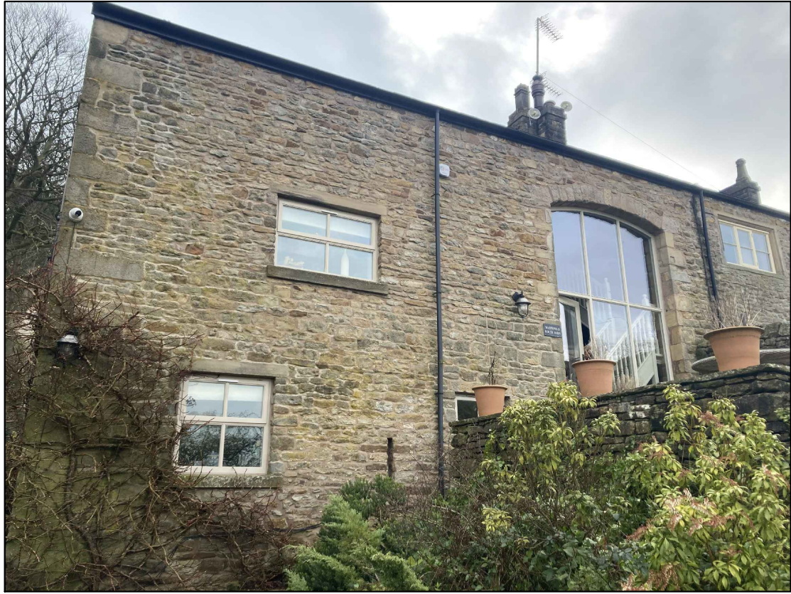
Photograph of North west elevation
