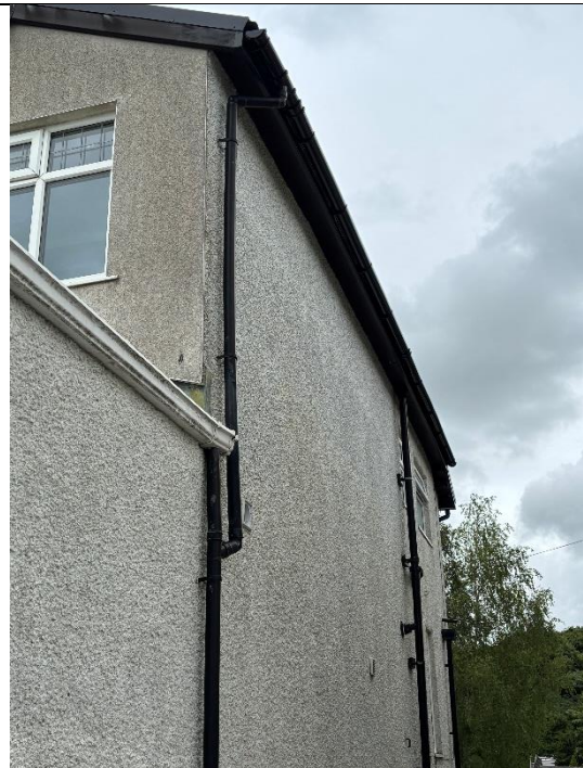
Photograph 4: View of the buildings south facing elevation.
