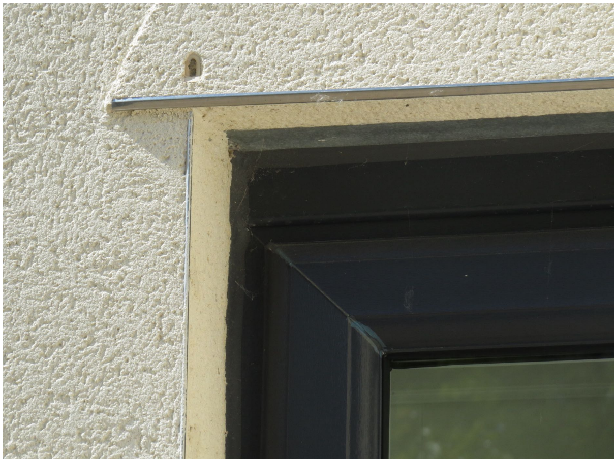
8 – Window and door frames are fitted tightly with no suitable gaps.
