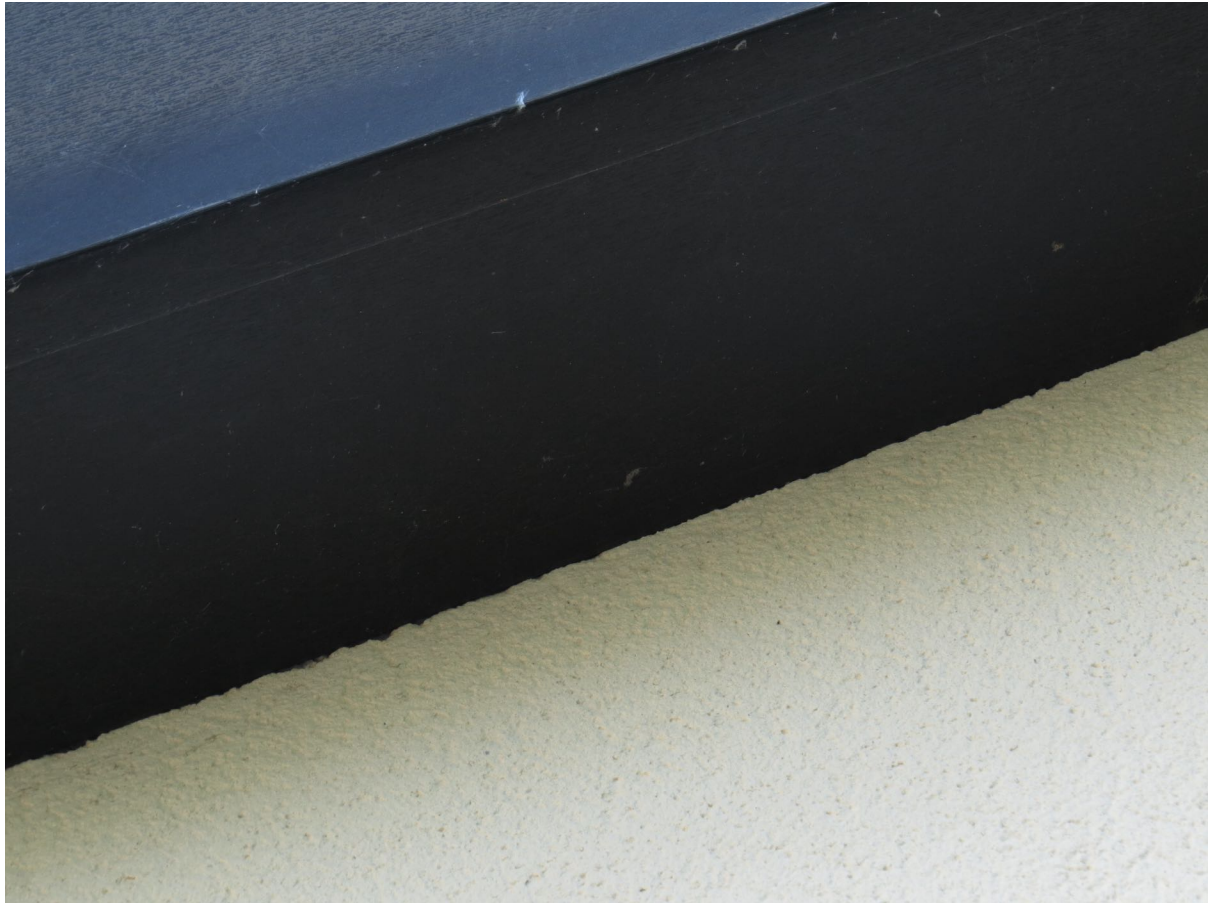
5 – Fascia boards and boxed soffits at the eaves are fixed tightly against brickwork.
