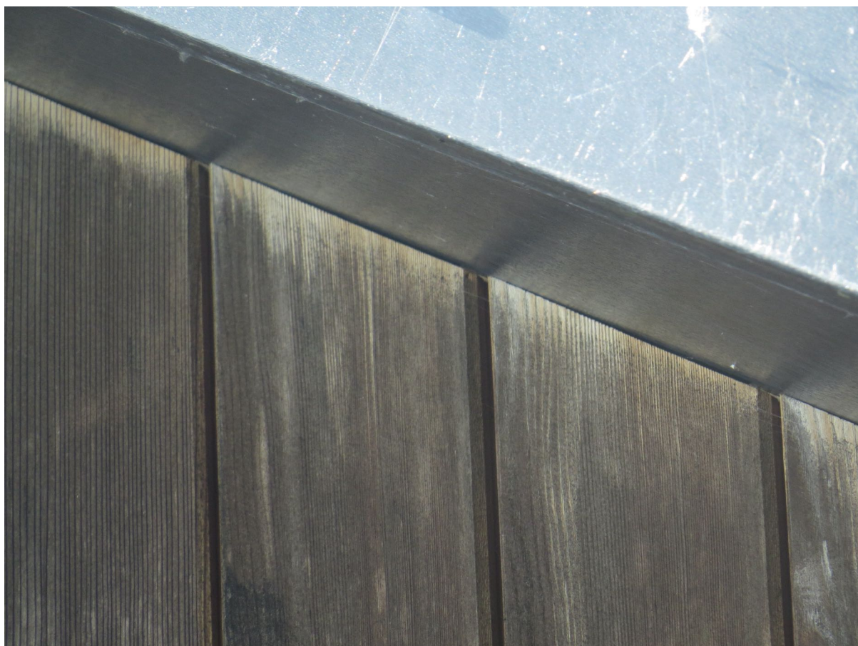
9 – Timber cladding is fitted tightly with no warped boards or gaps between materials.
