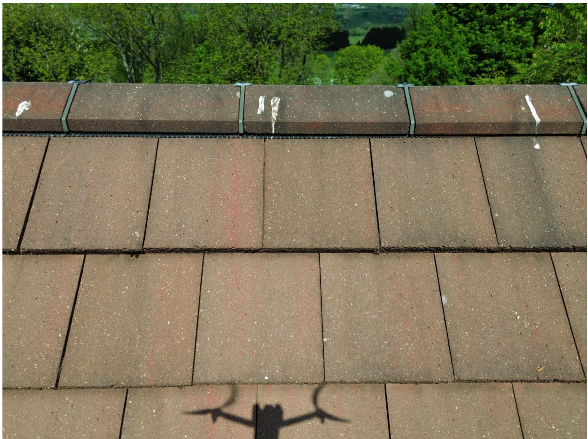
4 – Ridge tiles are mechanically fixed, roof tiles are in good condition.
