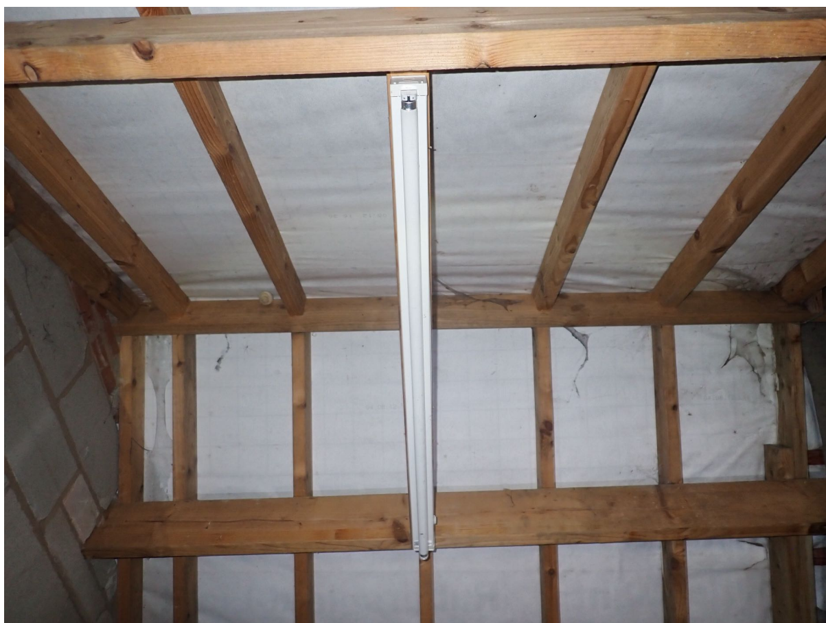
10 – The garage roof is lined with a modern breathable membrane.
