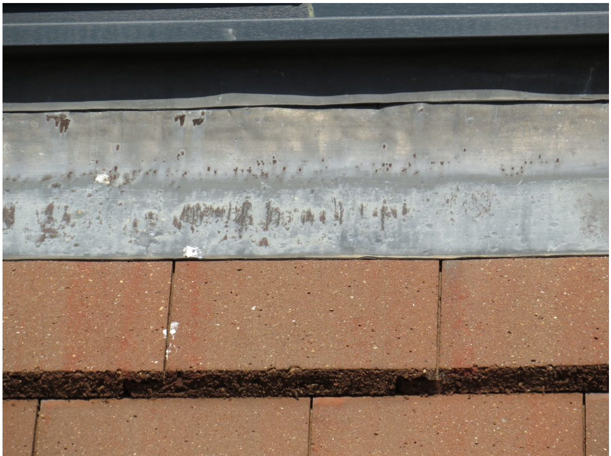
6 – Leadwork is fixed tightly with no viable gaps.
