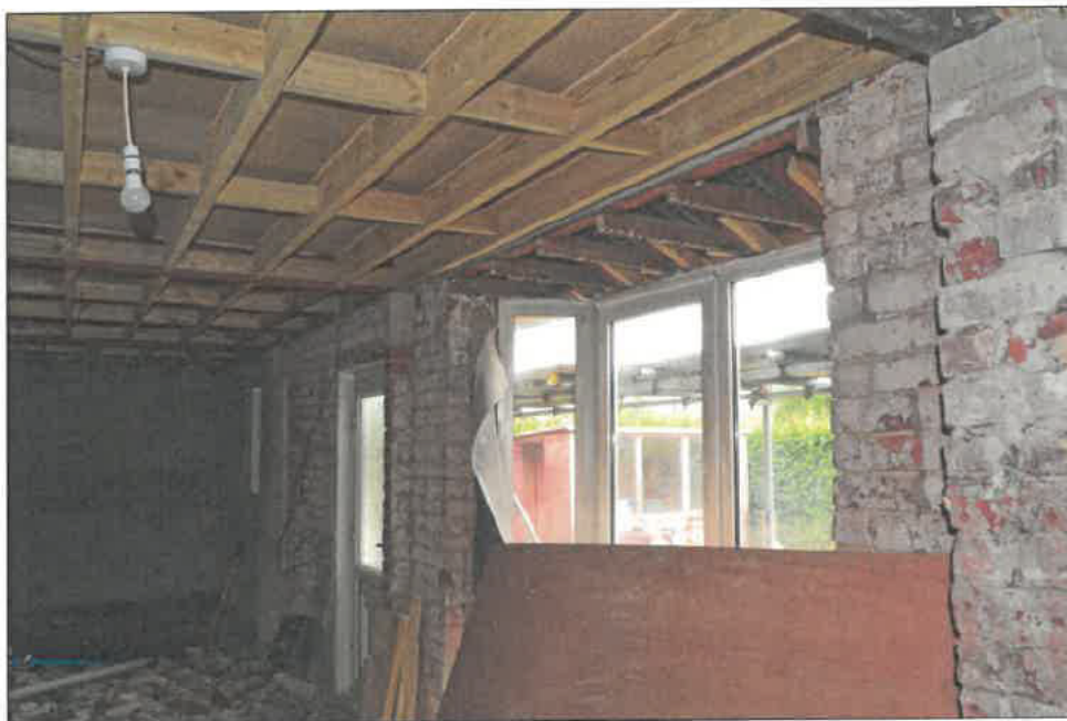
Internal view of 86 Whalley Road. At the time of survey, the building was undergoing extensive refurbishment, which included stripping of walls and installing of new floors.
