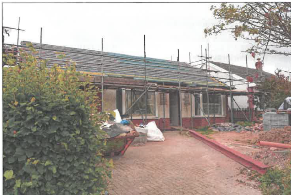
View of 86 Whalley Road from roadside to northwest. At the time of survey, the building was scaffolded and the northwest roof pitch was covered in a modern roof membrane and tile battens only.
