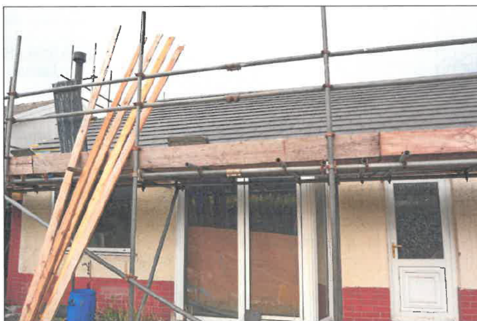
View of 86 Whalley Road from garden to southeast. At the time of survey, this part of the building was scaffolded, and the southeast roof pitch was newly-covered in interlocking cement roof tiles.
