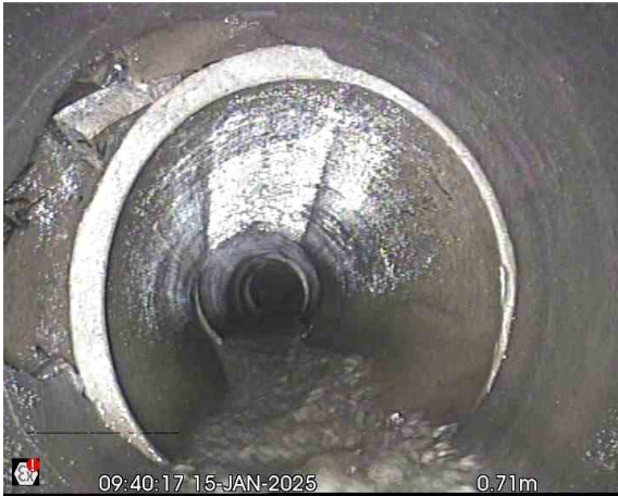
Branch BX_4dce1fac-847e-46a0-8b54-6a38226a0431_20250120_13 4445_963.jpg, 00:00:13, 0.71 m Hole in drain or sewer from 7 o'clock to 12 o'clock
