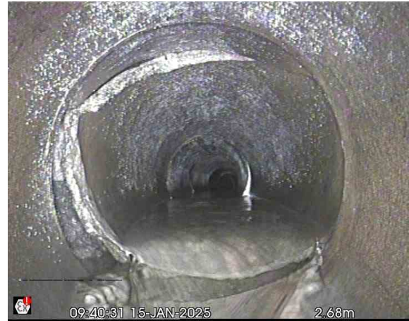
Branch BX_191e6468-be29-4b7d-ad17-b3a19b03bf7d_20250120_13 4506_450.jpg, 00:00:26, 2.68 m Broken pipe at joint from 12 o'clock to 12 o'clock
