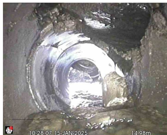
10:28:07 15-JAN-2025 14.98m Gully 6X_0b17438e-793e-4b31-8b67-90dc28e43b84_20250120_13 4913_730.jpg, 00:00:57, 14.98 m Hole in drain or sewer from 10 o'clock to 03 o'clock
