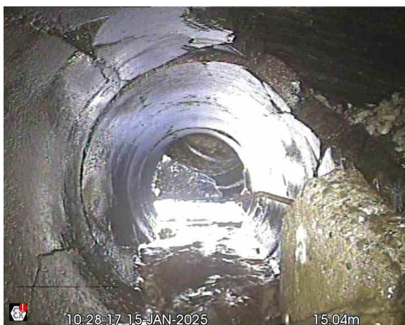
10:28:17 15-JAN-2025 15.04m Gully 6X_c4e54004-587e-41ca-ab3c-9ca7126bb01a_20250120_13 4949_800.jpg, 00:01:07, 15.04 m Other obstacles, other object in invert from 03 o'clock to 6 o'clock, 15% cross-sectional area loss, stone fallen from hole
