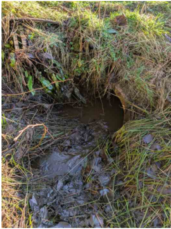
Outfall flowing better after jetting
