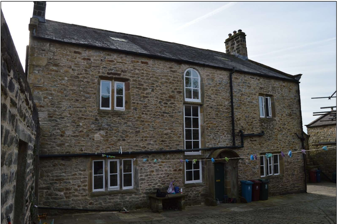
PL04: View of the rear north facing elevation of Eaves House Farmhouse.
