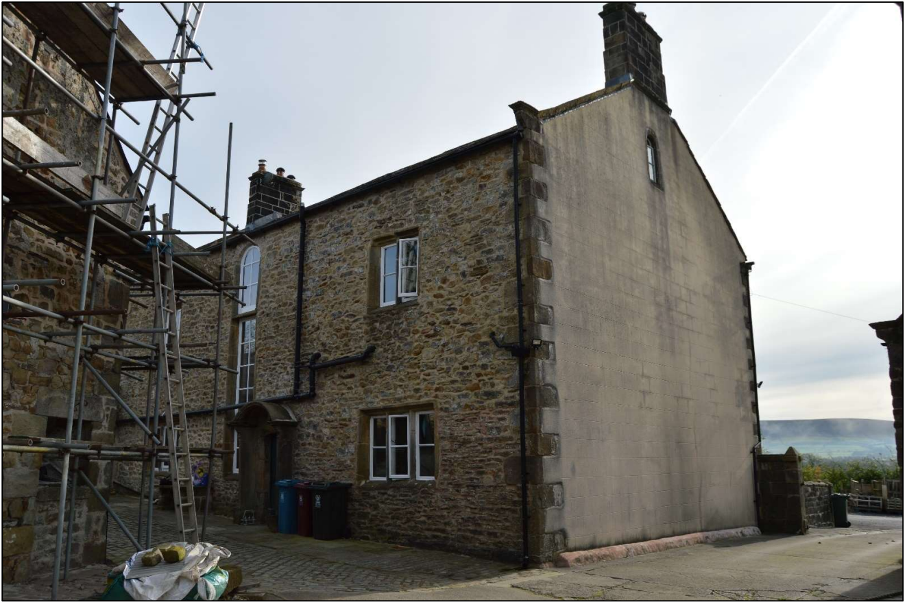
PL03: View of Eaves House farmhouse from the north west.
