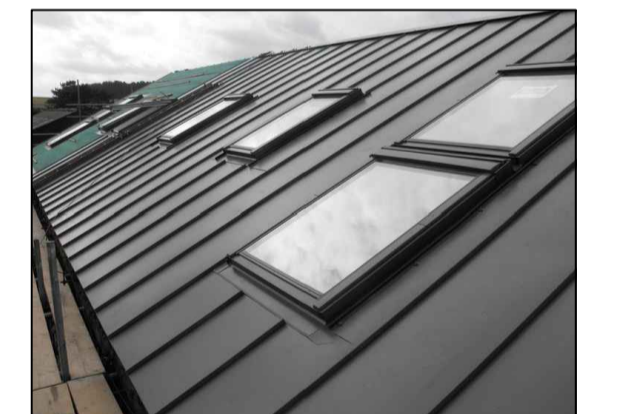
Example of Proposed Fakro GB FPW-V/C P2 Conservation Low Profile Roof Lights
