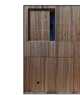
Louvered timber cladding over windows
