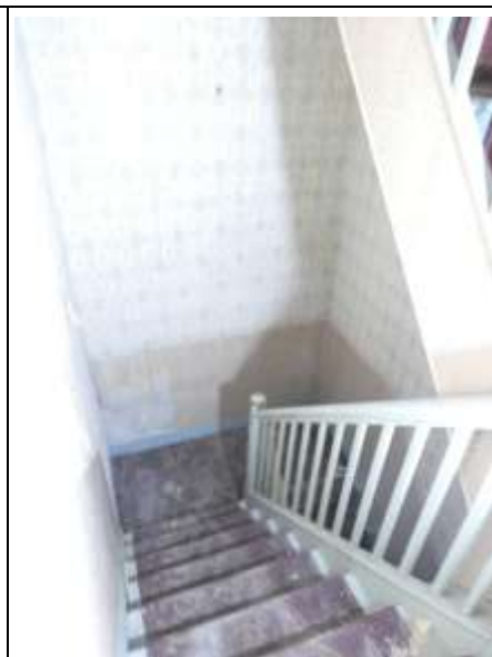
Looking From First Floor
