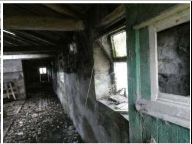
Timber Framed Windows
