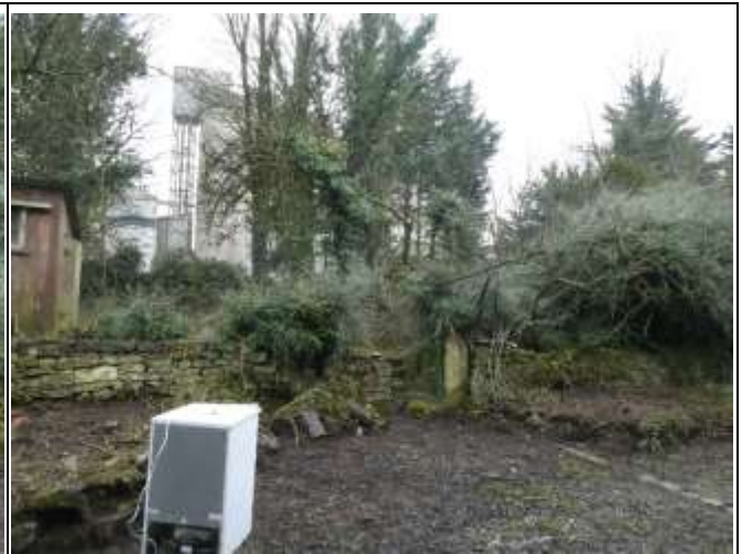
Stone Walling and Remaining Stone Pier
