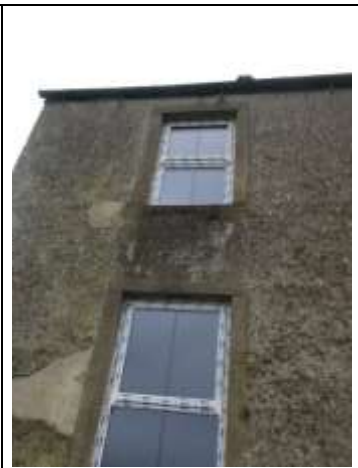
First Floor Window, West End of Elevation
