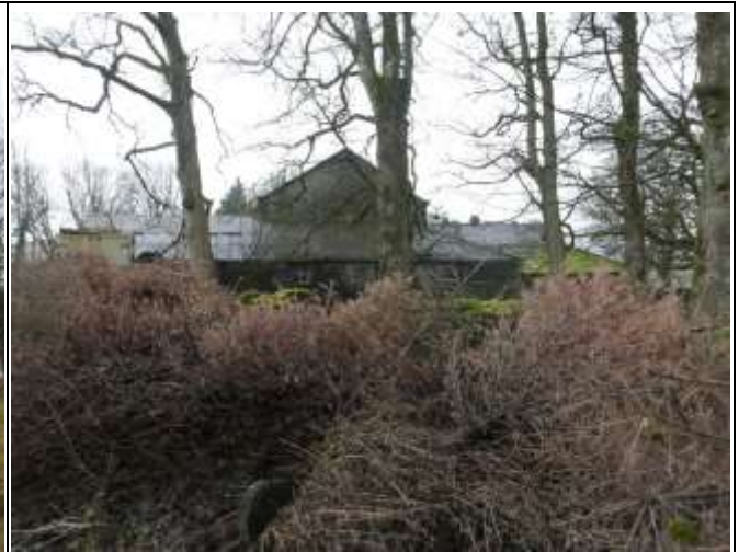
Looking North Towards Outshut and Outbuilding
