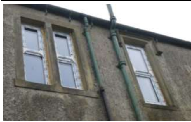
First Floor Windows at the Centre of the Elevation
