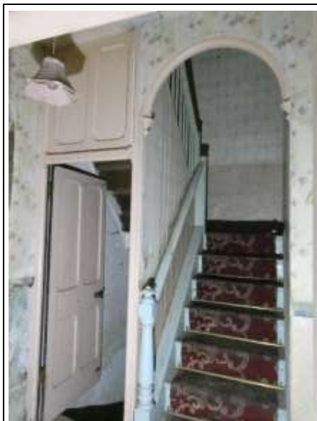
Archway Architrave and Timber Door at Basement Stairs
