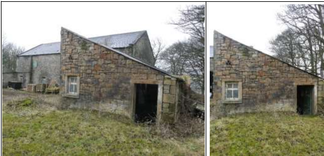
South Elevation, Single Storey Outshut
