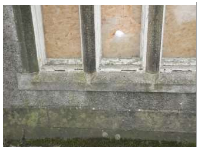
Dressed Stone Window Surround and Plinth
