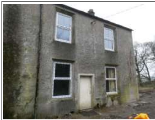
East Side of Elevation with Entrance
