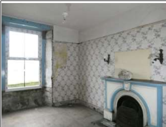
Replacement Window at the North Elevation
