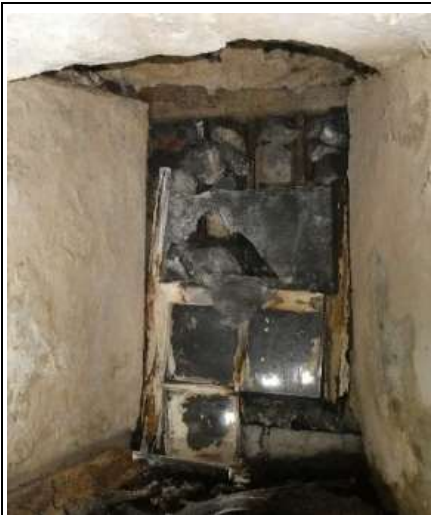
Small Blocked-up Opening at the East Elevation
