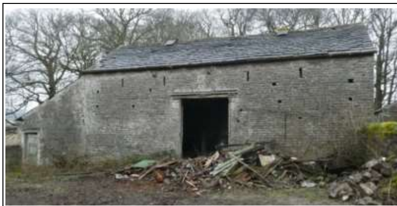
West Elevation, Ventilation Slits and a Tall Cart Entry
