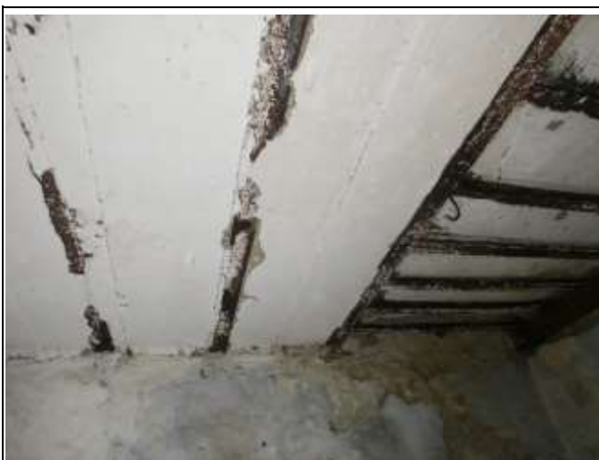
Ironwork at the Ceiling, with an Iron Hook in Situ
