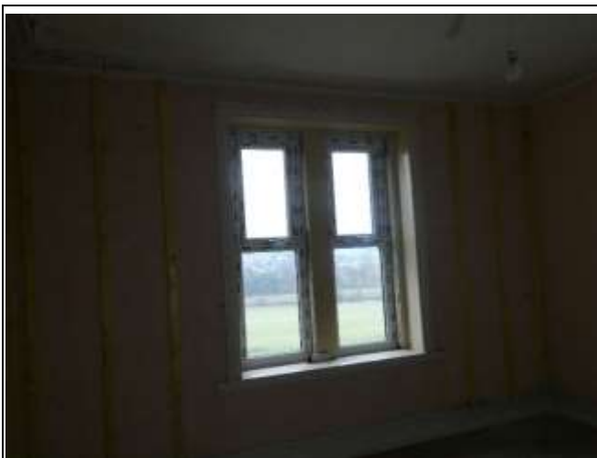
Replacement Window to the North
