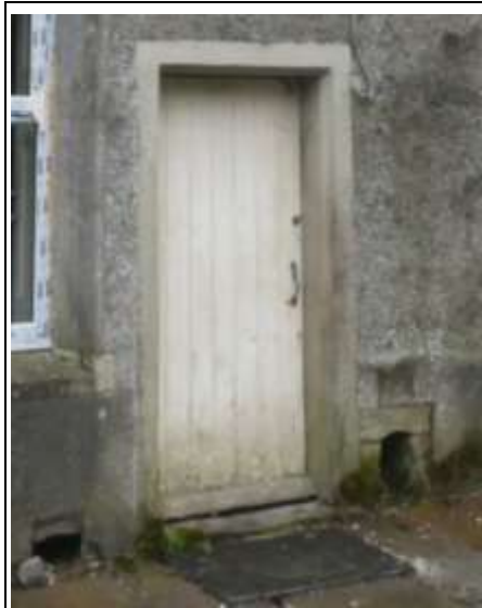
Stone Surround, Painted Timber Door
