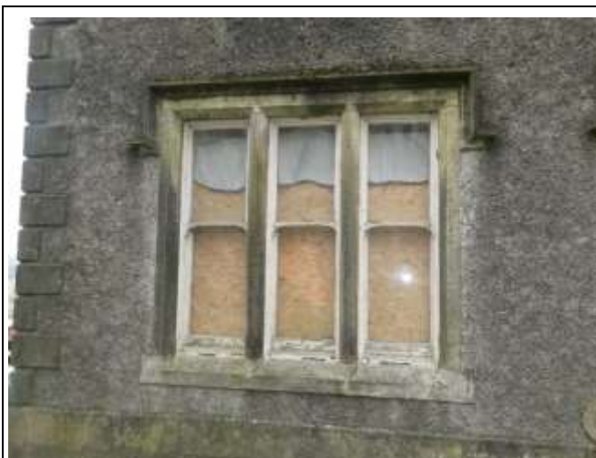
Triple Dressed Stone Window Surround, Ground Floor, to the North
