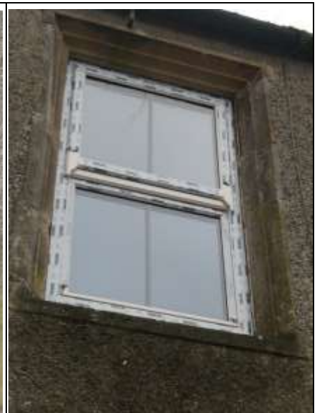
Window at the First Floor
