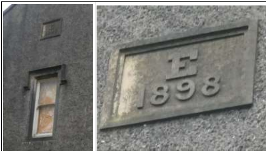
Stone Date Tablet Above Central Single Window
