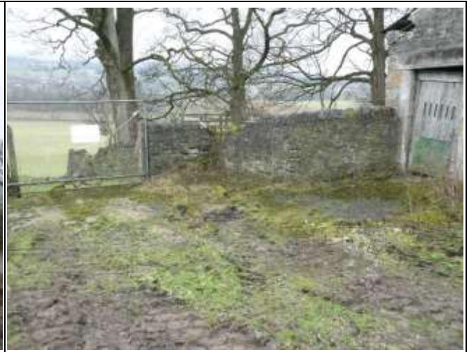
Stone Wall to the West of the Listed Barn, Approved New Access Point
