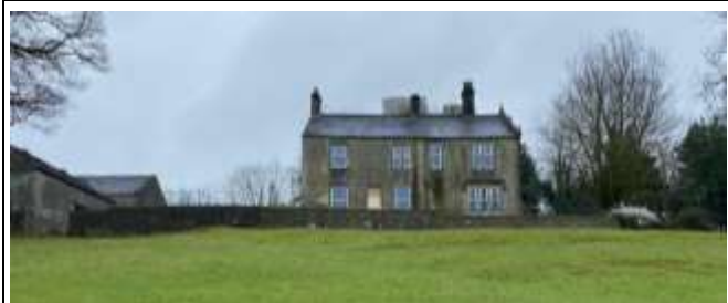
Looking South Towards the Farmhouse
