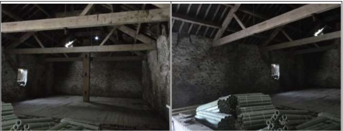
Timber Roof Structure in Main Section of the Barn
