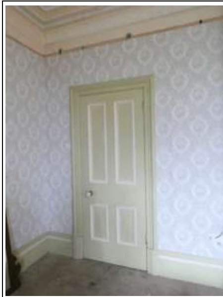
Painted Panelled Door Leading to Hall 1
