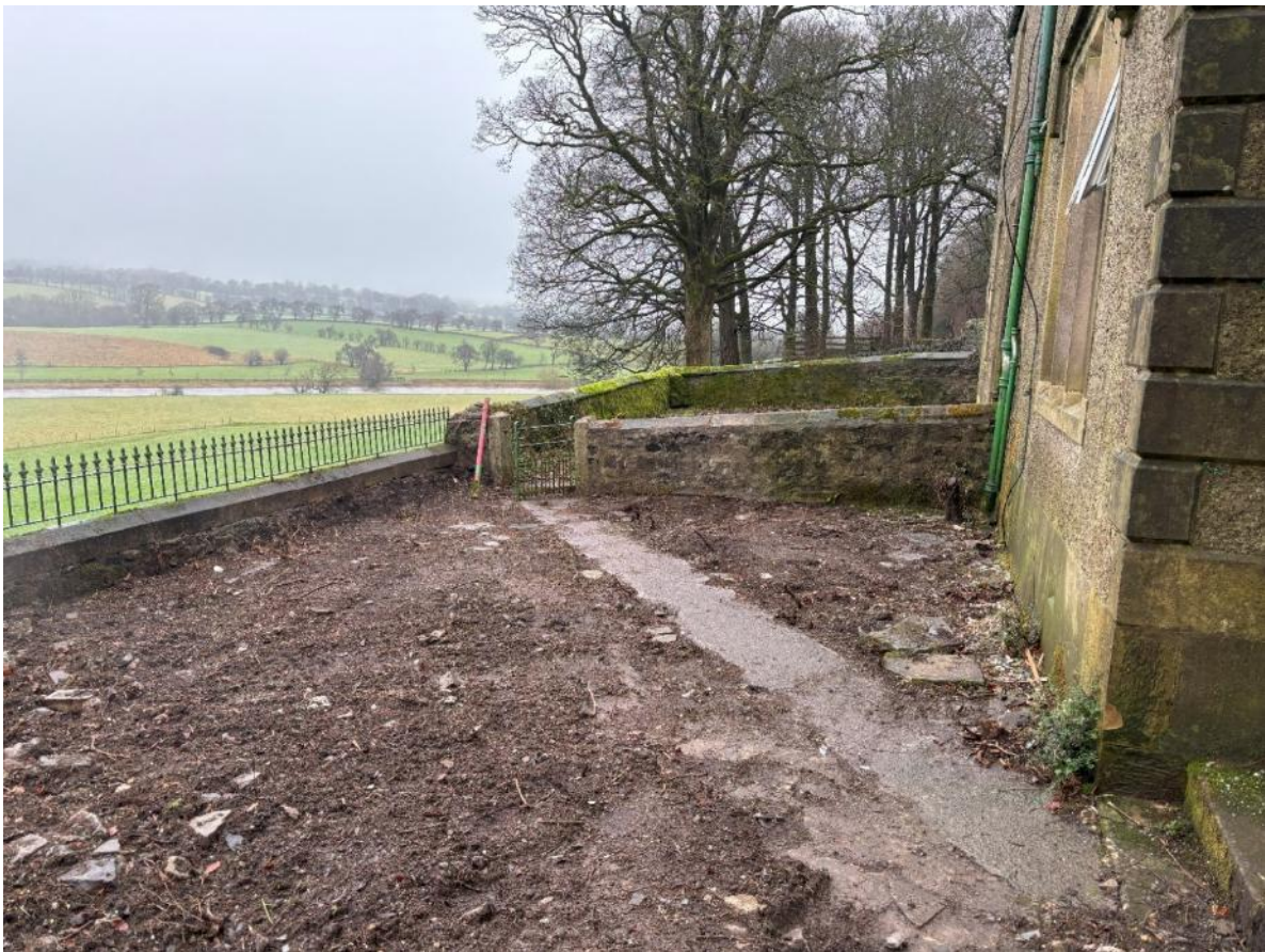
Figure 1. Unvegetated garden North West elevation of farm house
